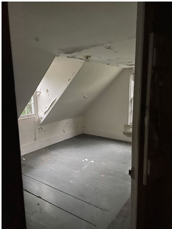
Figure 16: Second floor, northeast bedroom. Photograph taken June 9, 2022.
