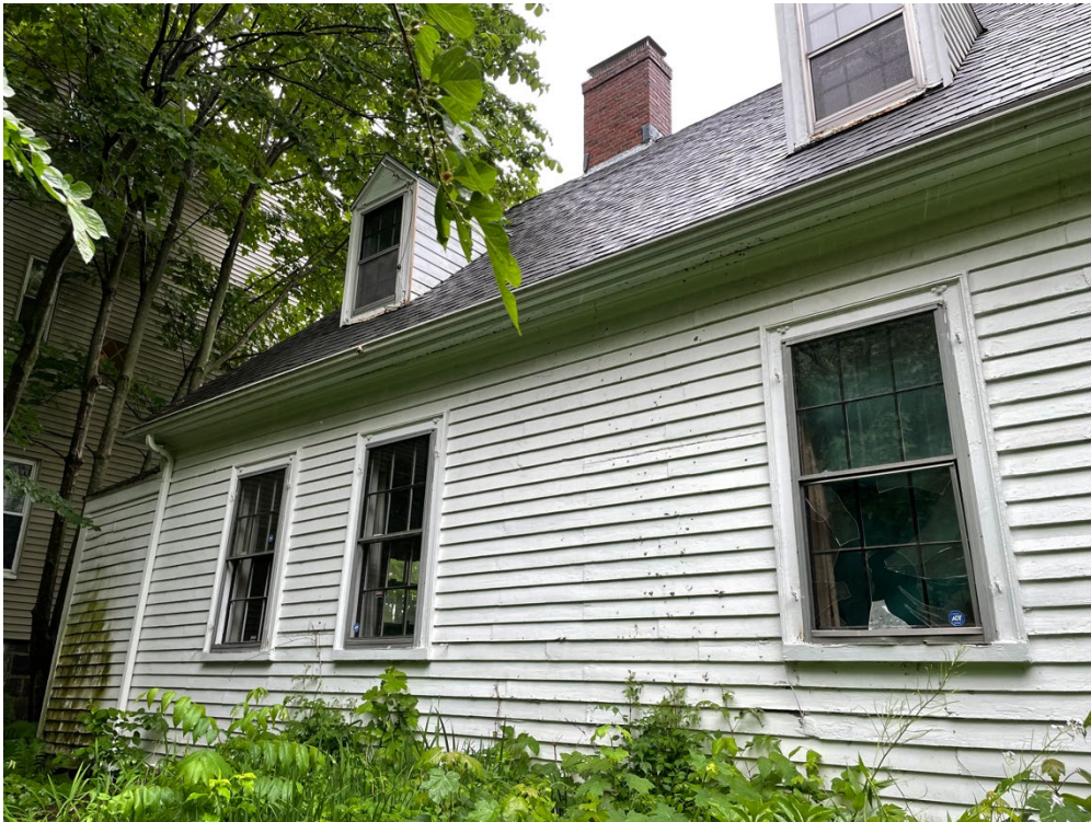
Figure 8: South facade (facing rear yard), looking northwest. Photograph taken June 9, 2022.
