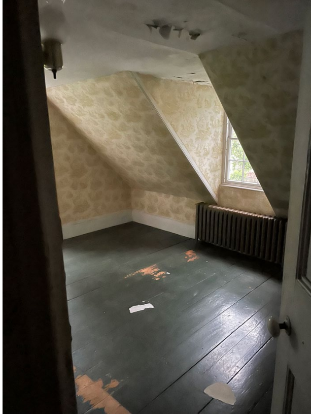
Figure 17: Second floor, southeast bedroom. Photograph taken June 9, 2022.
