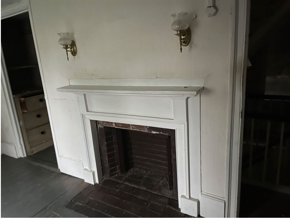
Figure 13: Fireplace in second floor northeast bedroom. Photograph by Joseph Cornish taken June 9, 2022
