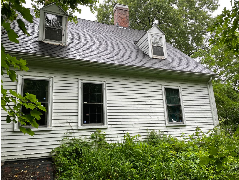
Figure 7: South facade (facing rear yard), looking northeast. Photograph taken June 9, 2022.
