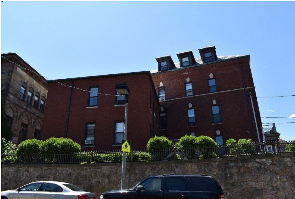
Figure 25. North elevation of the convent, facing south. Taken June 20, 2022.
