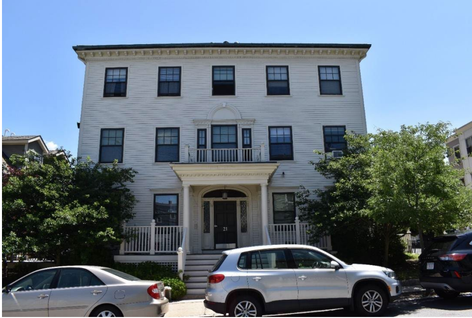
Figure 13. West (front) elevation of the rectory, facing east. Taken June 20, 2022.
