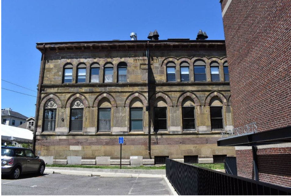
Figure 35. East elevation of the Cheverus School, facing west. Taken June 20, 2022.
