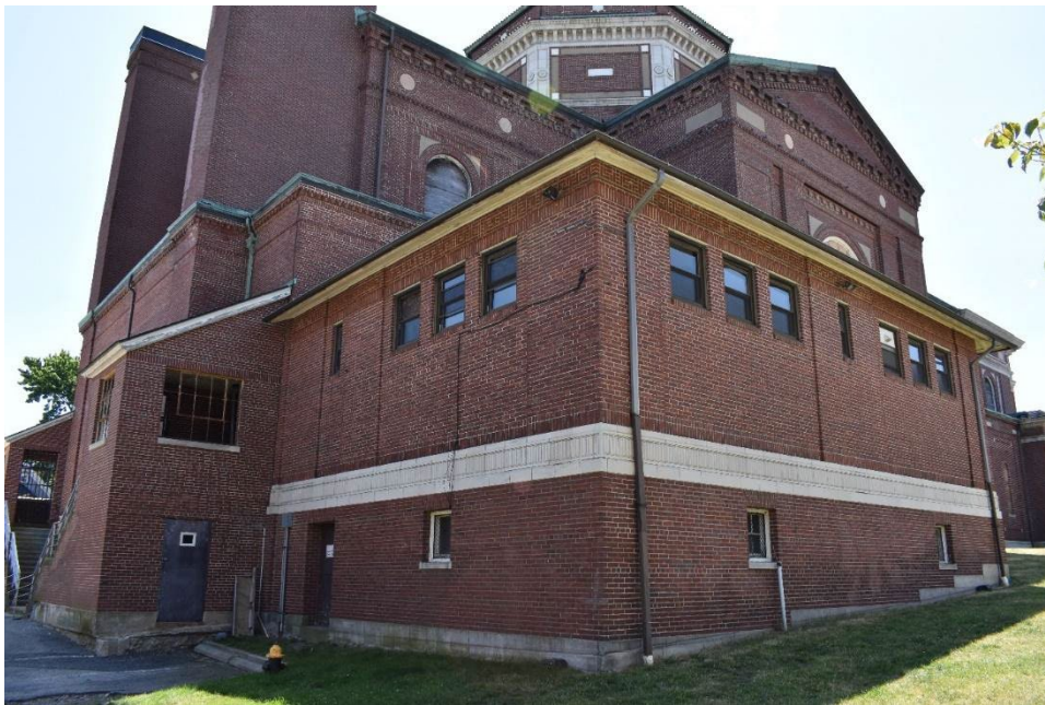
Figure 7. West elevation of the Church, facing southeast. Taken June 20, 2022.
