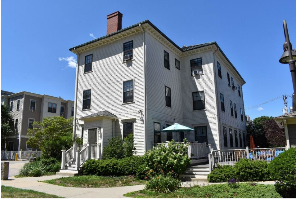
Figure 15. East (rear) elevation of the rectory, facing southwest. Taken June 20, 2022.
