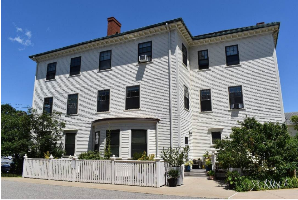
Figure 17. South elevation of the rectory, facing north. Taken June 20, 2022.
