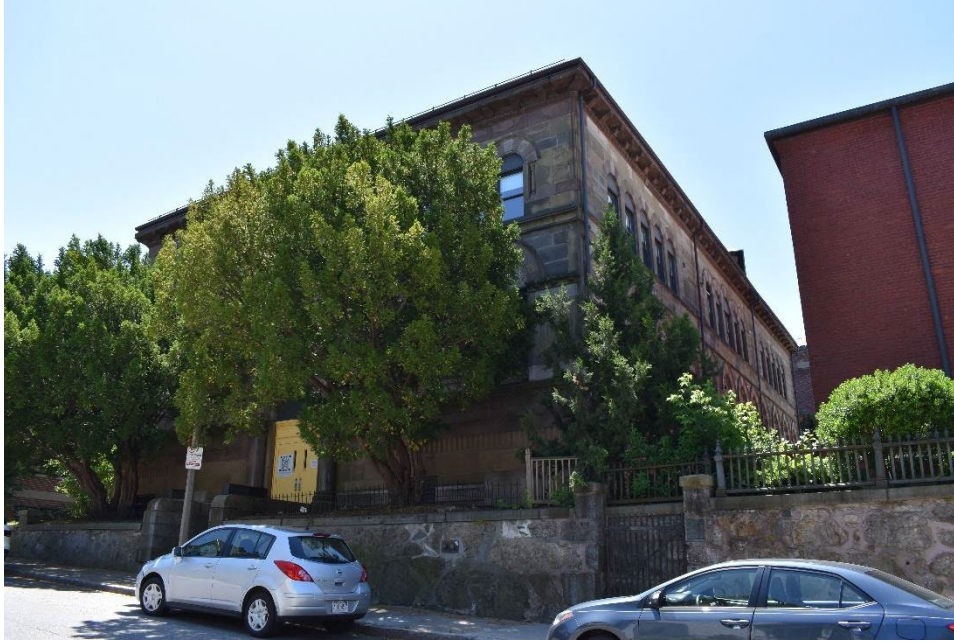
Figure 29. North (front) elevation of the Cheverus School, facing southeast. Taken June 20, 2022.
