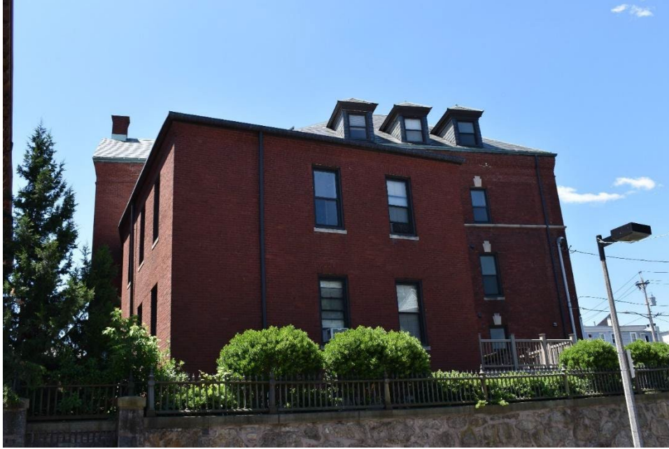
Figure 26. North elevation of the convent, facing south. Taken June 20, 2022.
