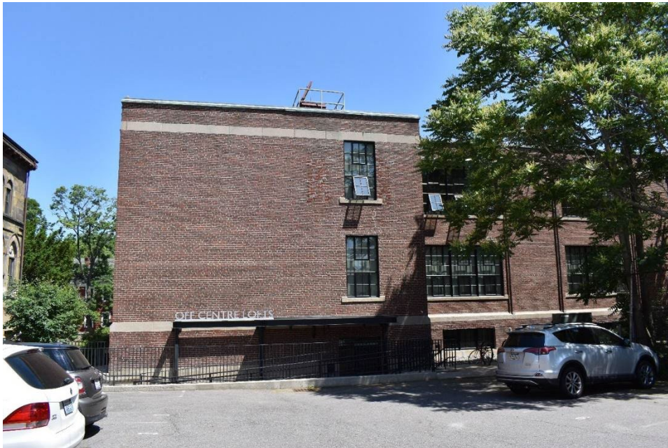
Figure 41. South (rear) elevation of St. Norbert School, facing north. Taken June 20, 2022.
