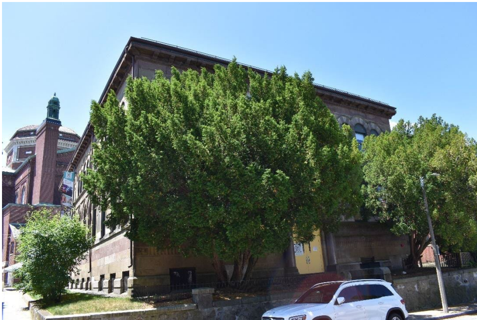
Figure 27. North (front) elevation of the Cheverus School, facing southwest. Taken June 20, 2022.
