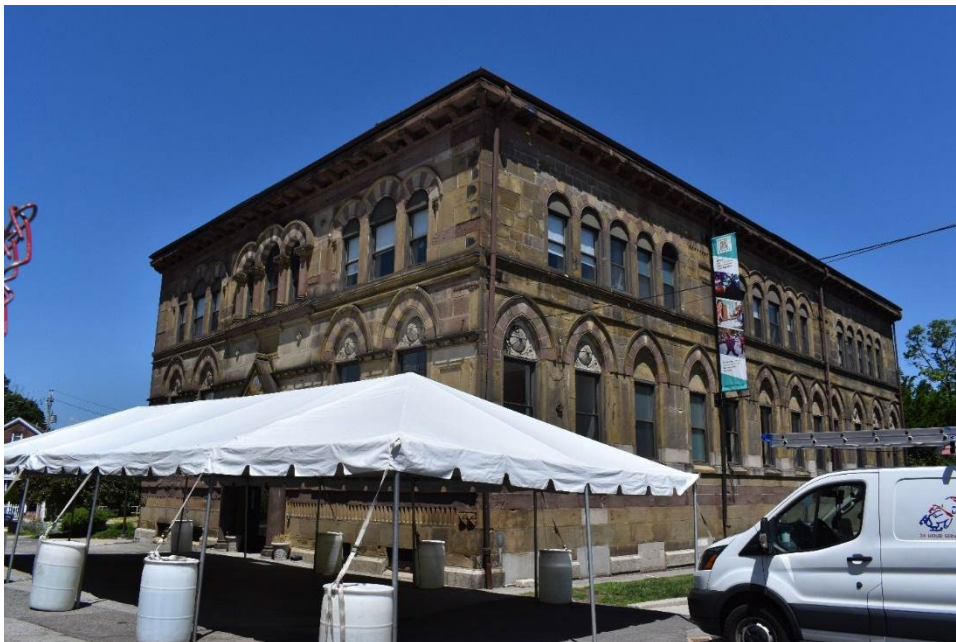
Figure 34. East elevation of the Cheverus School, facing northwest. Taken June 20, 2022.
