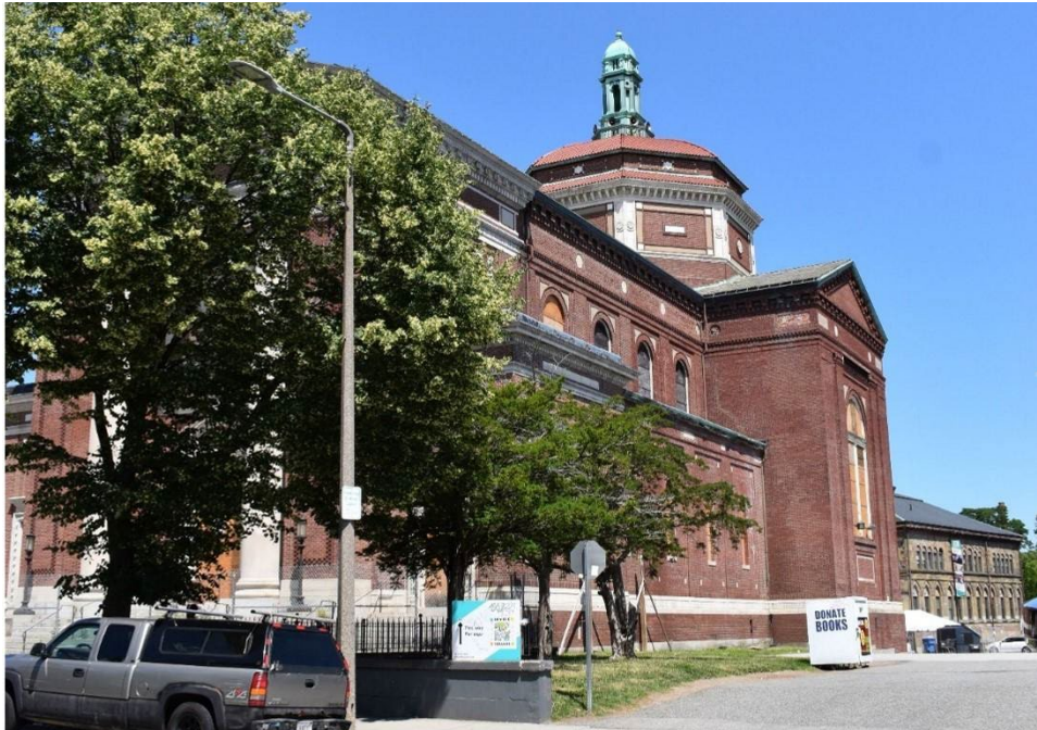
Figure 11. East elevation of the Church, facing northwest. Taken June 20, 2022.
