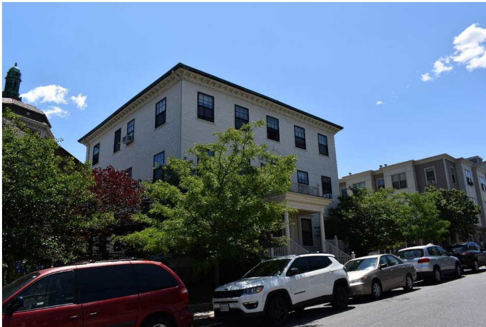
Figure 14. North elevation of the rectory, facing southeast. Taken June 20, 2022.
