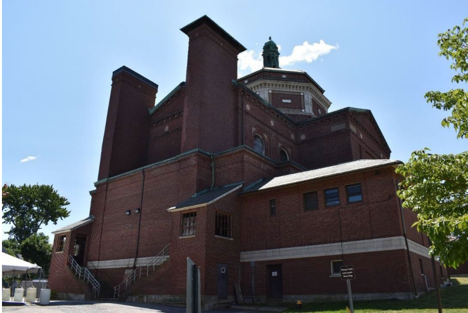
Figure 8. North (rear) elevation of the Church, facing southeast. Taken June 20, 2022.
