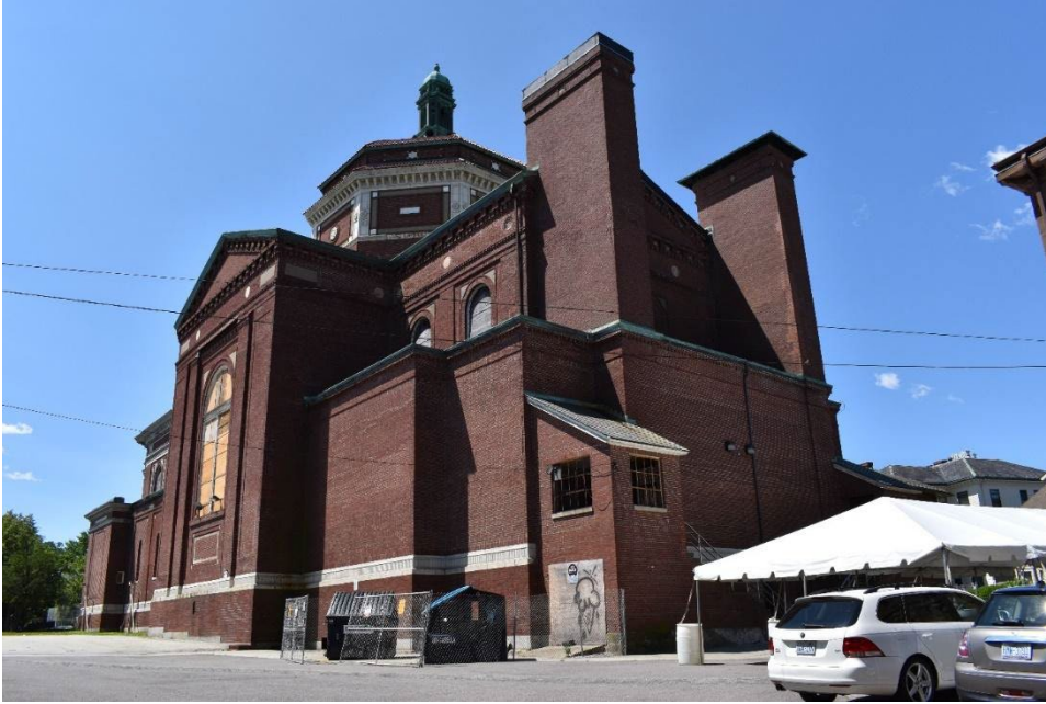
Figure 10. East elevation of the Church, facing southwest. Taken June 20, 2022.
