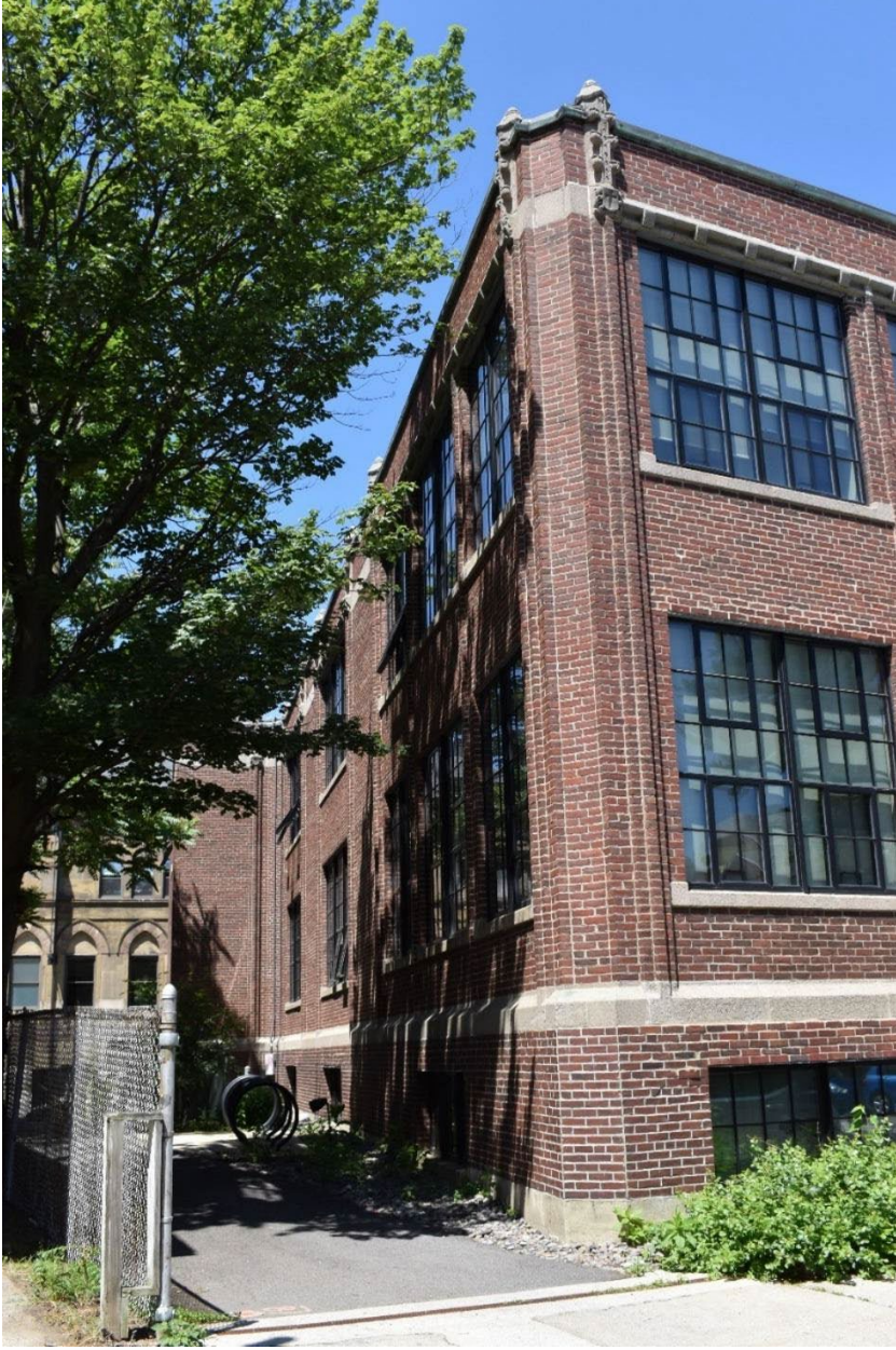
Figure 39. South (rear) elevation of St. Norbert School facing northwest. Taken June 20, 2022.
