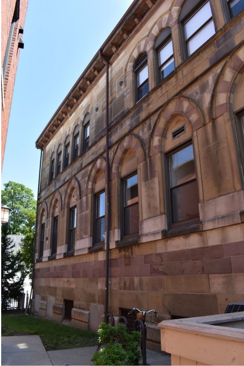
Figure 30. West elevation of the Cheverus School facing northeast. Taken June 20, 2022.
