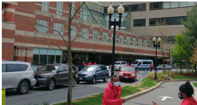
Existing Menino Entrance Canopy
