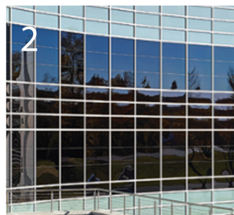
2 Glazed Extruded Alum. Curtain Wall System
