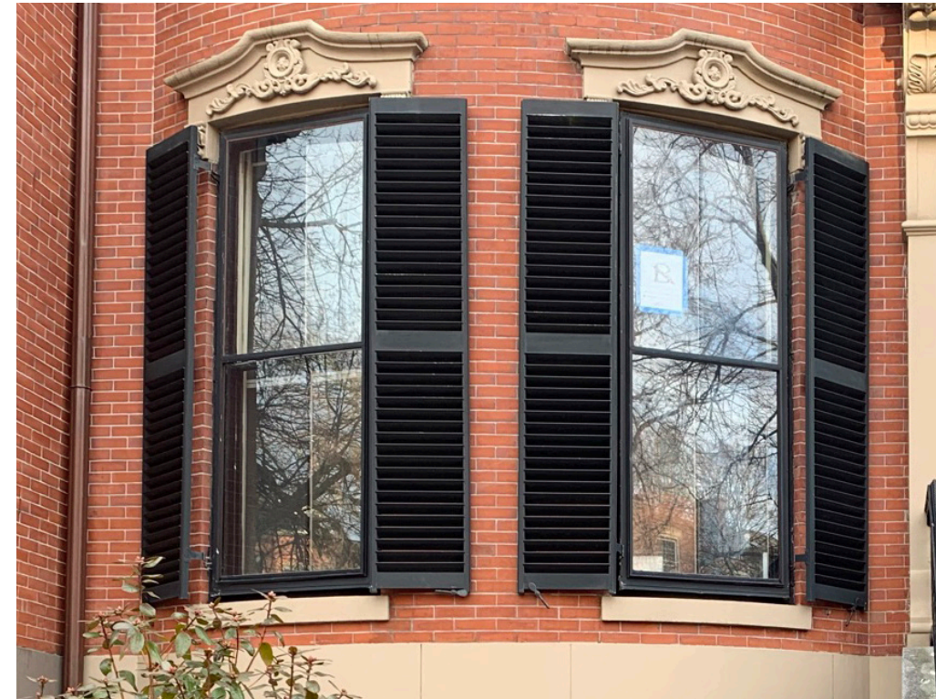
PARLOR WINDOWS WITH EXTERIOR STORMS
