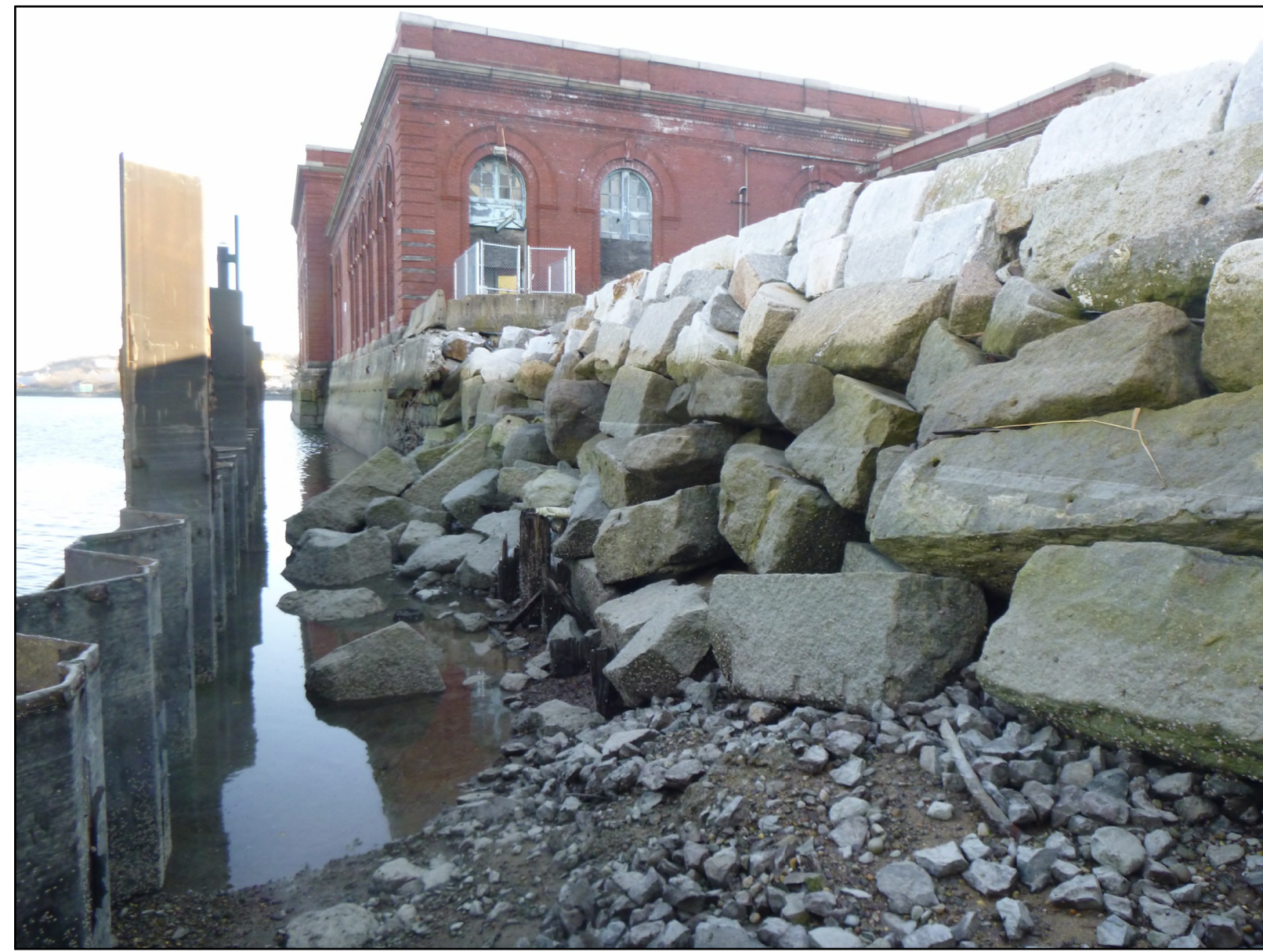
PHOTO 6: BRIDGE ABUTMENT SHORELINE
