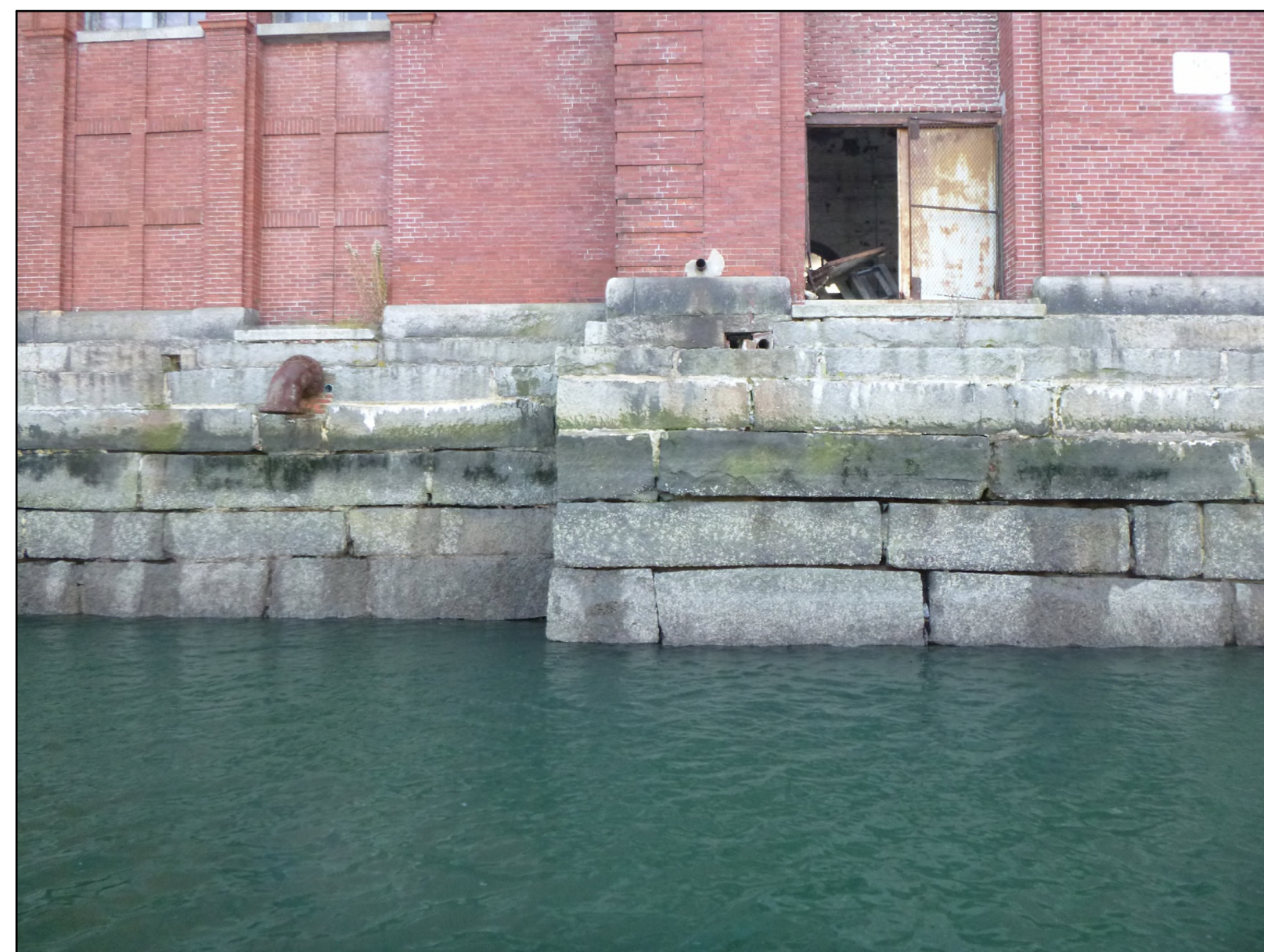
PHOTO 9: BLOCK SEAWALL CORNERS
