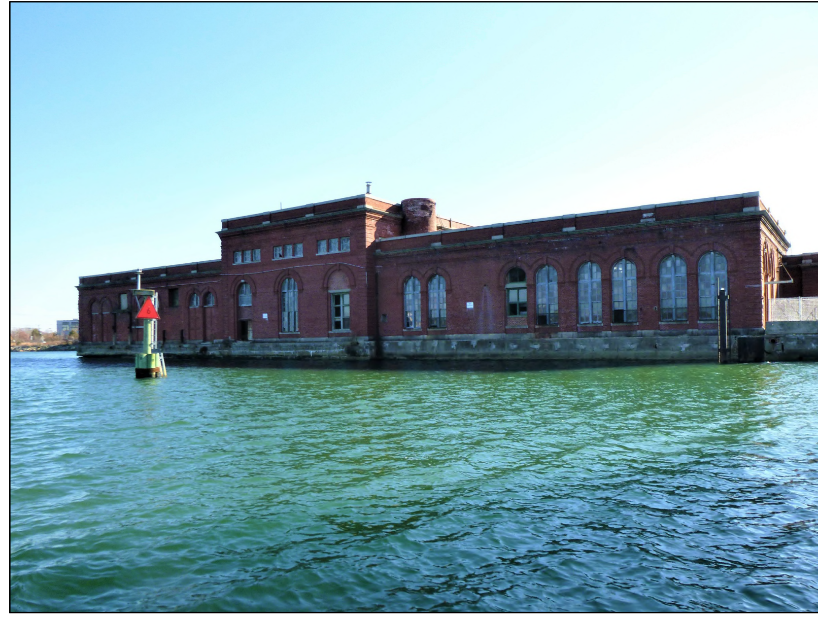
PHOTO 2: OUTSHORE VIEW OF THE NORTH SIDE OF THE BUILDING
