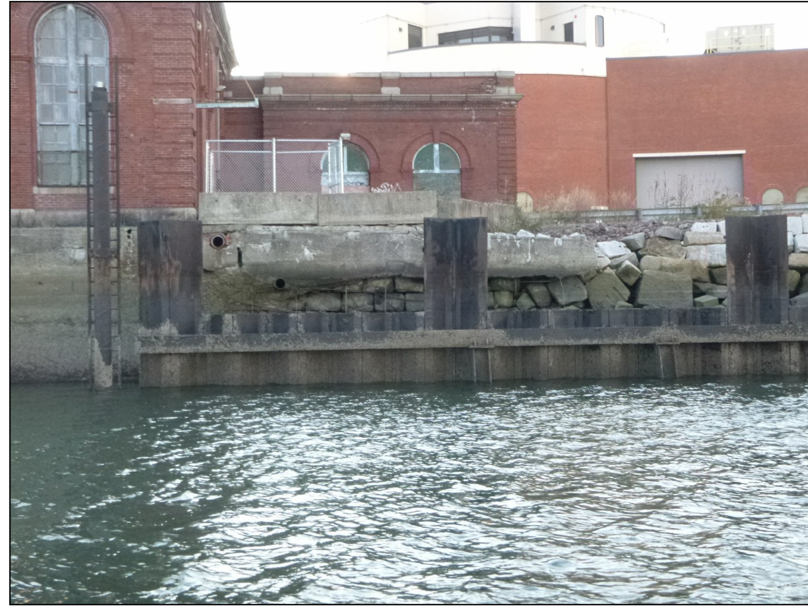
PHOTO 4: WEST SIDE OF BUILDING NEAR BRIDGE NAVIGATIONAL AID
