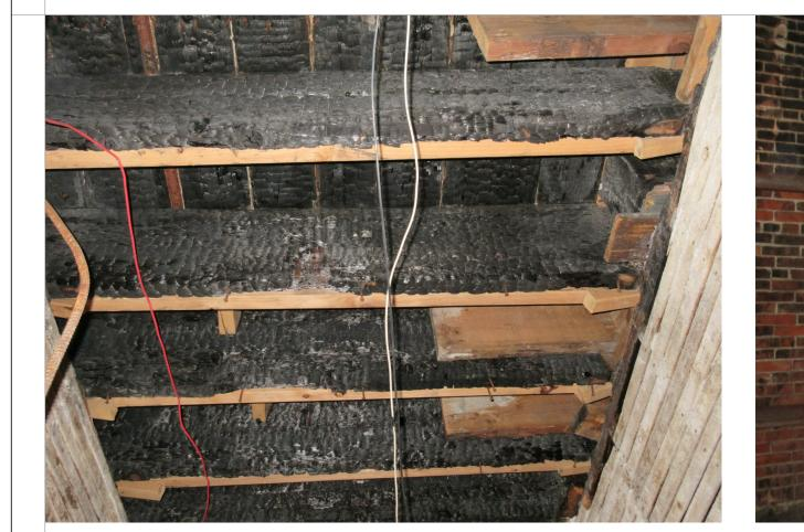
FIRE DAMAGE AT FLOOR FRAMING
