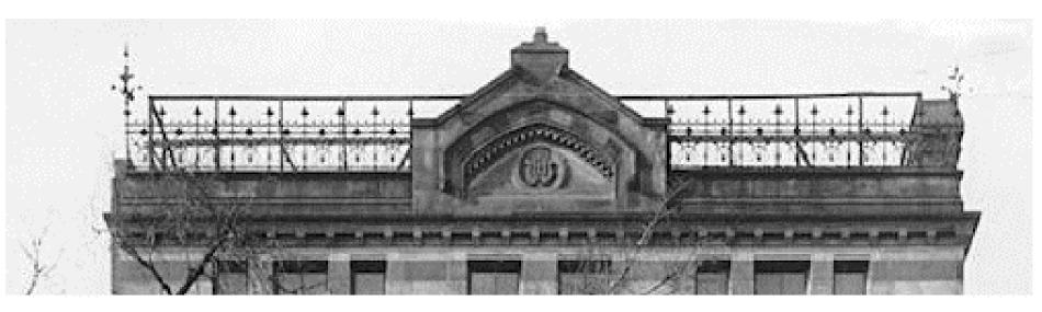
PHOTO 6: ORIGINAL CAST IRON ROOF CRESTING TO BE REPLICATED
