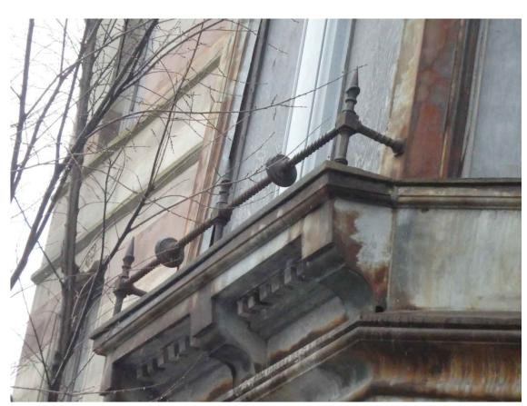
PHOTO 4: EAST ELEVATION, REPLICATE EXISTING HISTORIC CAST IRON RAIL ON BALCONY ON BAY WHERE MISSING
