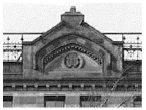
PHOTO 7: ORIGINAL SANDSTONE GABLE DETAIL TO BE REPLICATED WHERE DETAILS ARE NOW MISSING
