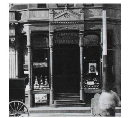
PHOTO 5: 1899 PHOTO SHOWING STORE FRONT WITH CAST IRON STAIRS WITH PRISM LIGHTS AND DOUBLE DOORS
