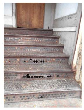
PHOTO 1: EXISTING BALCONY CAST IRON RAIL ON THE SOUTH ELEVATION. PHOTO 2: EAST ELEVATION. RESTORE REPLICATE EXISTING BALCONY RAIL WHERE MISSING ON SOUTH AND EAST CAST IRON STAIRS WITH PRISM LIGHTS ELEVATIONS.
