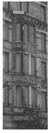
PHOTO 3: EAST ELEVATION, ORIGINAL SHEET METAL BAYS TO BE REPLICATED
