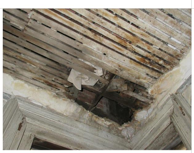
WATER DAMAGE AT CEILING
