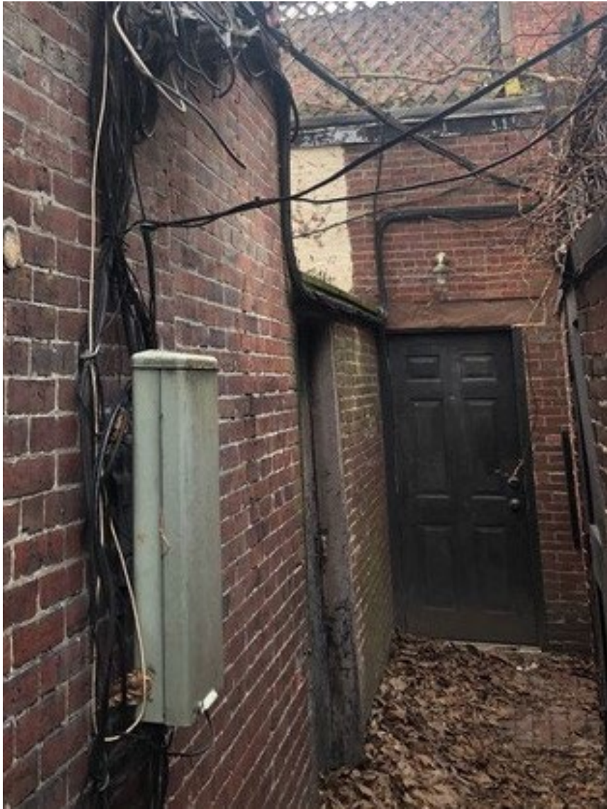
Public Alley egress door that was replaced
