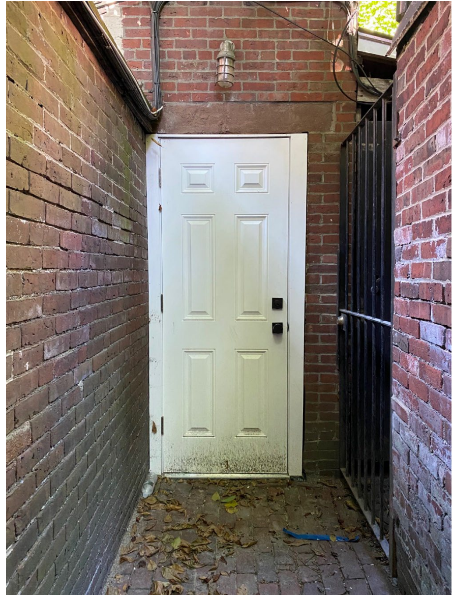
Newly installed egress door
