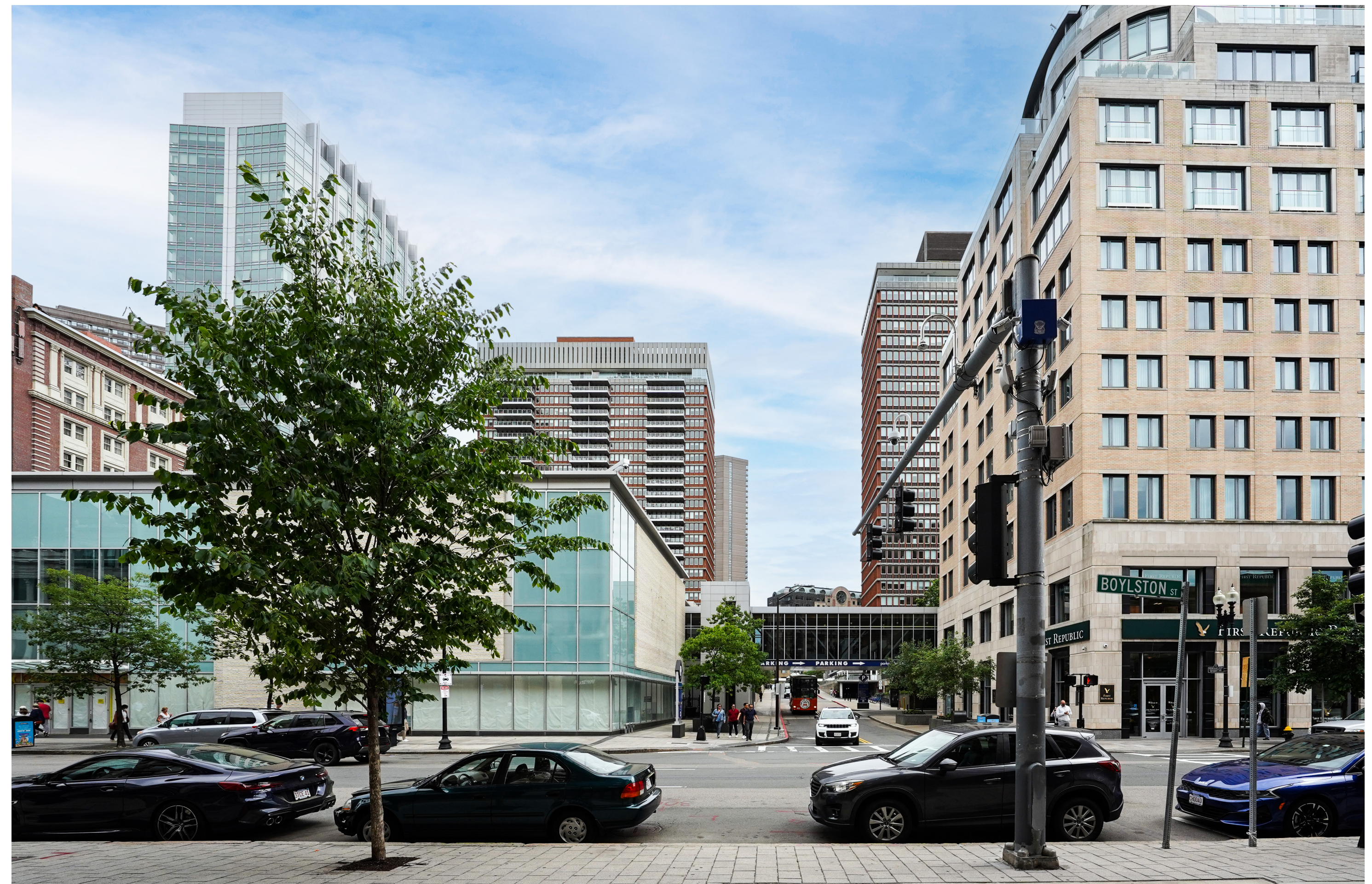
View Across the Street from Max Brenner Store Location
