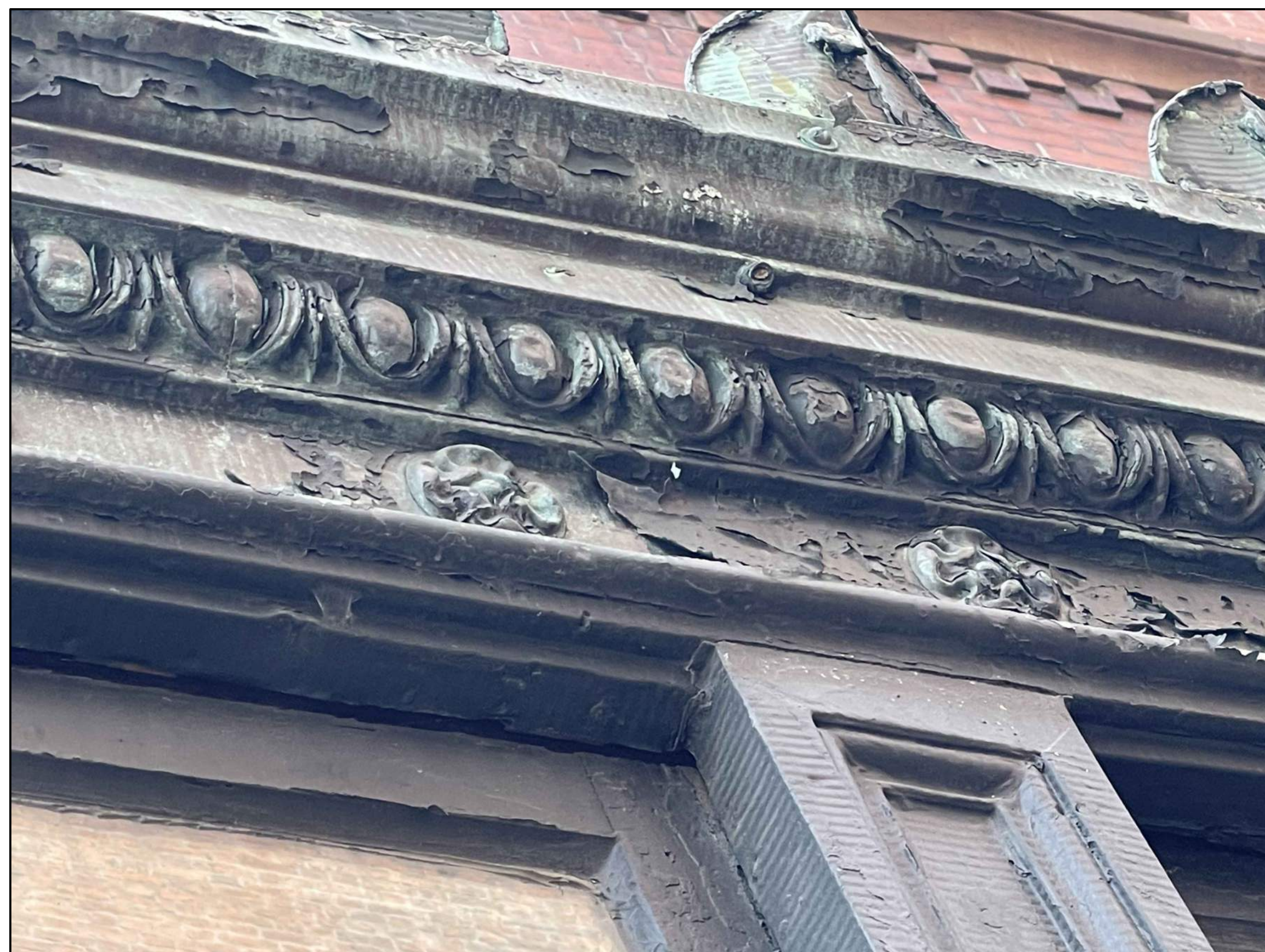
COPPER WALL CLADDING
