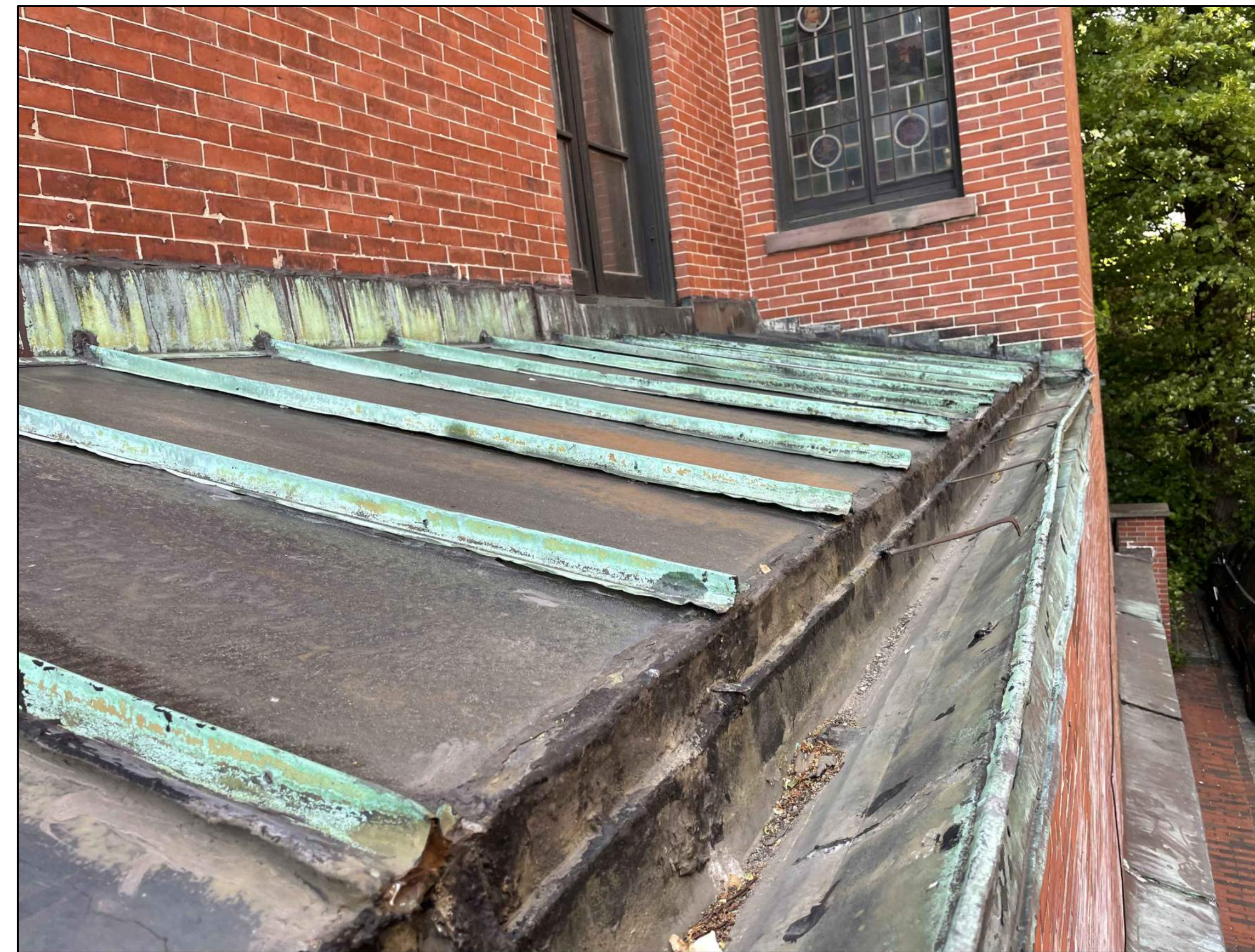
SOLARIUM AS VIEWED FROM ABOVE
