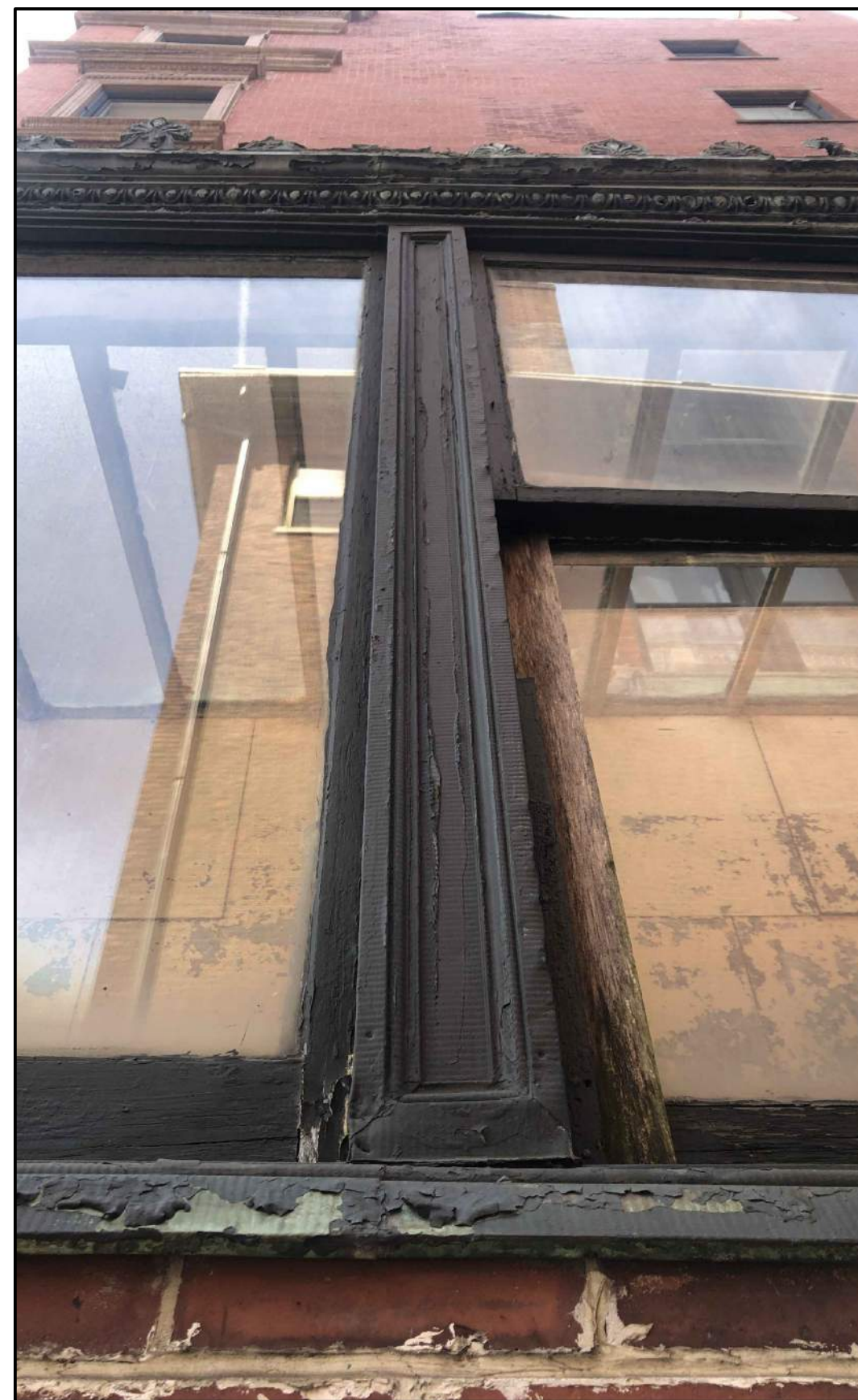
ROTTED WOOD AND DETERIORATED COPPER WALL CLADDING, TYPICAL
