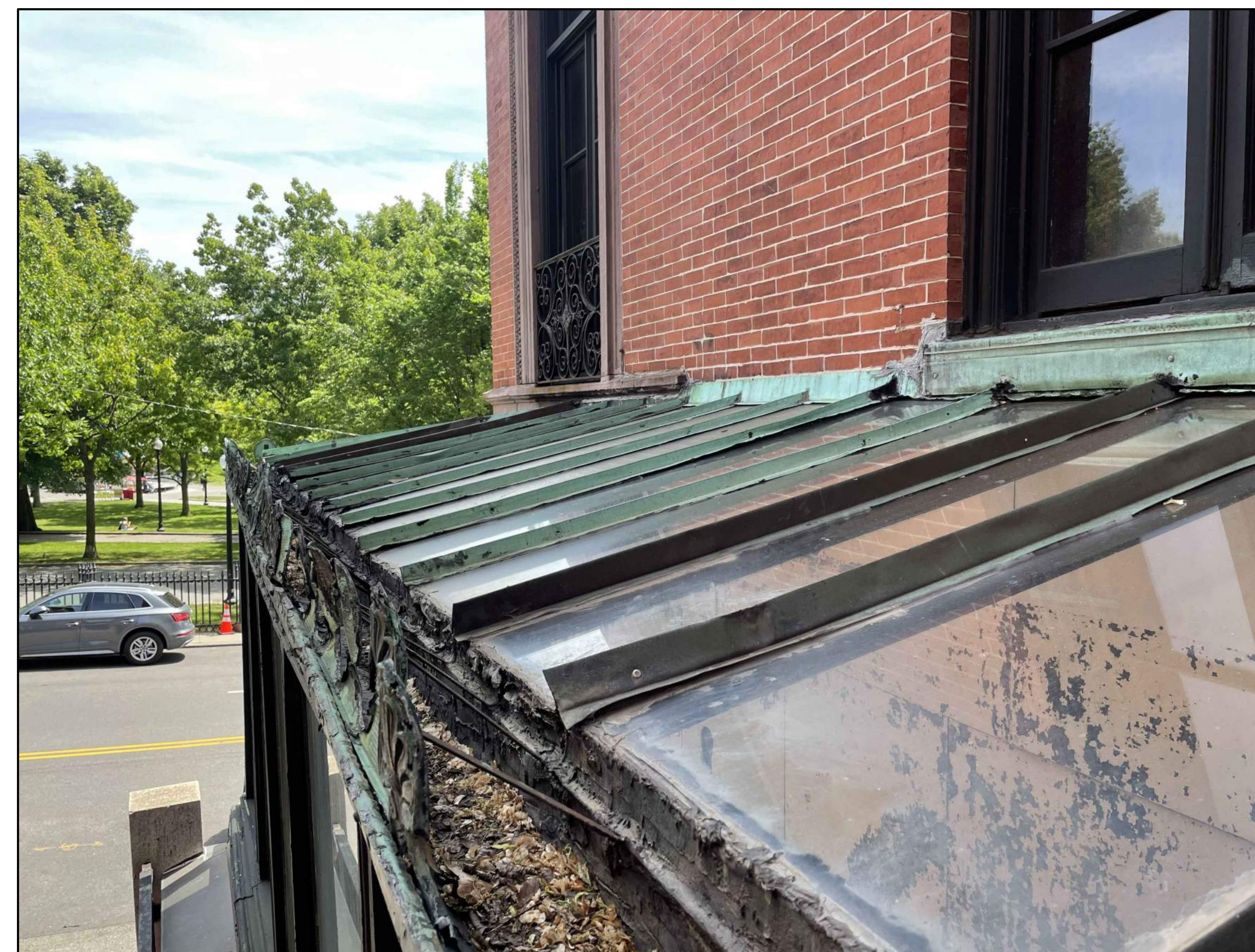
SOLARIUM AS VIEWED FROM ABOVE
