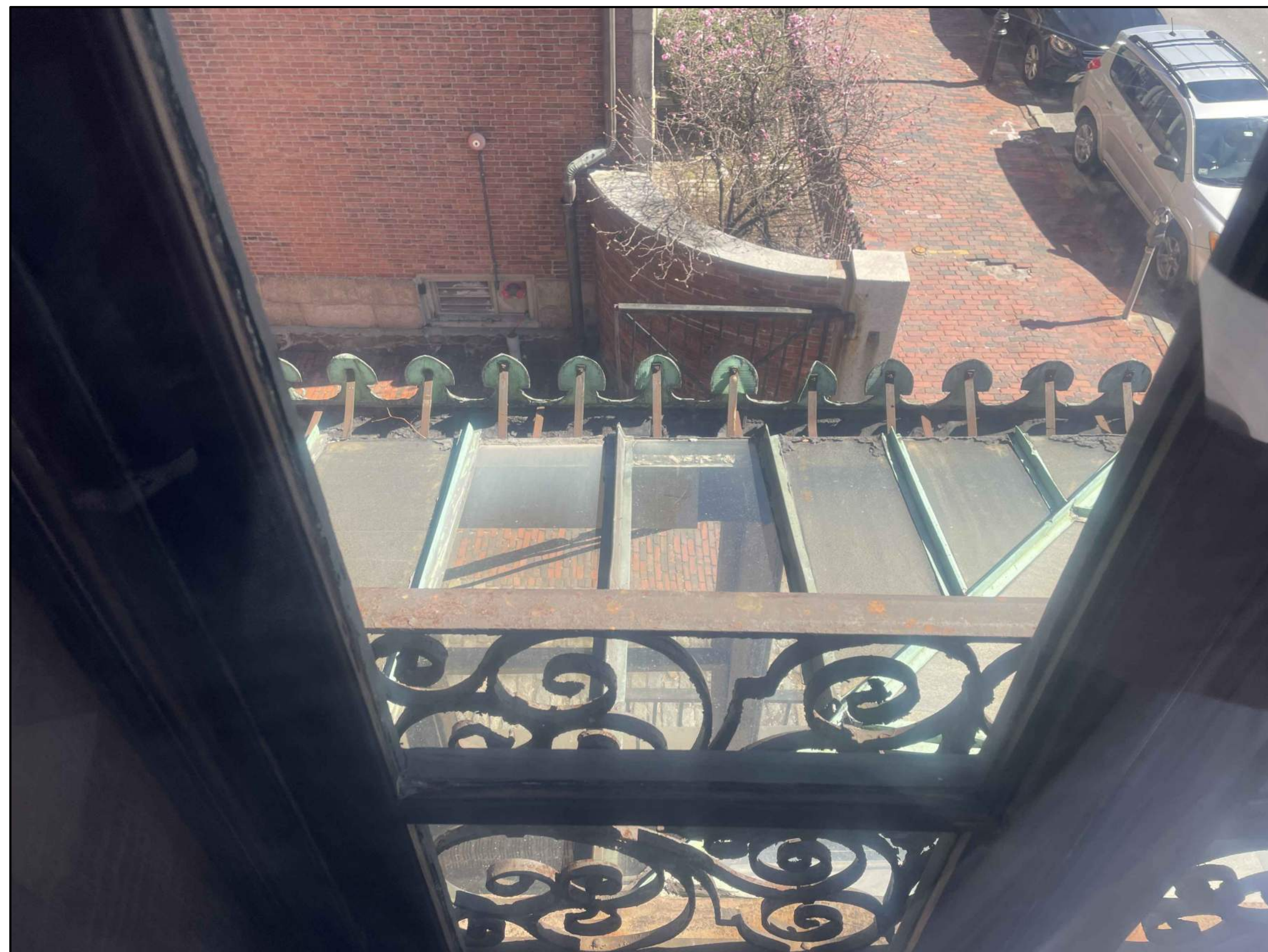
SOLARIUM ROOF AS VIEWED FROM THE INTERIOR
