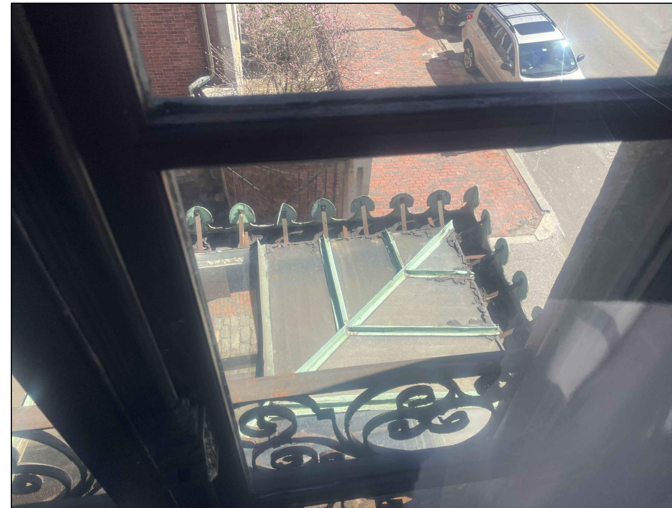
SOLARIUM ROOF AS VIEWED FROM THE INTERIOR
