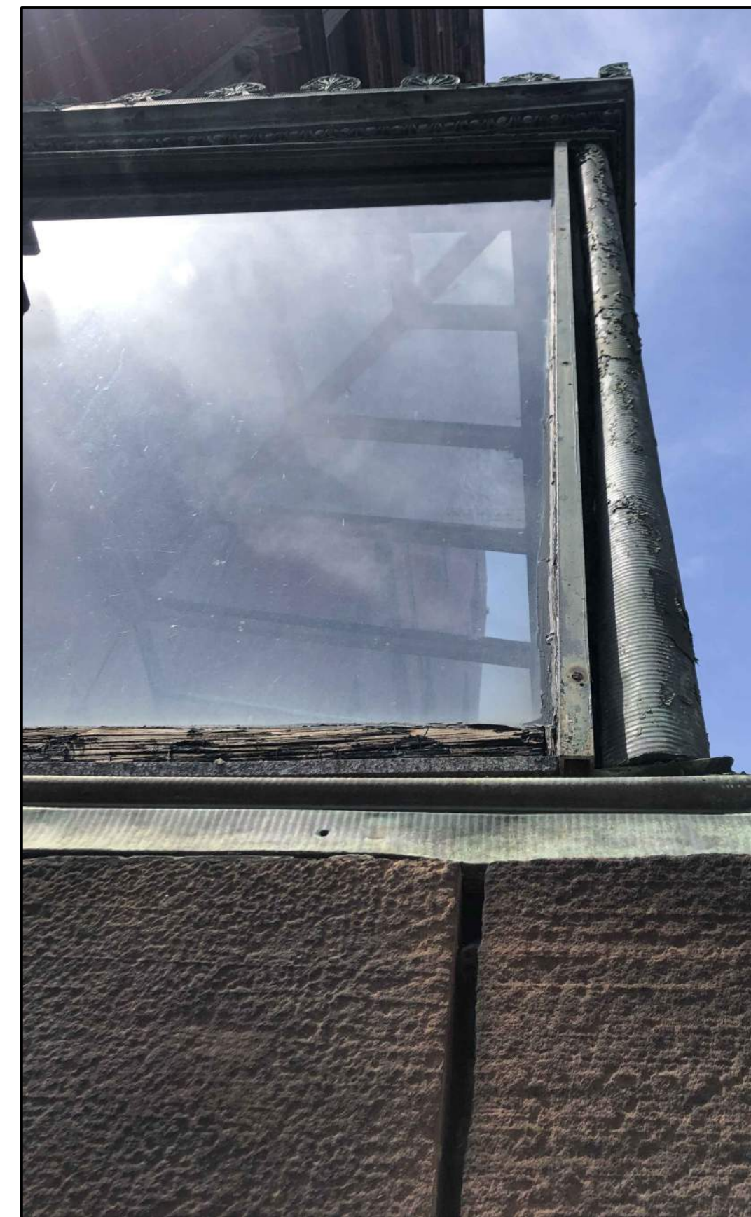
ROTTED WOOD AND DETERIORATED COPPER WALL CLADDING, TYPICAL
