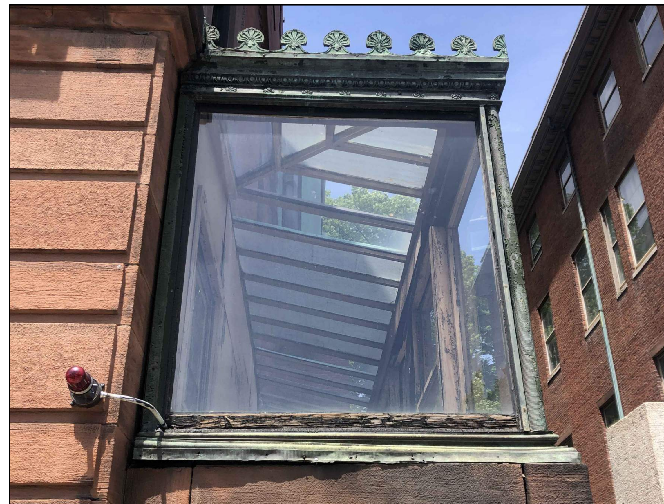
SOLARIUM AS VIEWED FROM BEACON STREET
