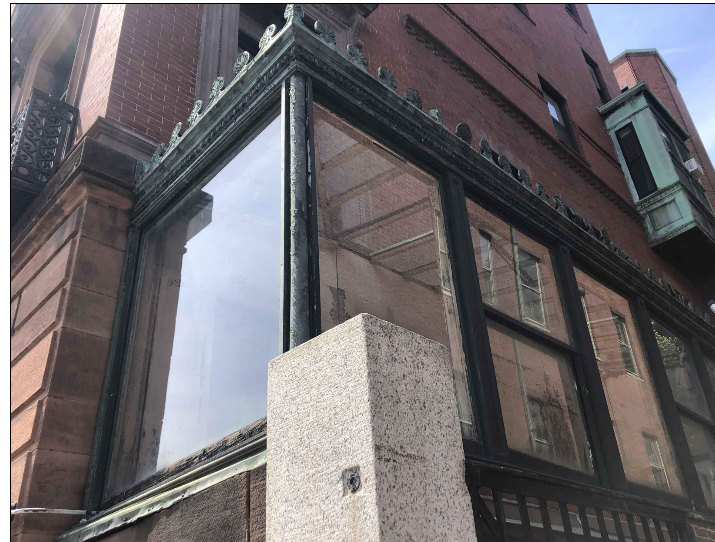
SOLARIUM AS VIEWED FROM BEACON STREET
