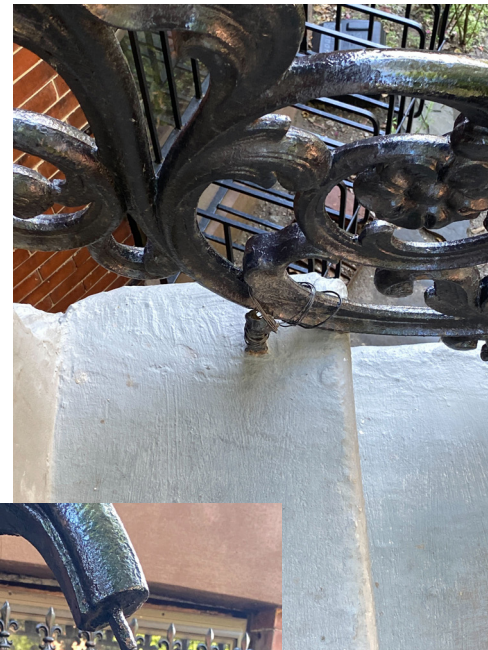
Damage on existing front railings
