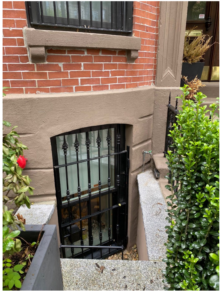
Existing window well at 8 Rutland Square
