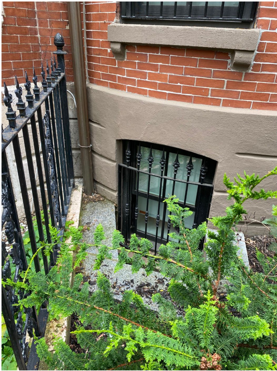
Existing window well at 8 Rutland Square
