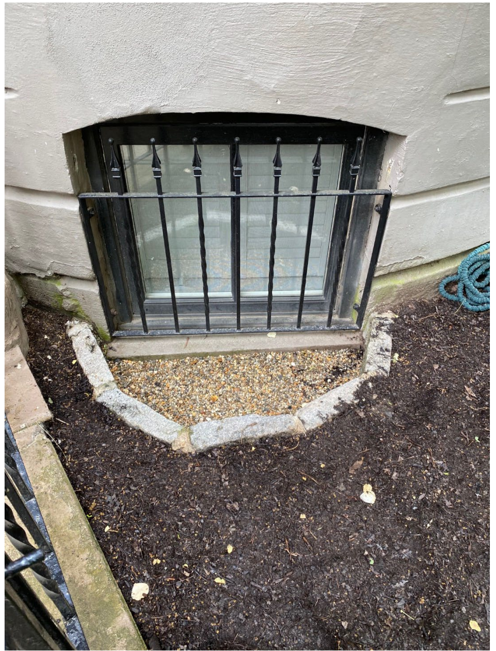
Existing window well
