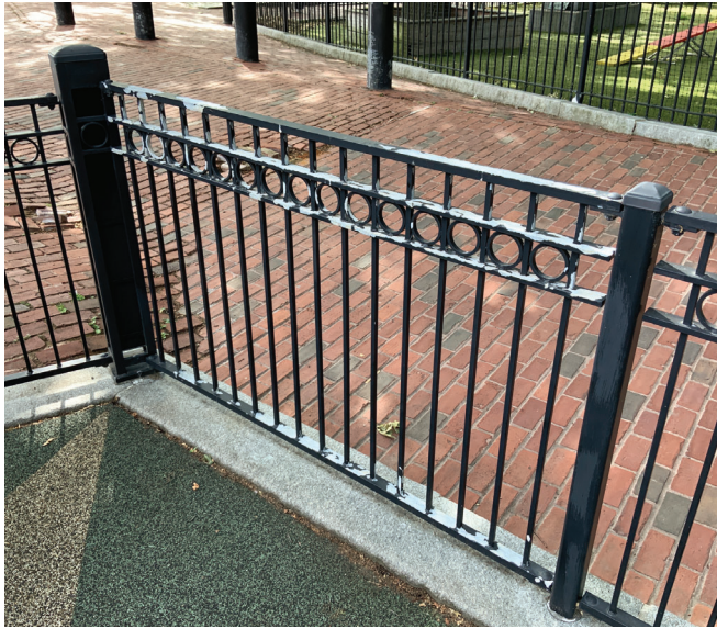
Existing fence to remain and be touched-up.
