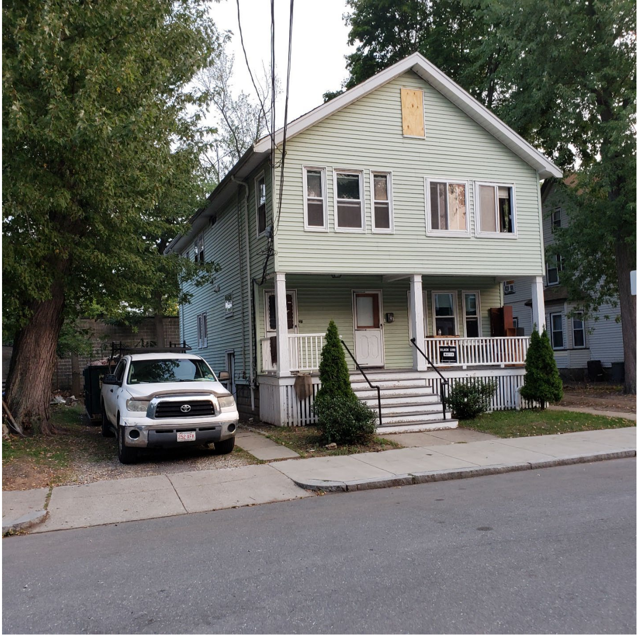
1. Front view of 103-105 Hooker Street
