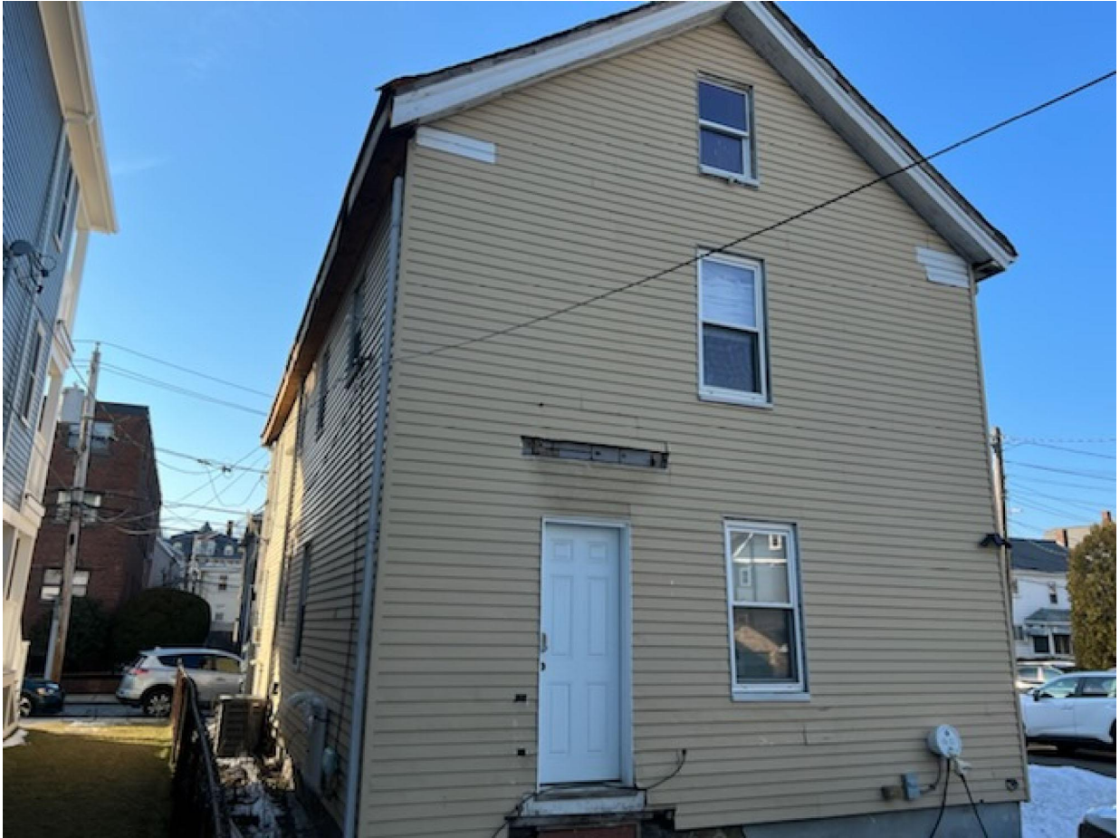
36 Shepard Street - Rear View
