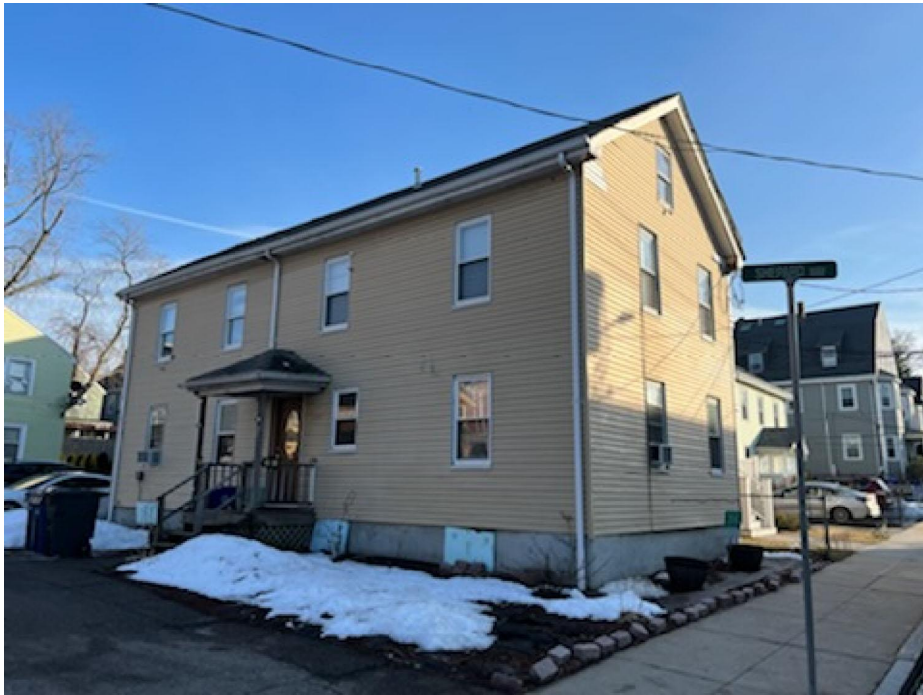
36 Shepard Street - Left Side View - Building Entrance
