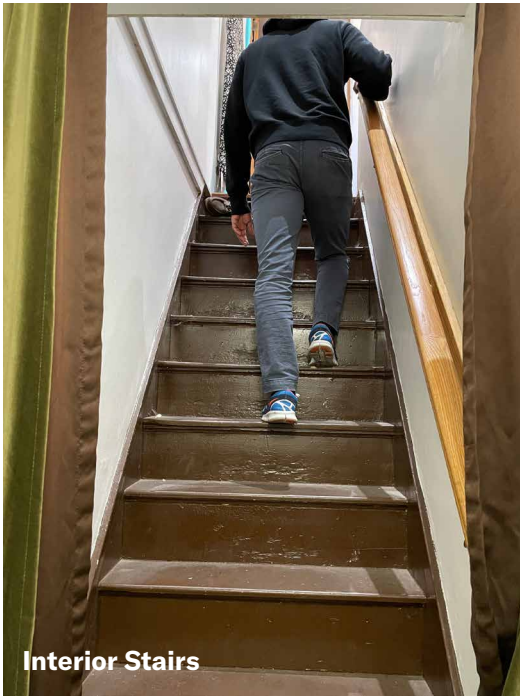
Risers and treads are not to current building code
