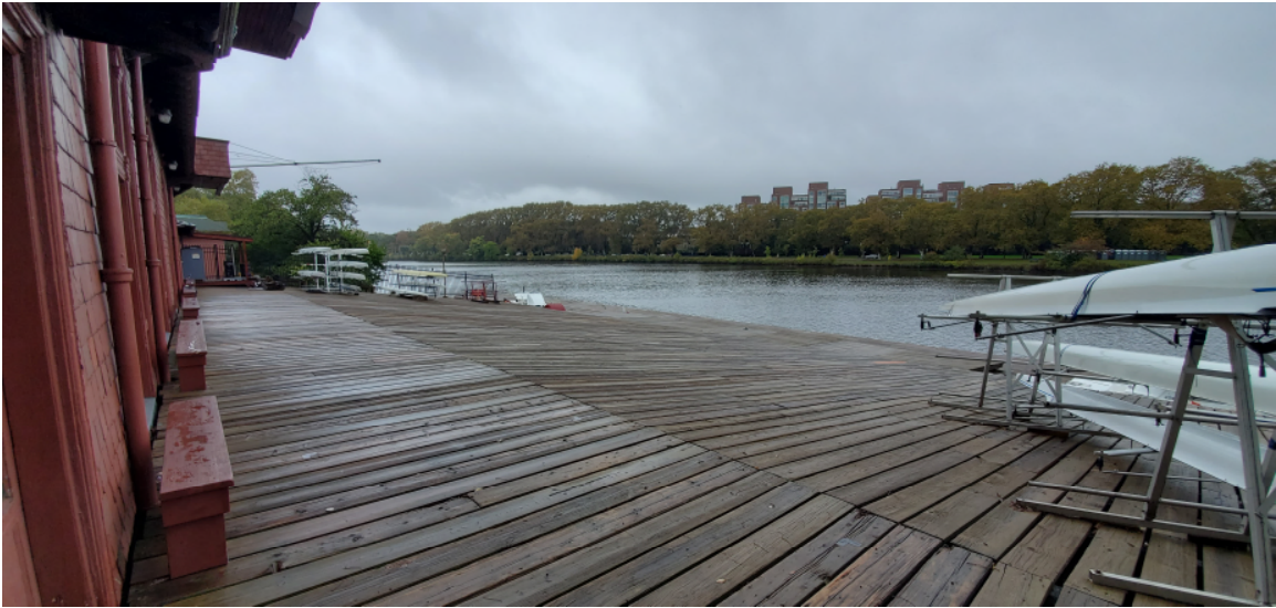
Photo 5 – Looking northwest from the top of the dock
