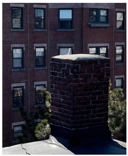
Remove derelict chimney, which is structurally unsound, and logistically difficult to restore
