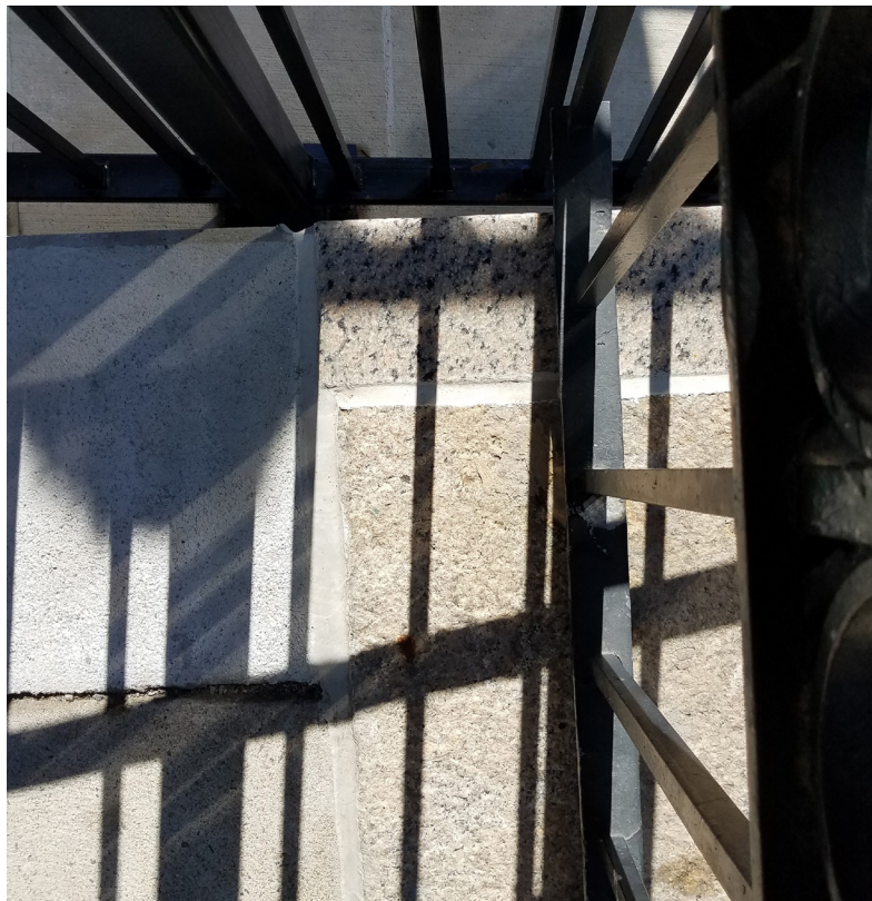
V: GRANITE TO CONCRETE TRANSITION BY RAMP AND MCKINLEY TERRACE
