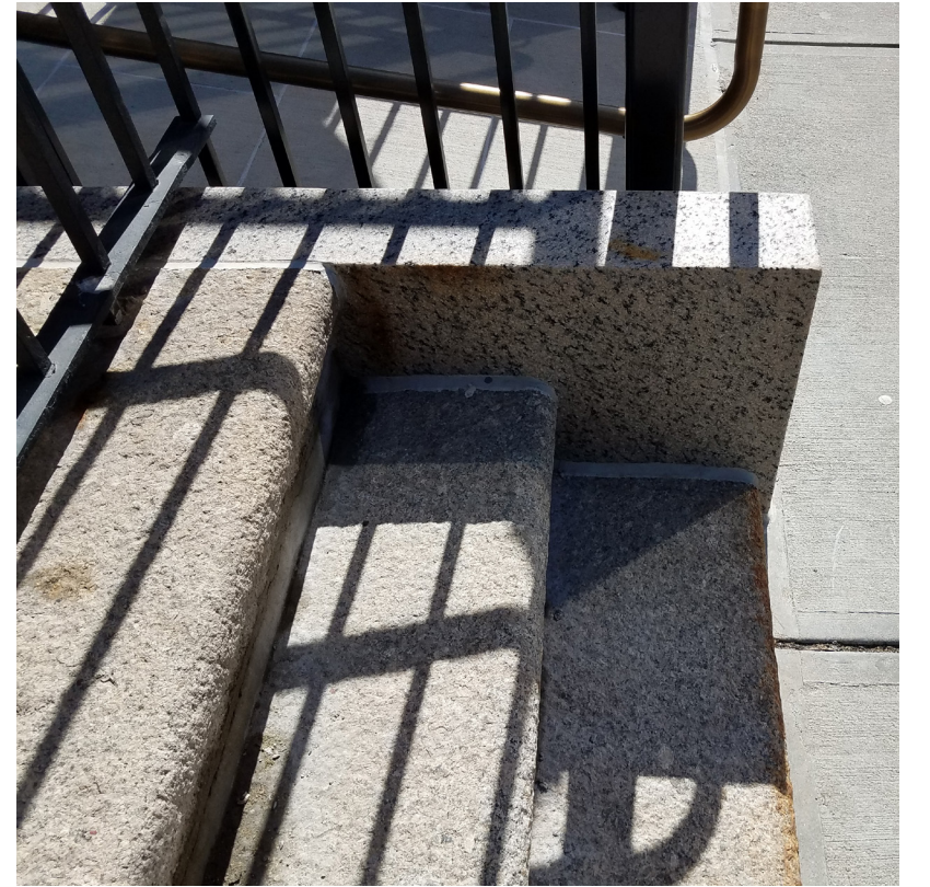
T: GRANITE CHEEK WALL AT TERRACE STEPS
