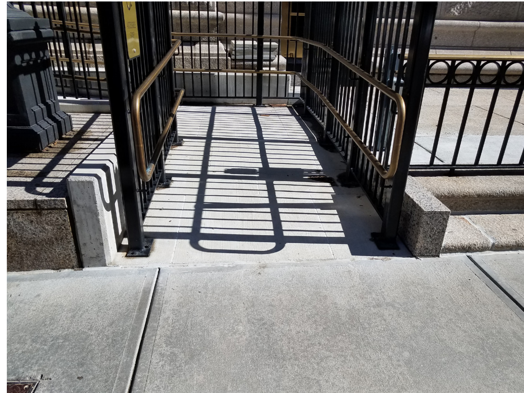
B: RAMP VIEW FROM SIDEWALK
