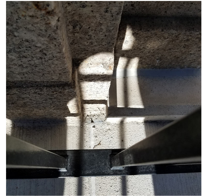
N: CONCRETE SHELF AT FACADE
