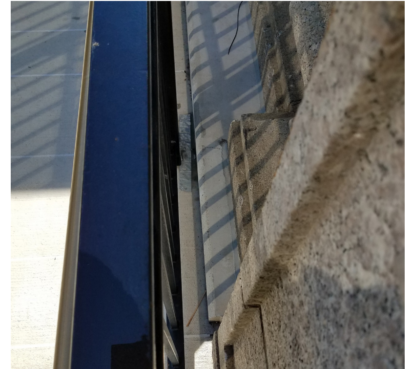
Z: CONCRETE SHELF BY FACADE
