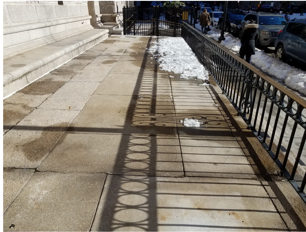
EE: TERRACE - STONE PAVERS AND POURED CONCRETE
