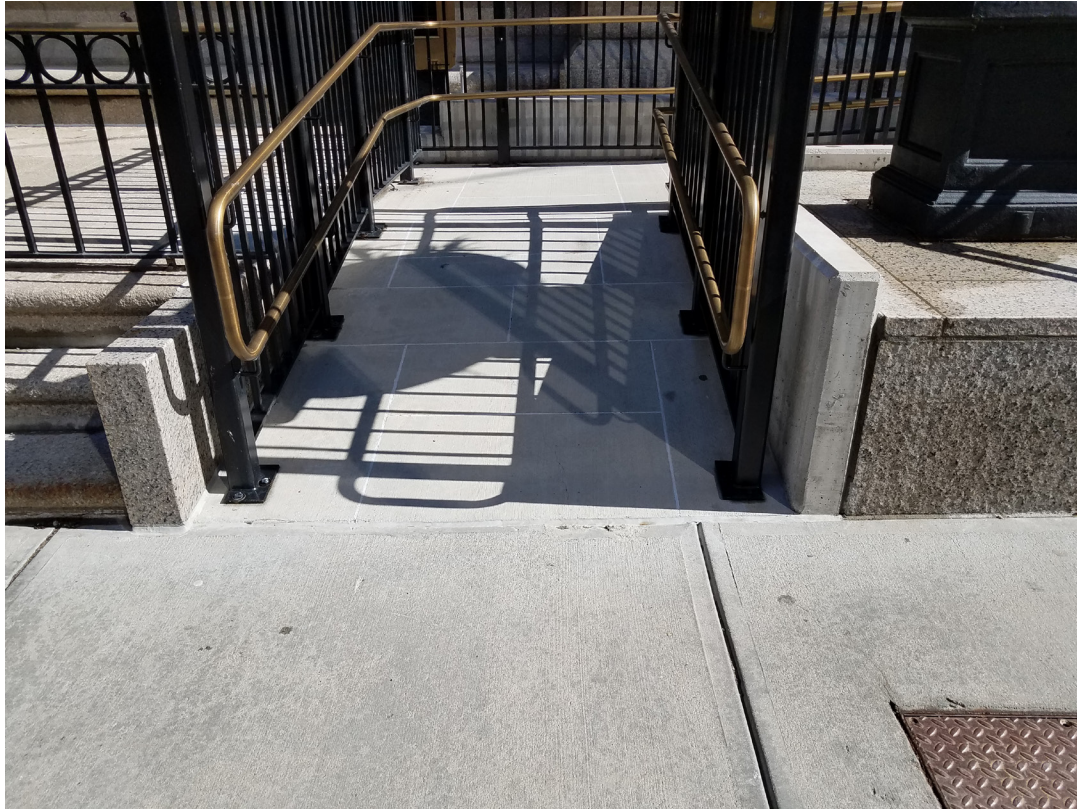
R: RAMP FROM SIDEWALK
