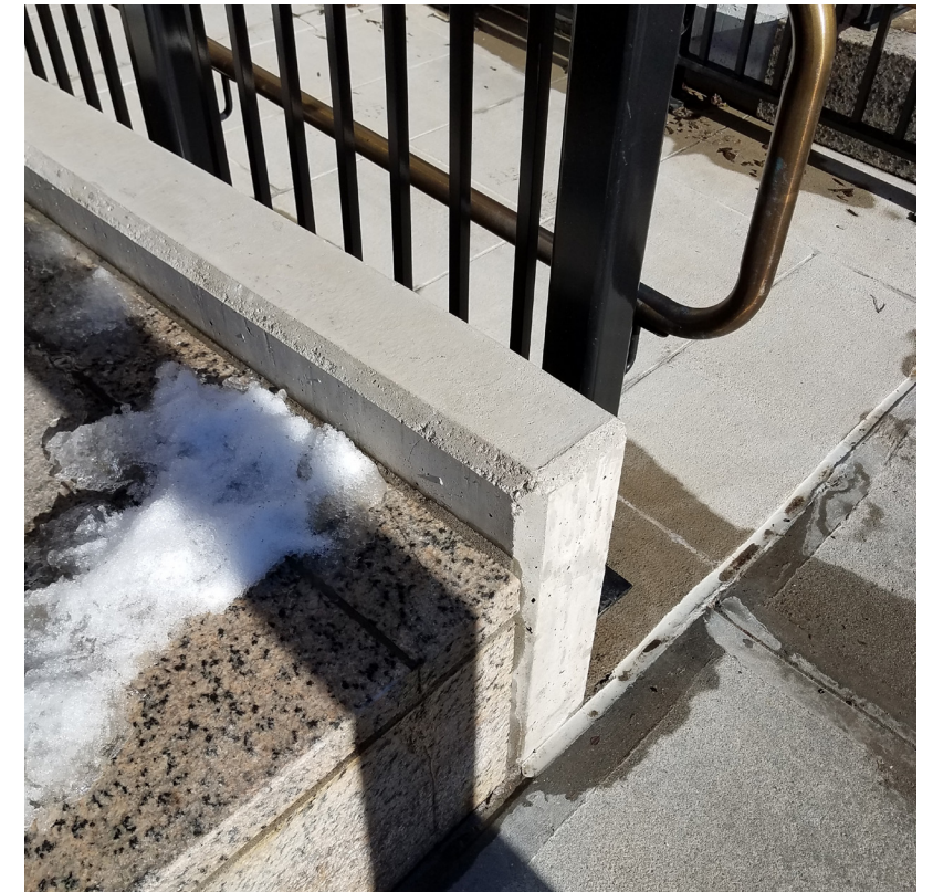
F: CONCRETE KNEE WALL AT SIDEWALK
