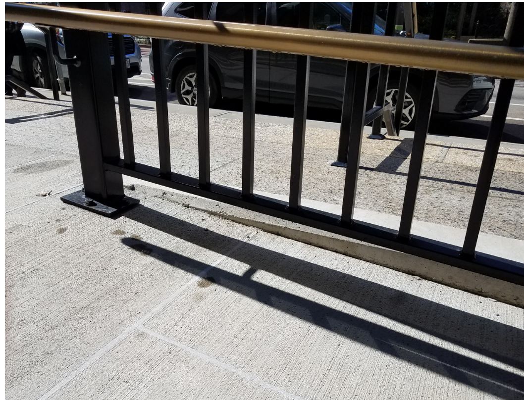
BB: RAMP TO TOP LANDING TRANSITION
