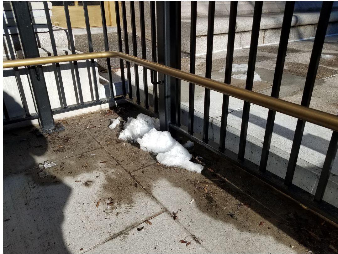
G: INTERIOR CORNER OF RAMP FROM STEP LANDING
