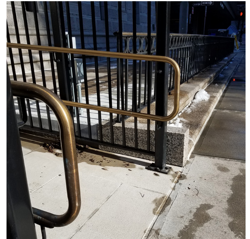
C: GRANITE KNEE WALL AT SIDEWALK
