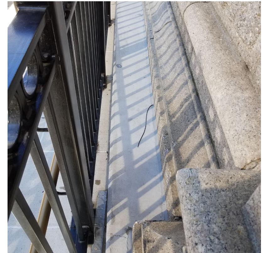
CC: CONCRETE SHELF BY FACADE
