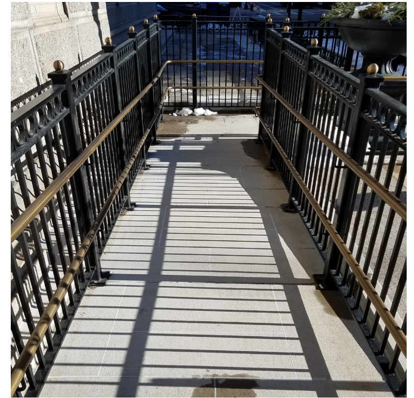
I: UPPER PORTION OF RAMP LOOKING TOWARD INTERMEDIATE LANDING
