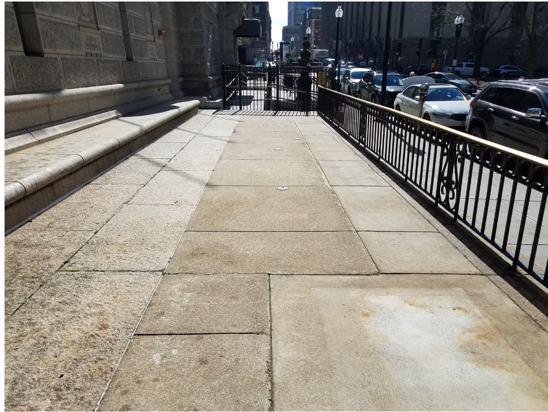
DD: TERRACE - STONE PAVERS AND POURED CONCRETE
