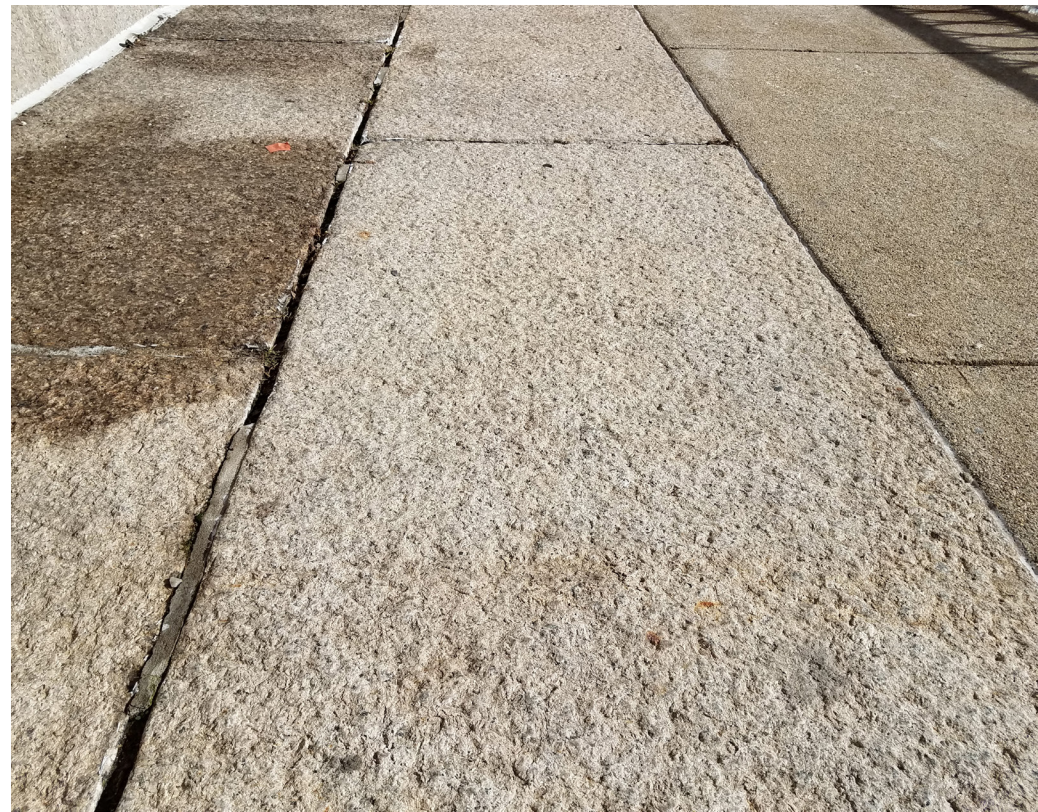
HH: CLOSE UP OF EXISTING FLAMED FINISH
