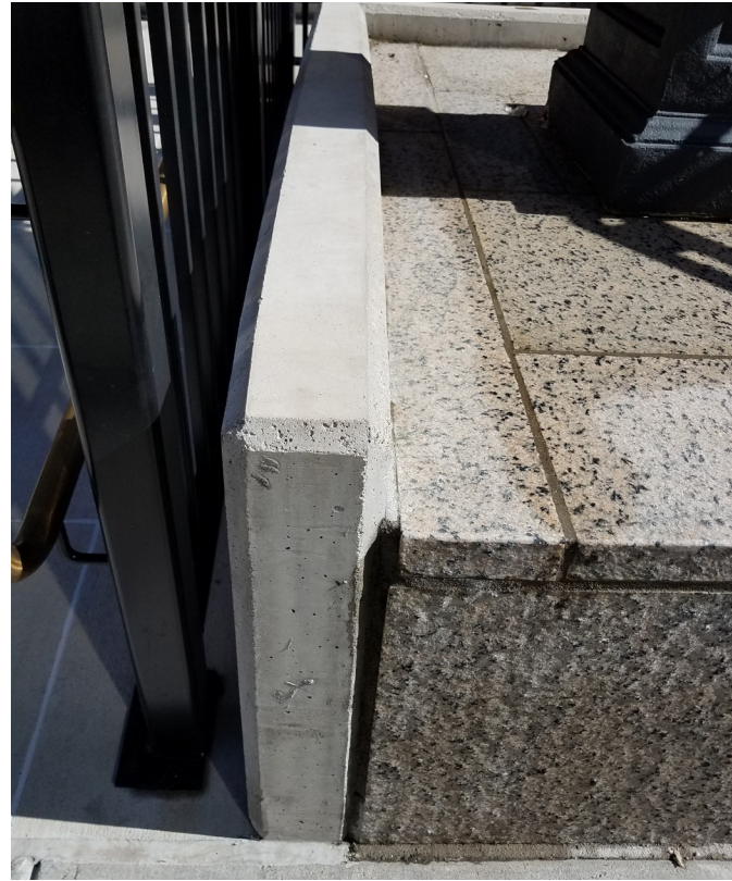
S: CONCRETE CHEEK WALL AT SIDEWALK
