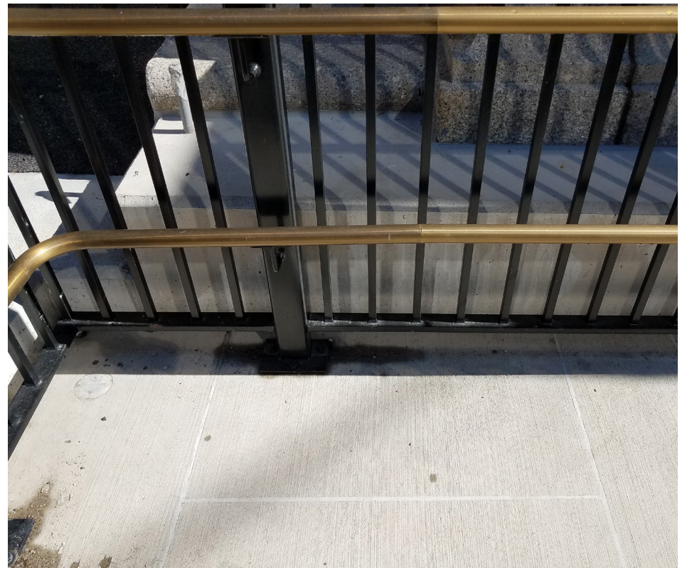
W: CONCRETE SHELF AT FACADE FROM UPPER PORTION OF RAMP
