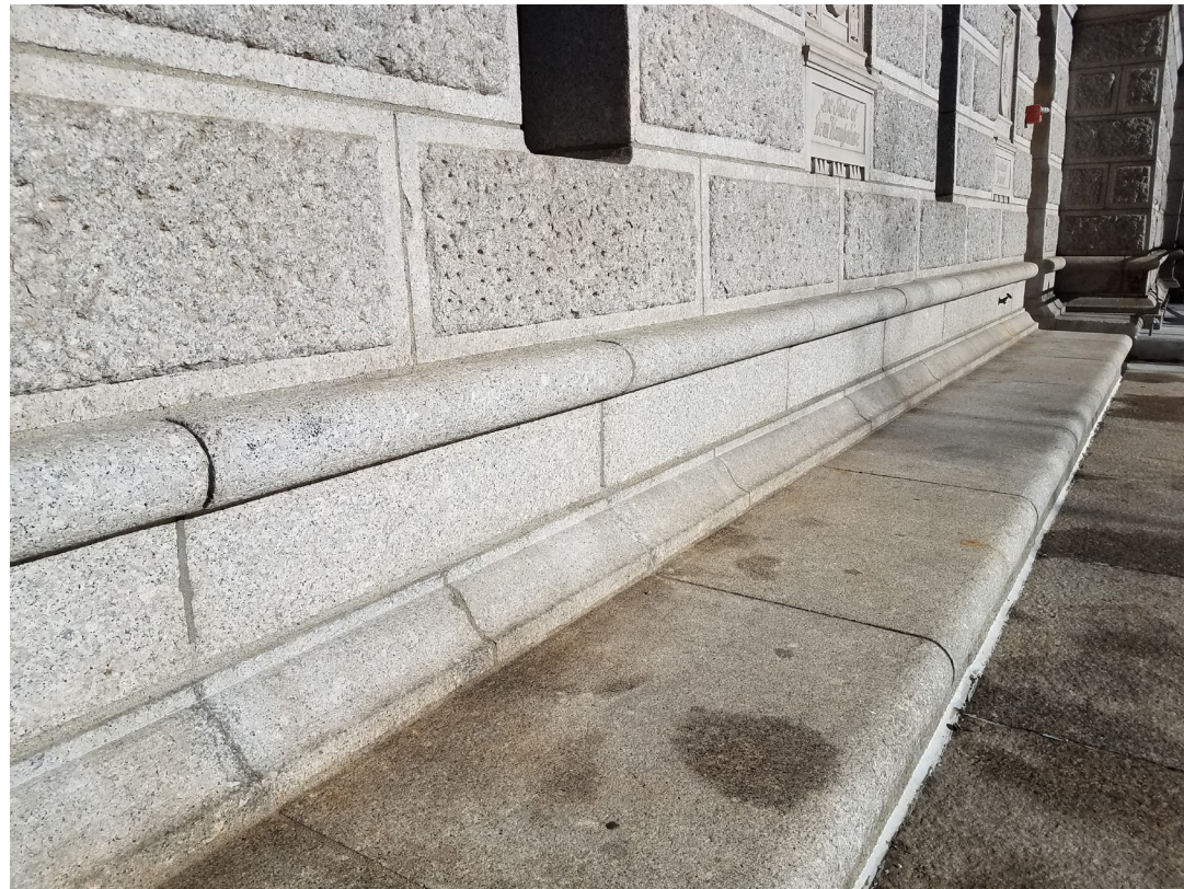
GG: EXISTING STONE BENCH ALONG FACADE
