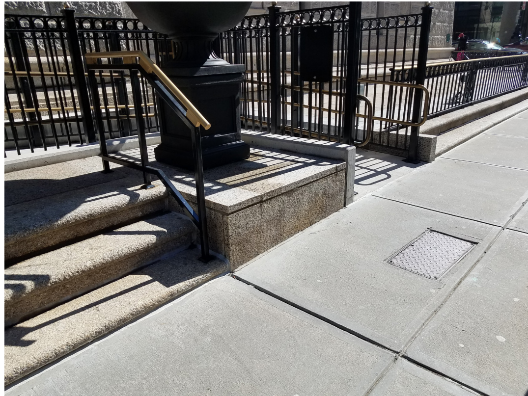
A: RAMP, STEPS AND STEP LANDING FROM SIDEWALK
