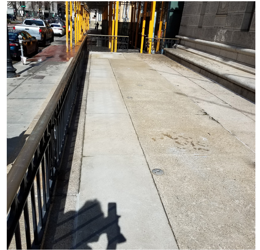
FF: NEW POURED CONCRETE ALONG EXISTING FENCE
