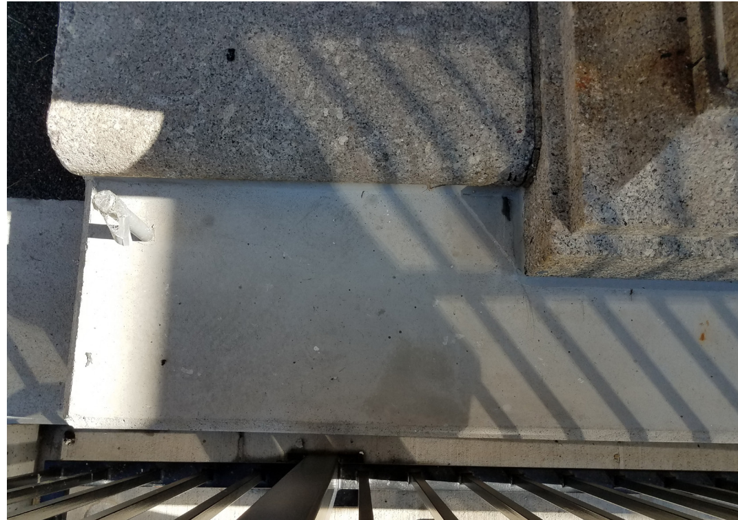
Y: CONCRETE SHELF BY FACADE
