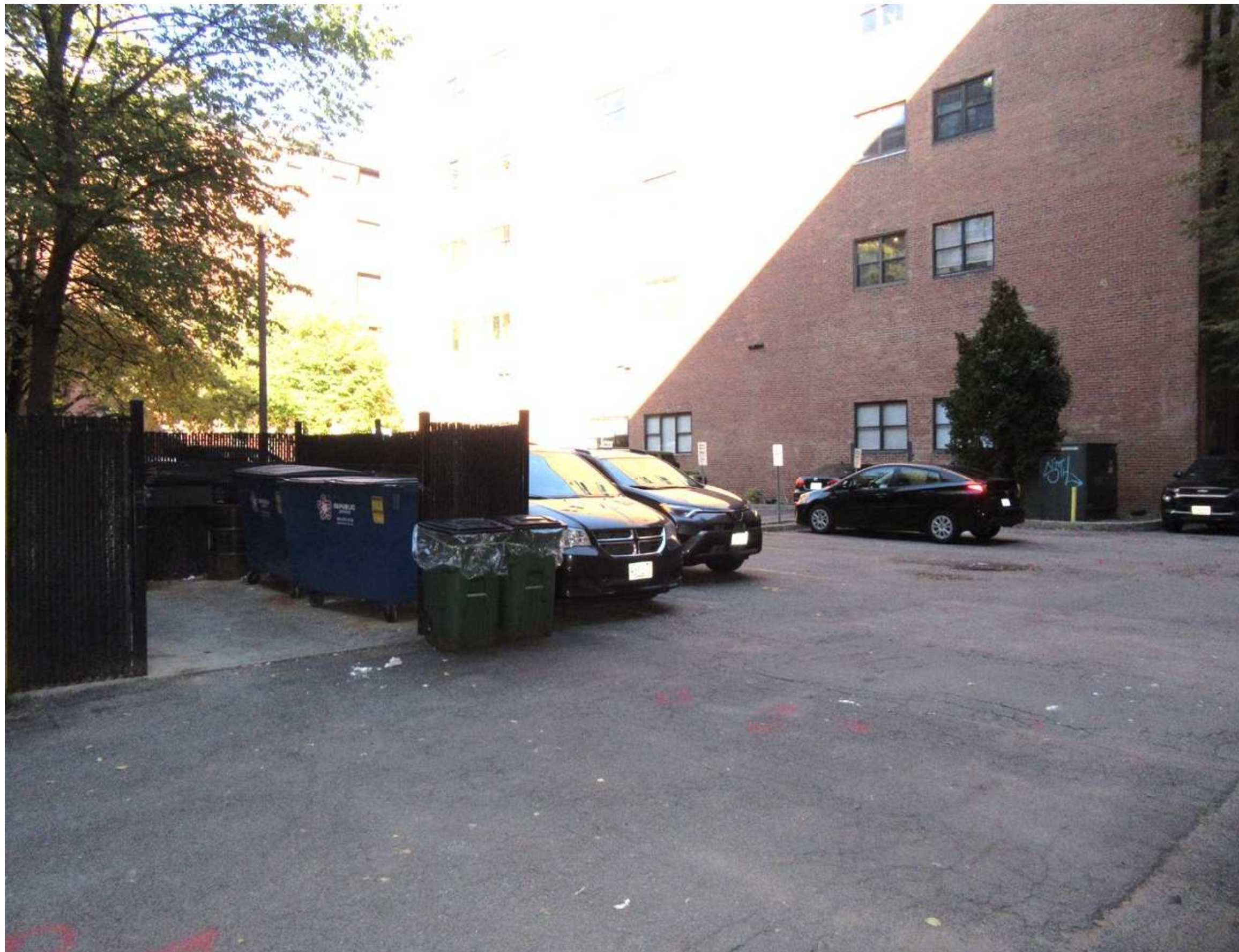
PHOTO 4 - 11 SLEEPER STREET PARCEL - TRANSFORMER AT FAR RIGHT - VIEW NORTHEAST
