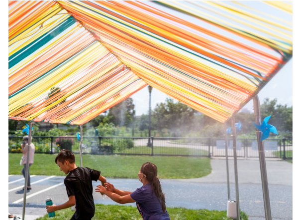
Misters installed under tents at the East Boston Branch
