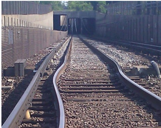
Heat kink along the Orange Line rail tracks
