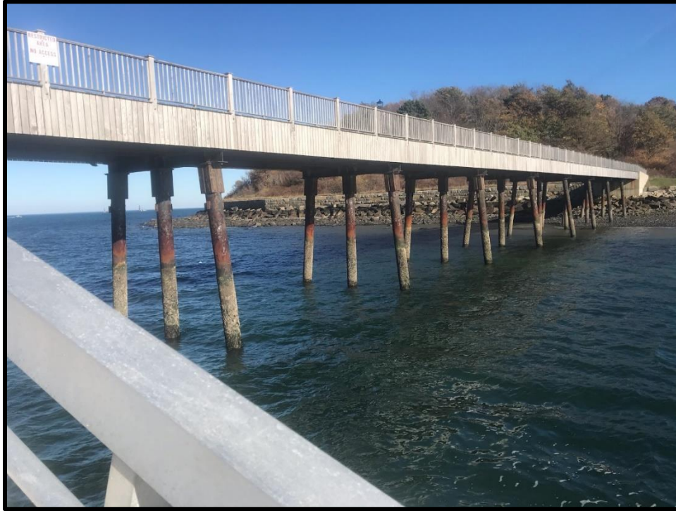
Photograph 3: Existing Conditions of the Long Island Pier (looking East from gangway)
