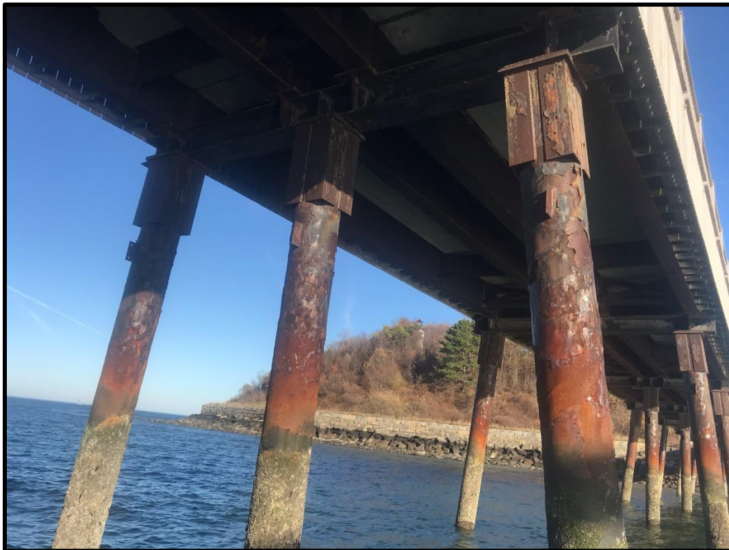
Photograph 2: Existing Conditions of the Pier Supporting Pipe Piles (looking East)
