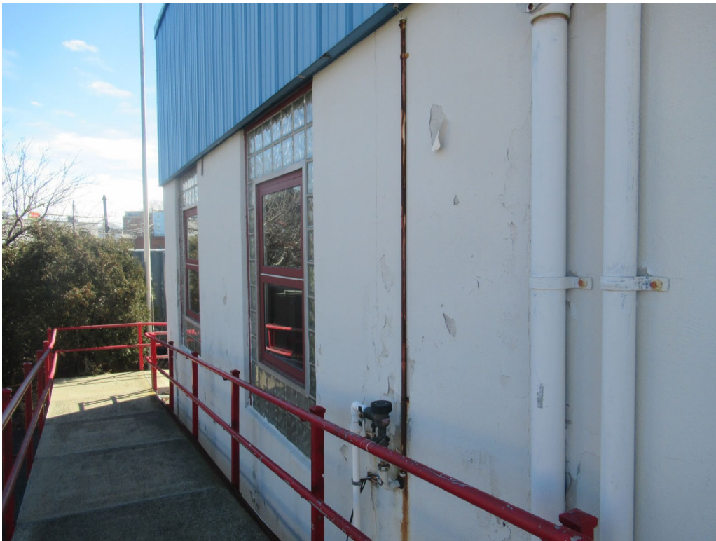
8. North elevation, looking east
