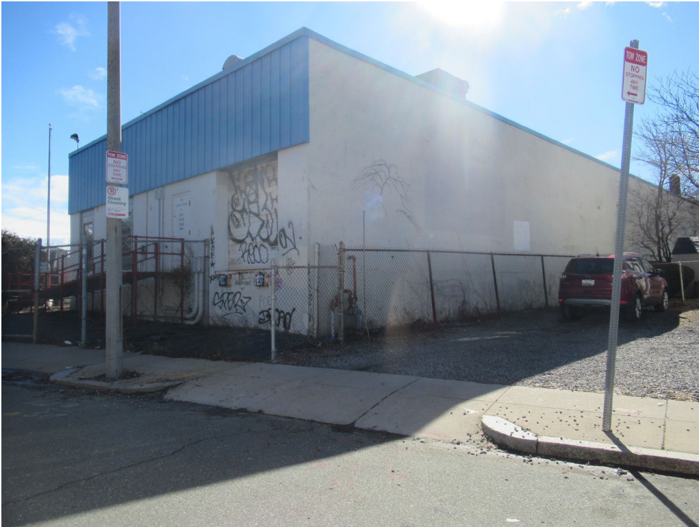
10. North and west elevations, looking southeast
