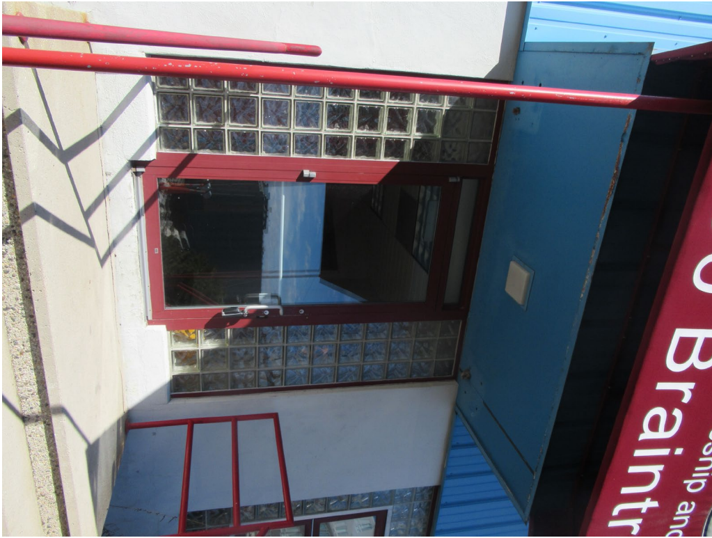
11. Main entryway detail
