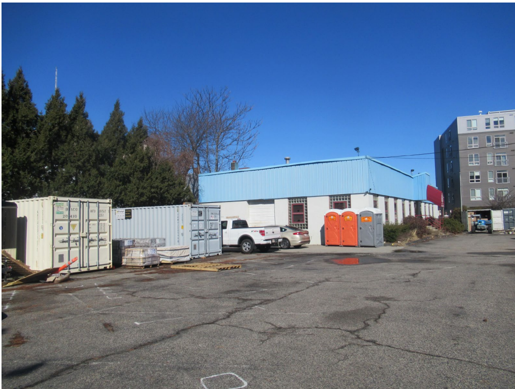
2. South and east elevations, looking north
