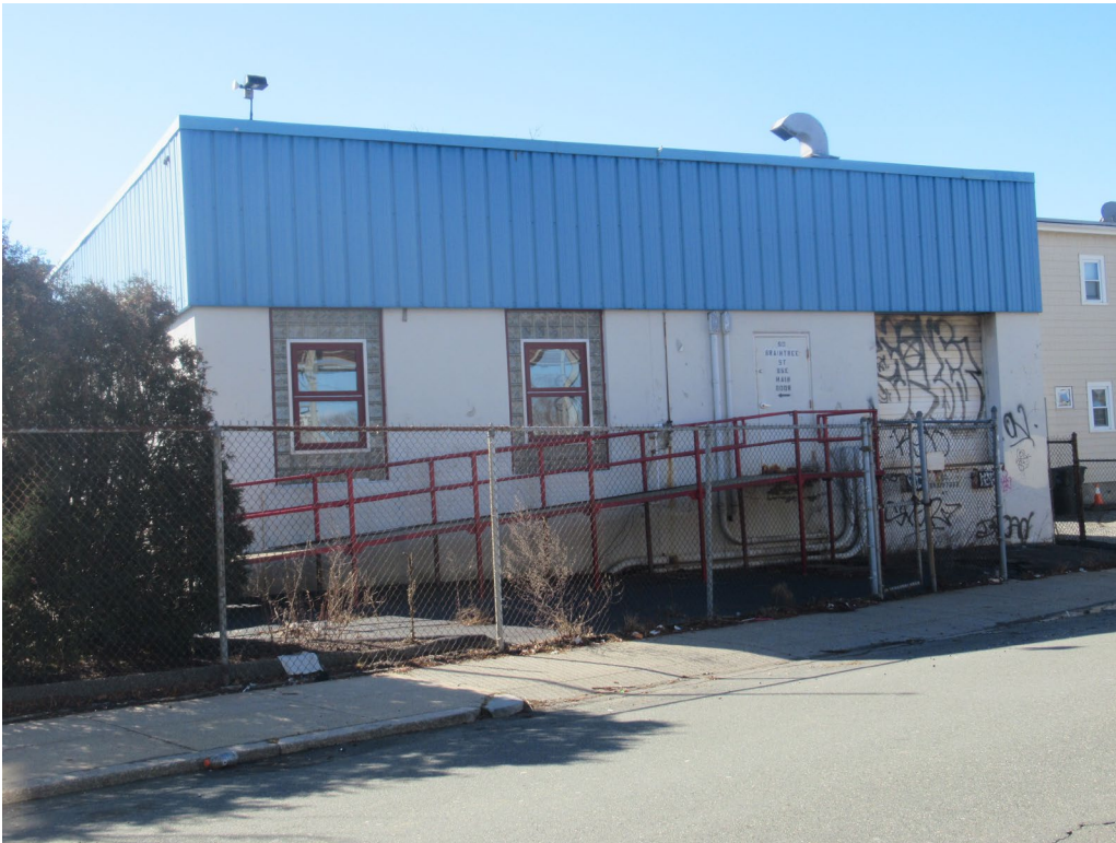
9. North elevation, looking southwest
