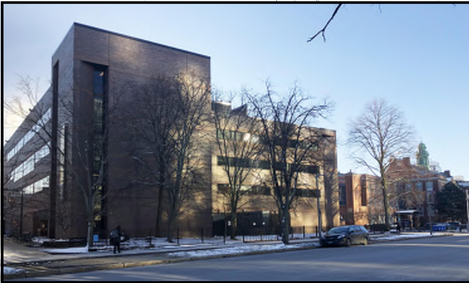
1. PARK SCIENCE NW CORNER. TAKEN FROM AVENUE LOUIS PASTEUR FAR SIDEWALK
