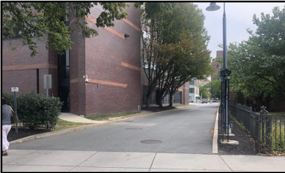
4. PARK SCIENCE SOUTH ELEVATION. TAKEN FROM SERVICE DRIVE LOOKING EAST
