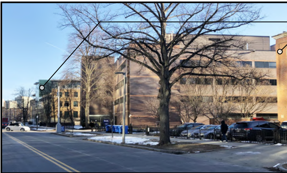
3. PARK SCIENCE SW CORNER. TAKEN FROM AVENUE LOUIS PASTEUR. ADJACENT BUILDINGS SHOWN FOR CONTEXT; SIMMONS UNIVERSITY LEFAVOUR & BOSTON LATIN SCHOOL
