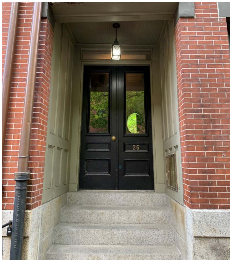
Photo of Existing Vestibule at 26 Hanson Street
