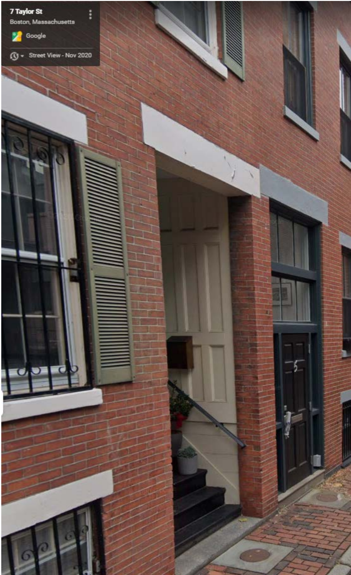
Representative Photo of Similar Handrail at 7 Taylor Street
