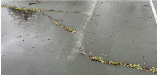
Cracked, uneven pavement with drainage issues
