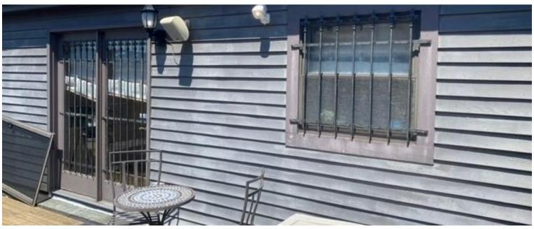
DUE TO SAFETY CONCERNS (DECK IS ACCESSIBLY FROM STREET LEVEL DUE TO STAIRS) WE WILL INSTALL NEW DOORS, SAME SIZE AND STYLE MADE OF FIBREGLASS AND REINSTALL THE BARS MORE SECURELY. REPAINT ONLY FOR WINDOW BARS
