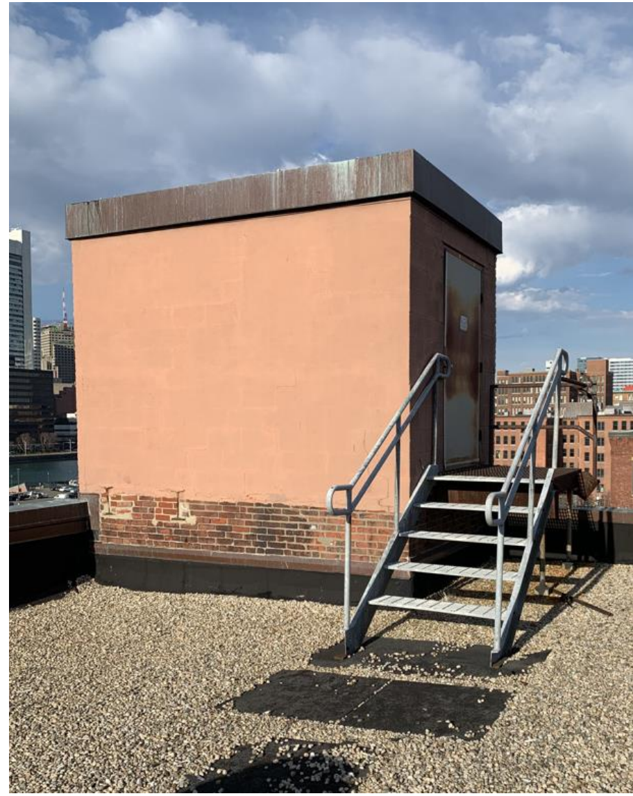
Existing Elevator Machine Room
