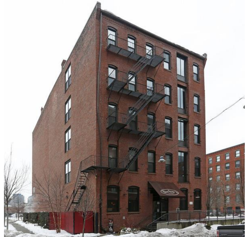
Existing Fire Escape View - Channel Center Street
