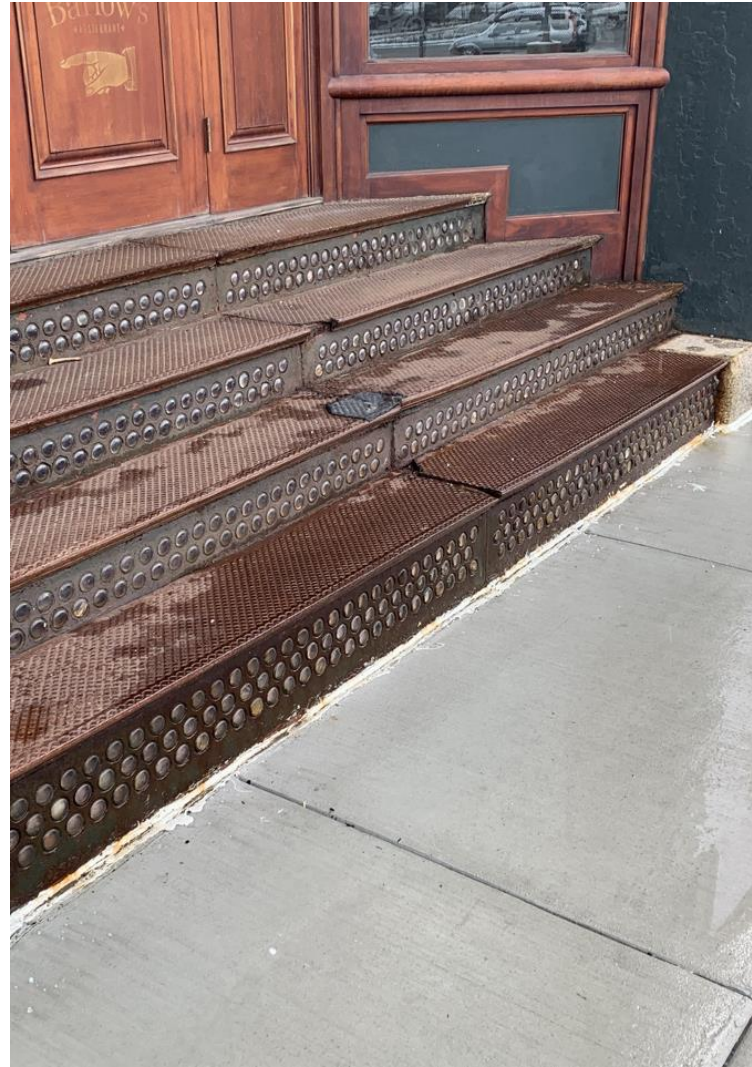
Front Step Restoration/wood refinishing
