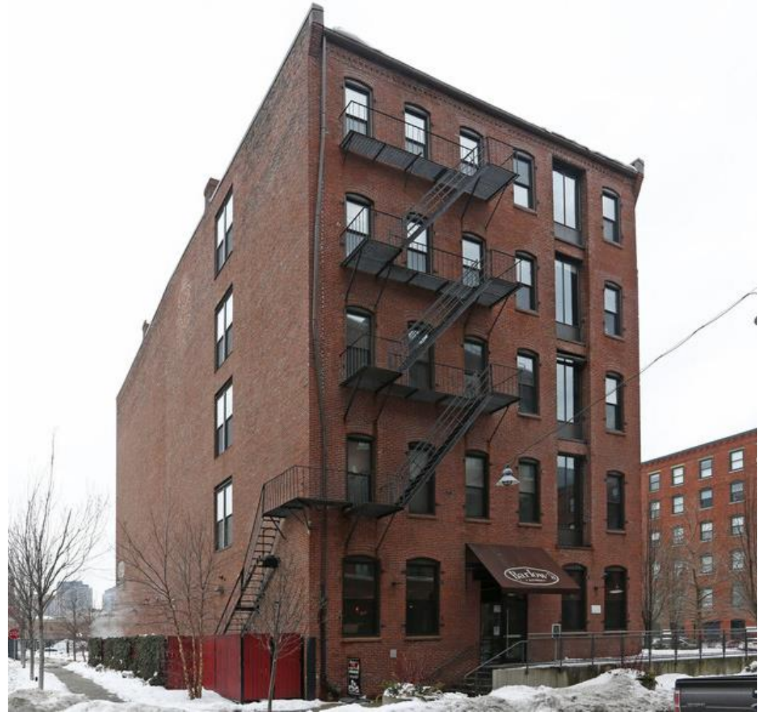
Exterior view from Channel Center
