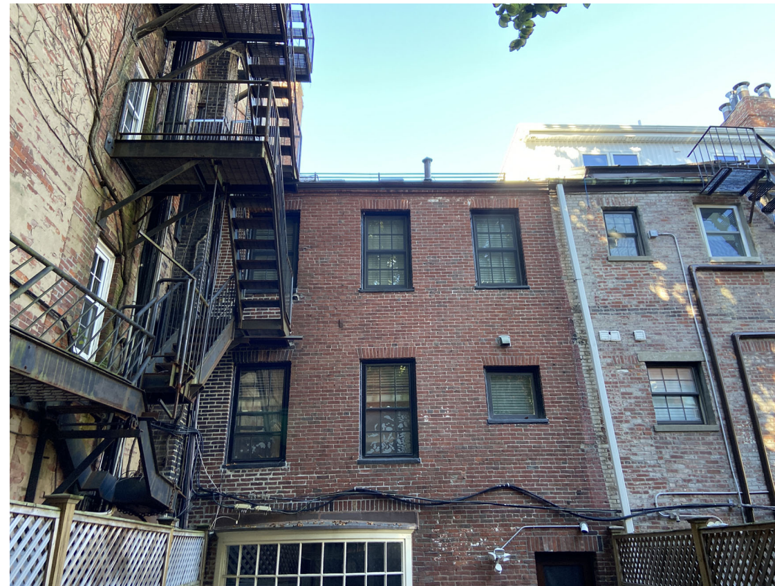
VIEW TO EXISTING REAR ELEVATION ROOF
