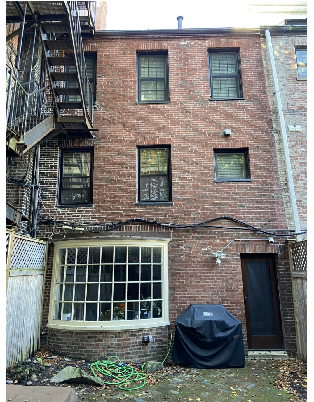
EXISTING REAR FACADE
