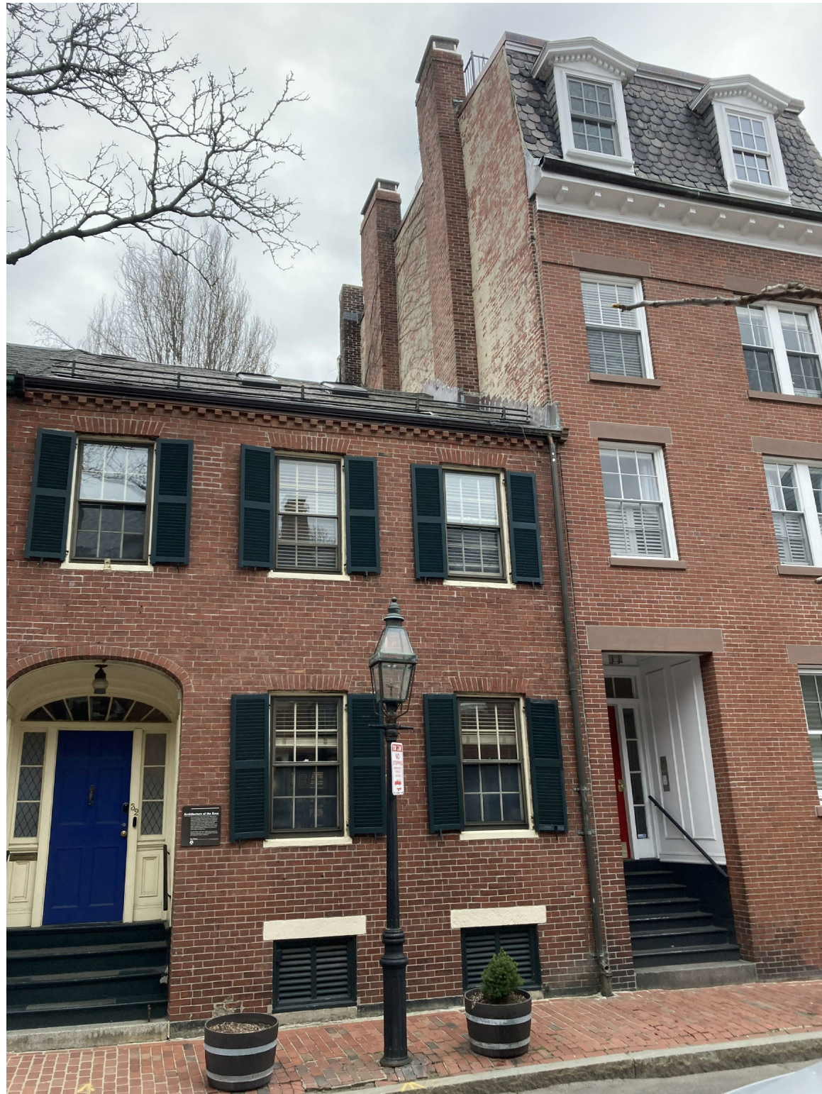
EXISTING STREET FACADE
