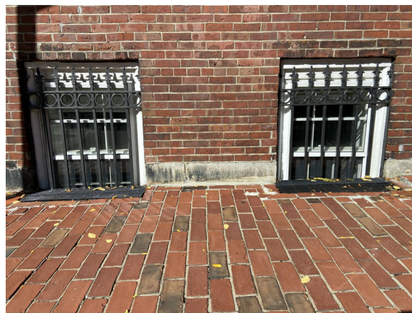
PHOTO OF GROUND LEVEL WINDOWS AT NEIGHBORING HOUSES
