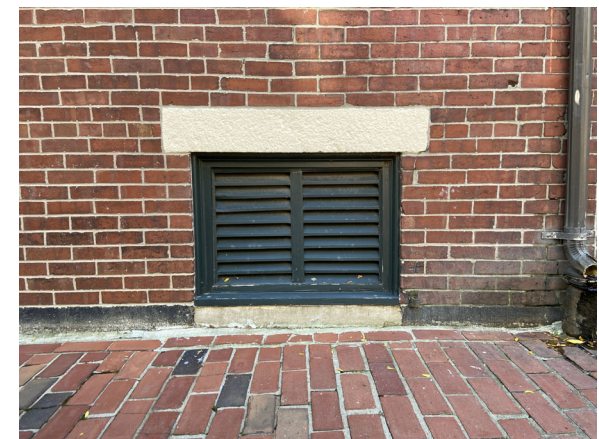
PHOTO OF EXISTING LOUVRE ON STREET FACADE
