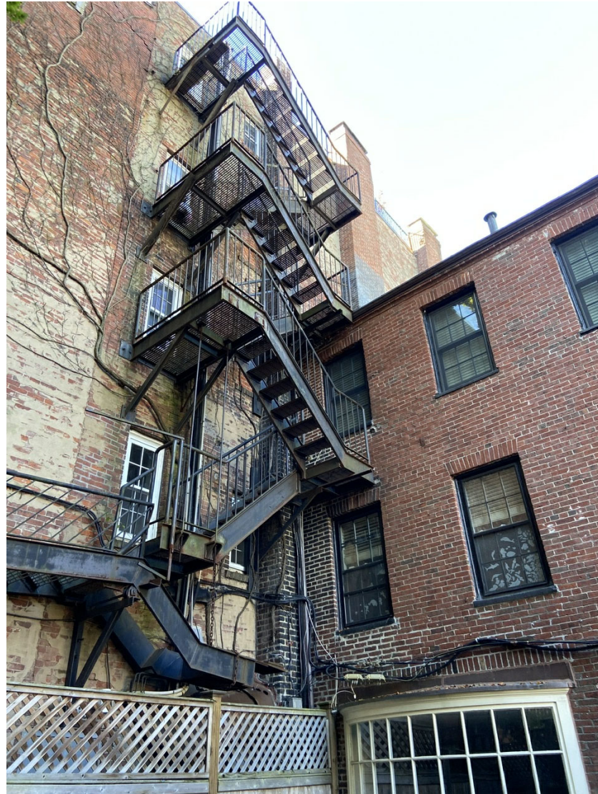
EXISTING FIRE ESCAPE
