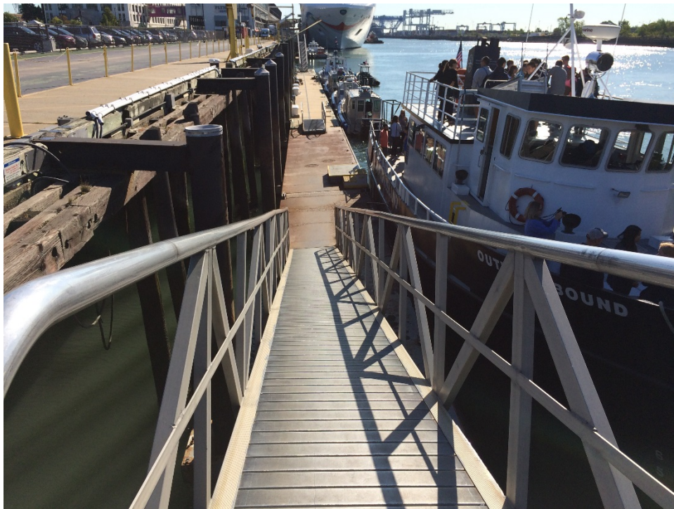
Photograph No.: 4 Thompson Island ramp and float with ferry. View looking east in Reserved Channel.
