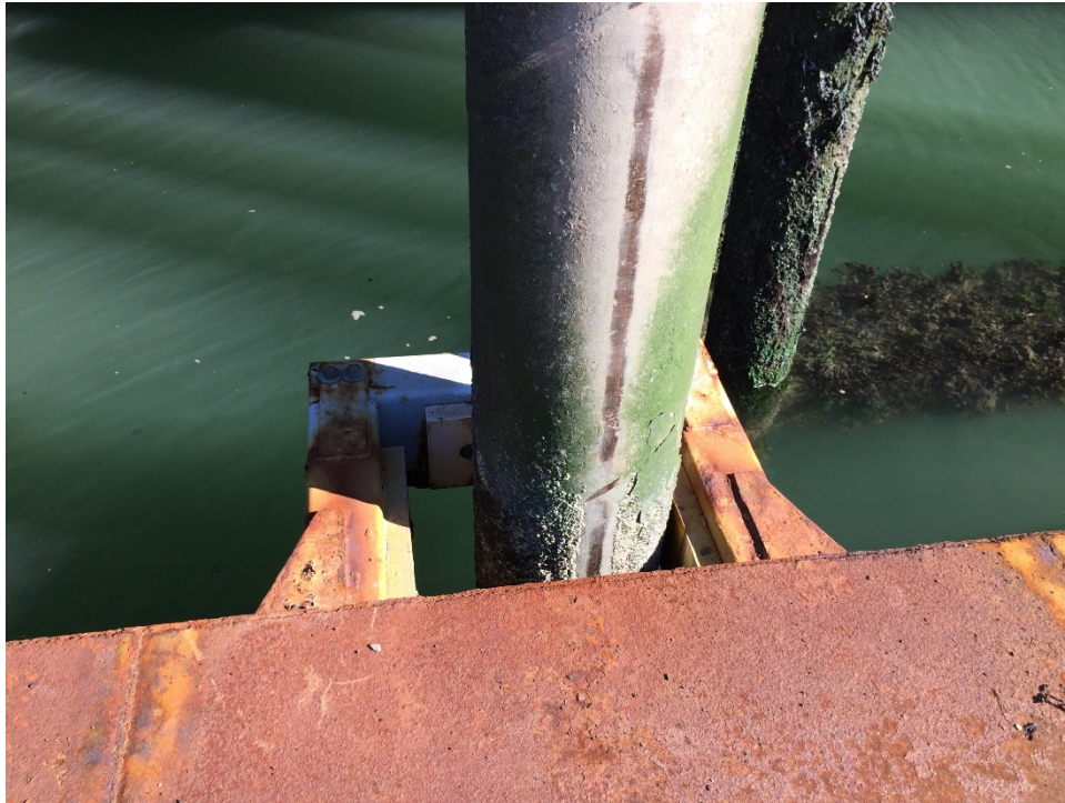
Photograph No.: 7 Thompson Island float and pile connection.
