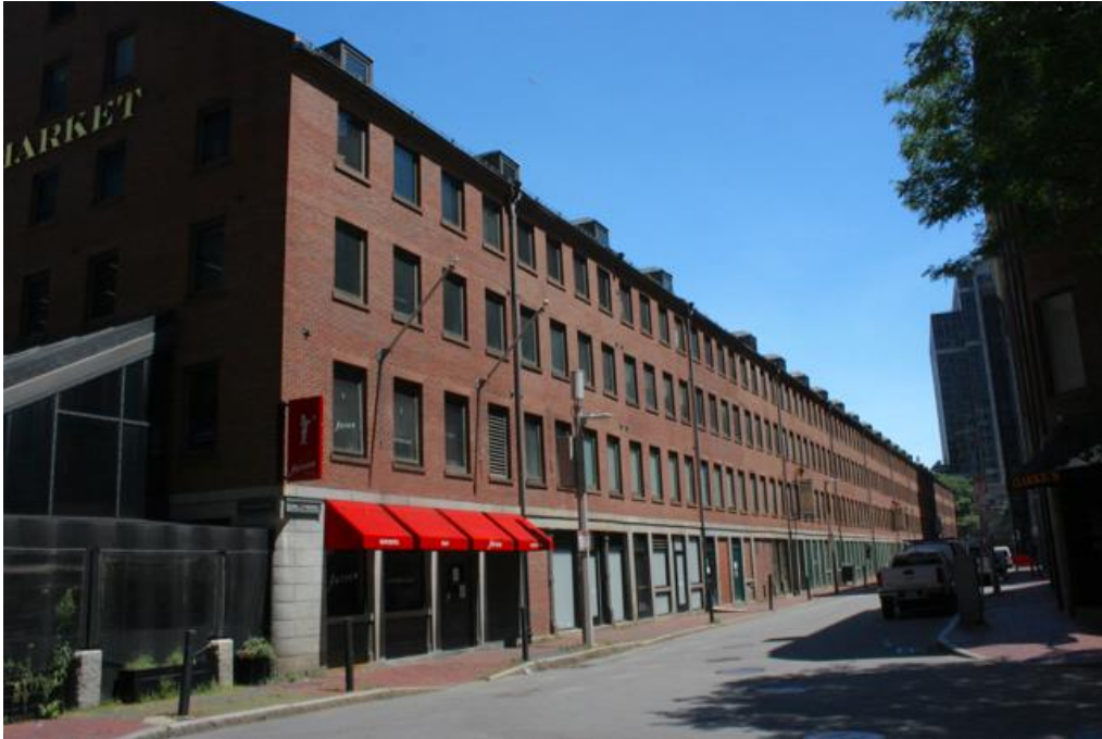
Figure 16. Back (south) elevation, looking east.
