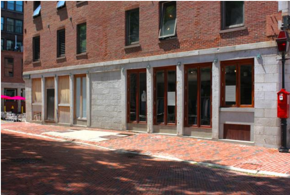
Figure 13. East elevation: Detail of first floor.
