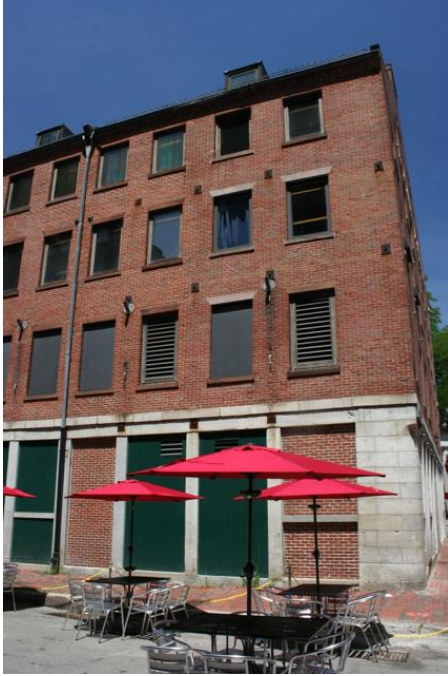
Figure 14. Back (south) elevation: East end of block with typical granite storefront.
