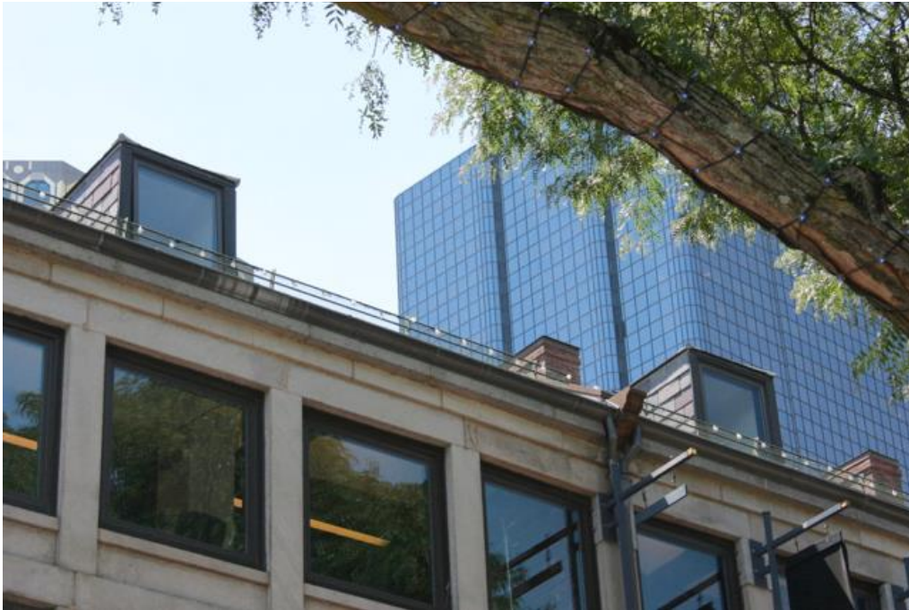
Figure 9. Façade (north elevation): Detail of roof edge.
