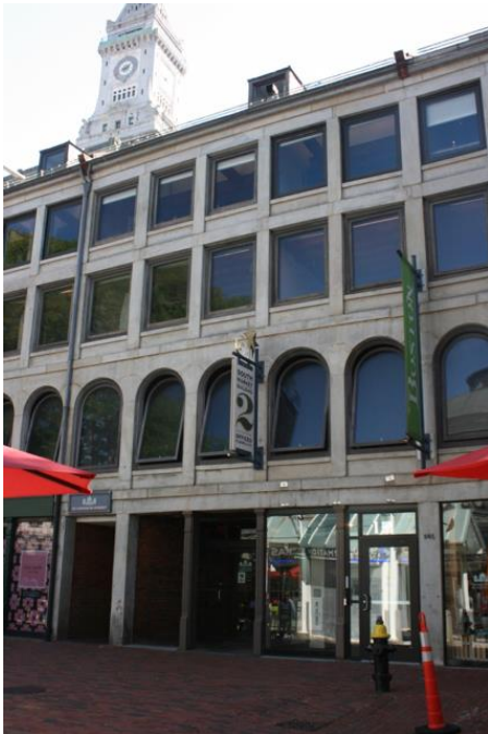
Figure 7. Façade (north elevation): Five-bay unit in center of block (includes Entrance 2 to upper levels of the block).
