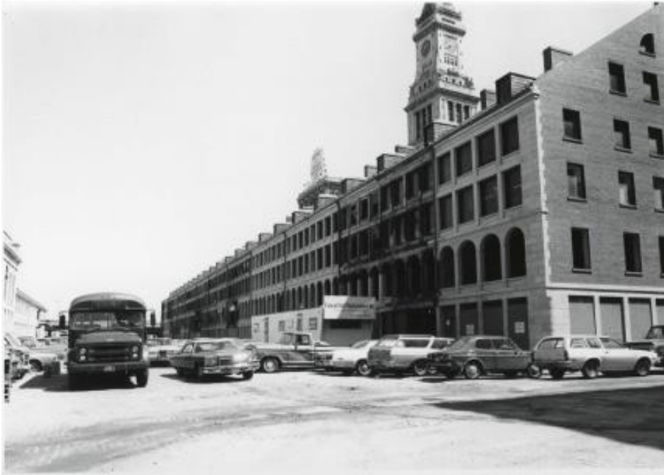
Historic Image 4. South Market undergoing rehabilitation, 1975. View east. Courtesy of U.S. Department of the Interior, National Park Service.
