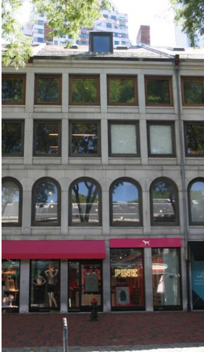
Figure 6. Façade (north elevation): Typical four-bay building unit.
