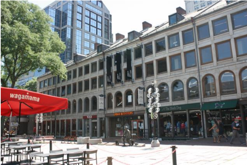
Figure 4. Façade (north elevation): East end of block, looking southeast.
