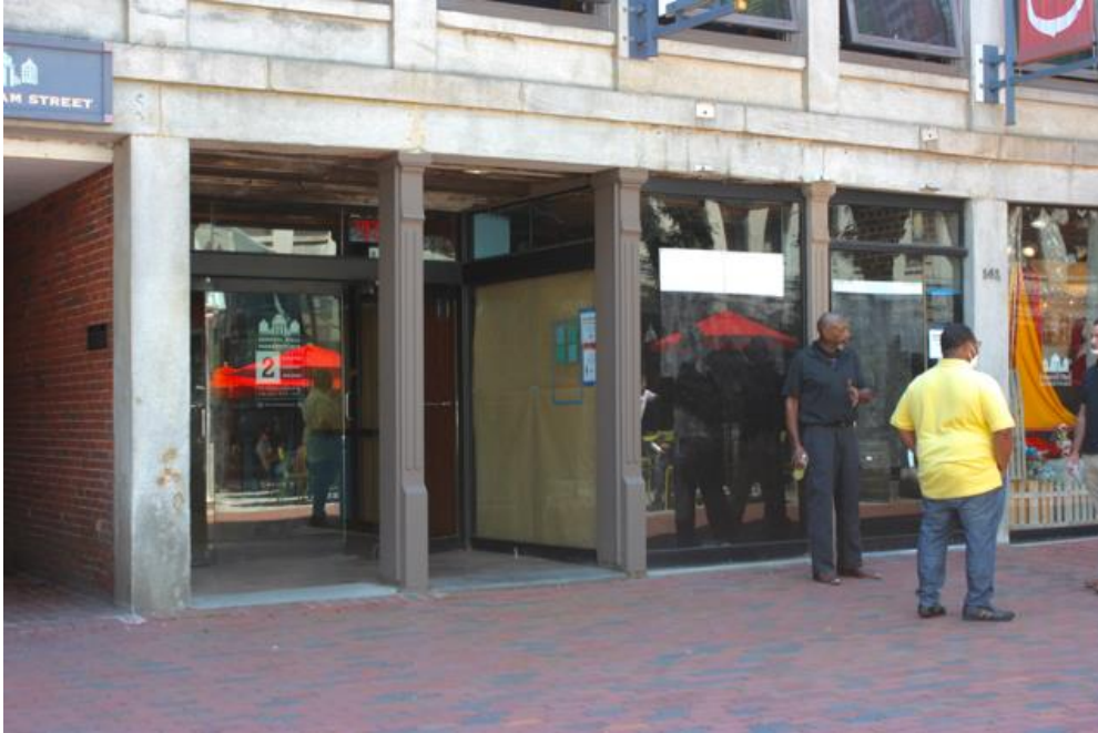
Figure 10. Façade (north elevation): Detail of storefront with cast iron piers.
