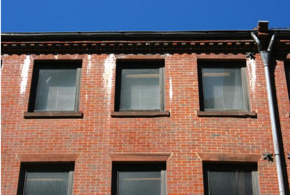
Figure 18. Back (south) elevation: Detail of windows and roof edge.
