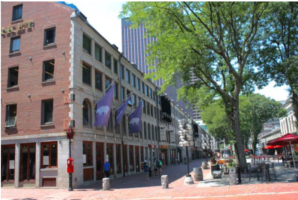
Figure 5. Façade (north elevation): East end of block, looking southwest.
