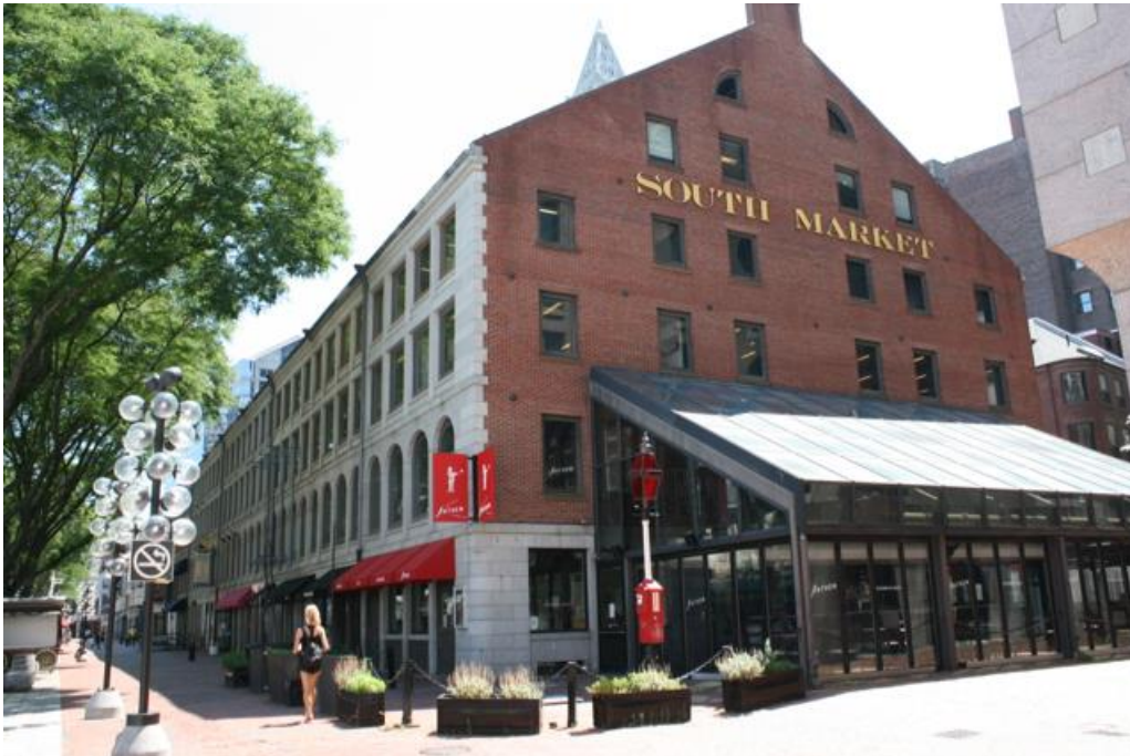
Figure 2. Façade (north) and west elevations, looking southeast.
