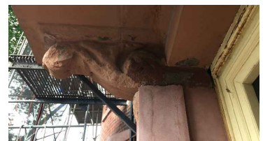
EXISTING BRACKET TO BE RESTORED
