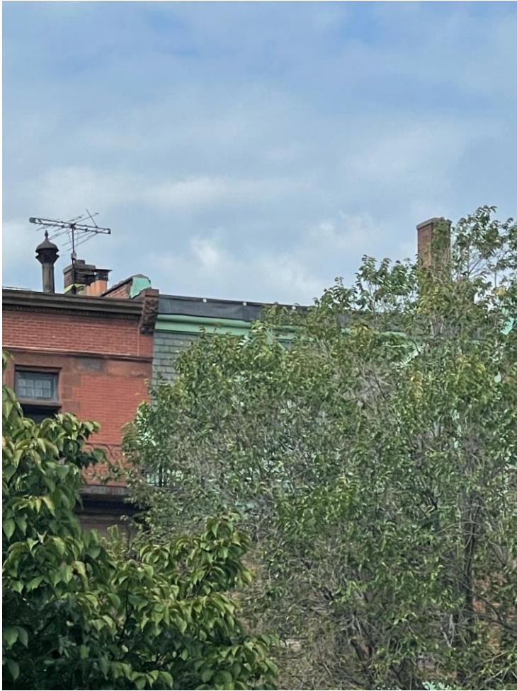
Exhibit 1: Front of Building Sidewalk view
