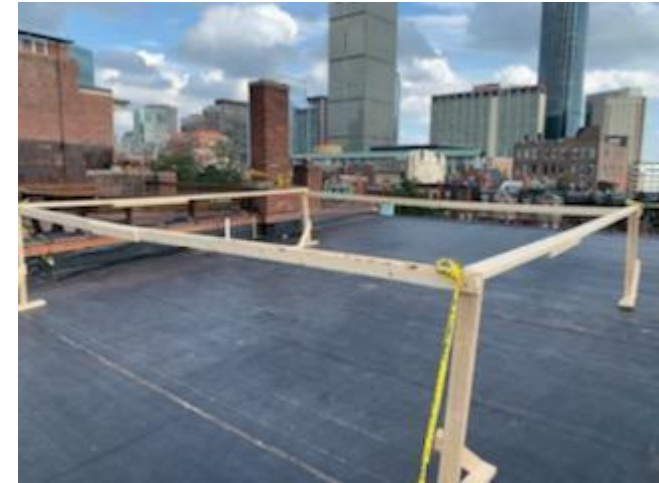
Exhibit 6: Deck South-East View
