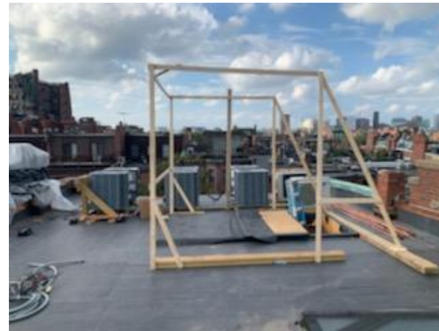
Exhibit 10: Headhouse North facing
