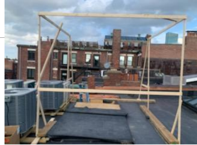
Exhibit 8: Headhouse West Facing
