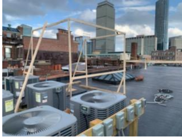
Exhibit 8: Headhouse South-East Facing
