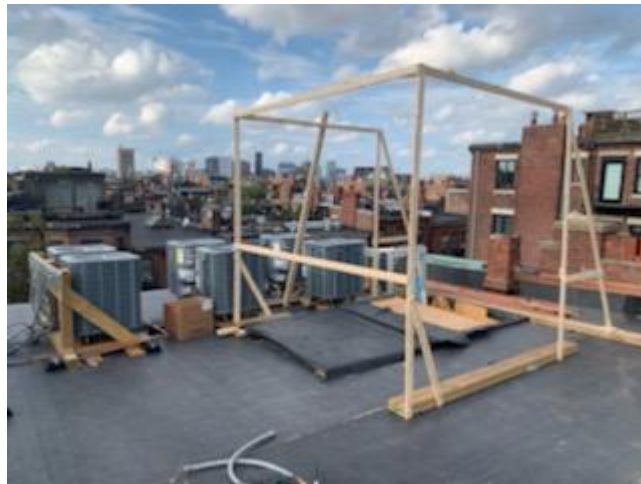
Exhibit 9: Headhouse North Facing
