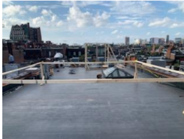
Exhibit 5: Deck North View facing Public Alley
