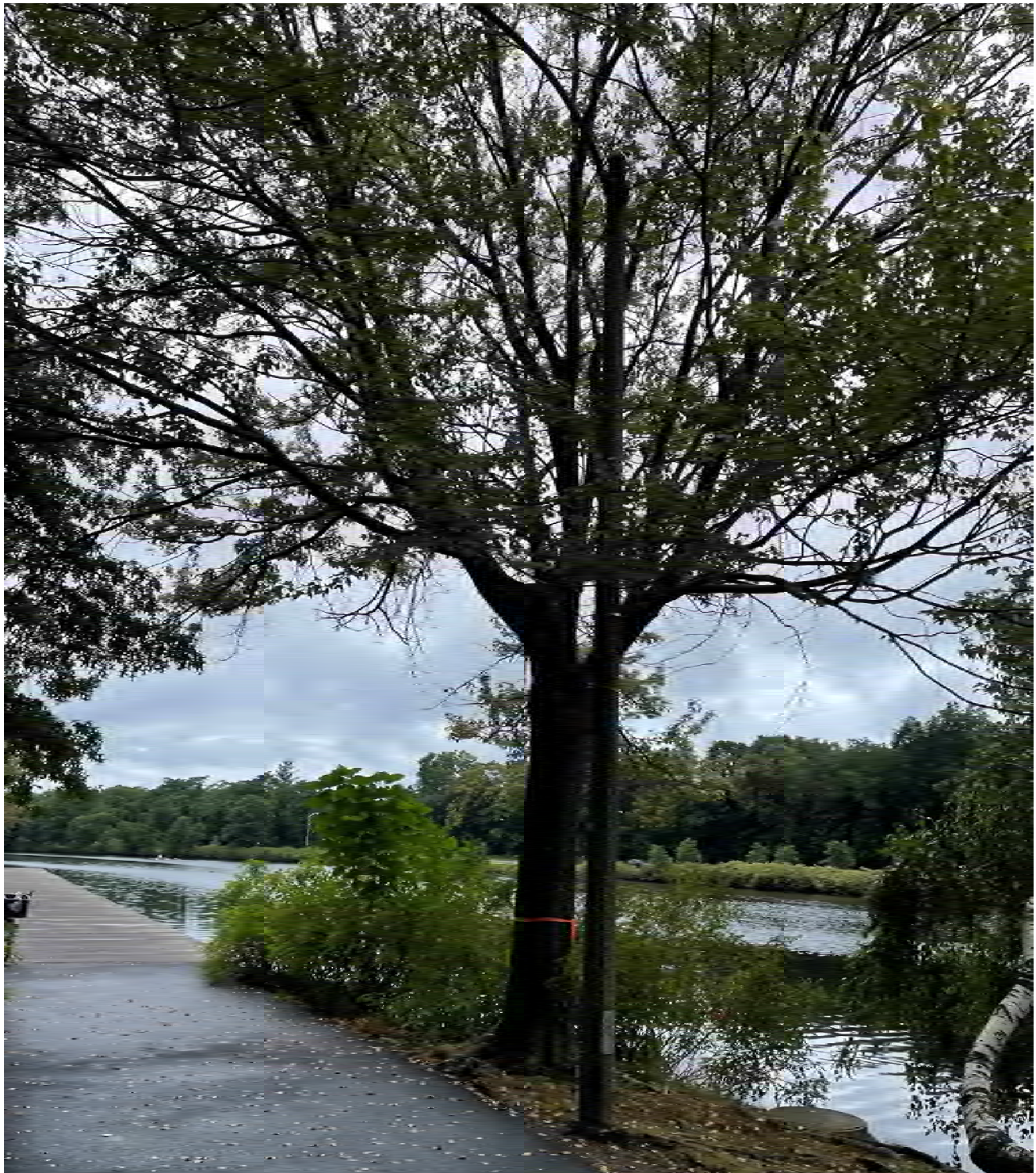
Photo #3: View of hazardous tree “C,” a red maple in poor health located at the top of Bank.
