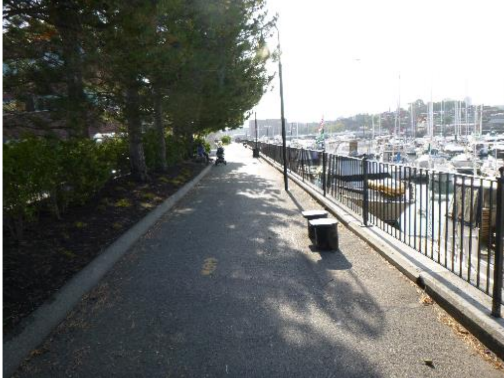
Photo 3: Typical view of the Harborwalk behind the sheet pile bulkhead.
