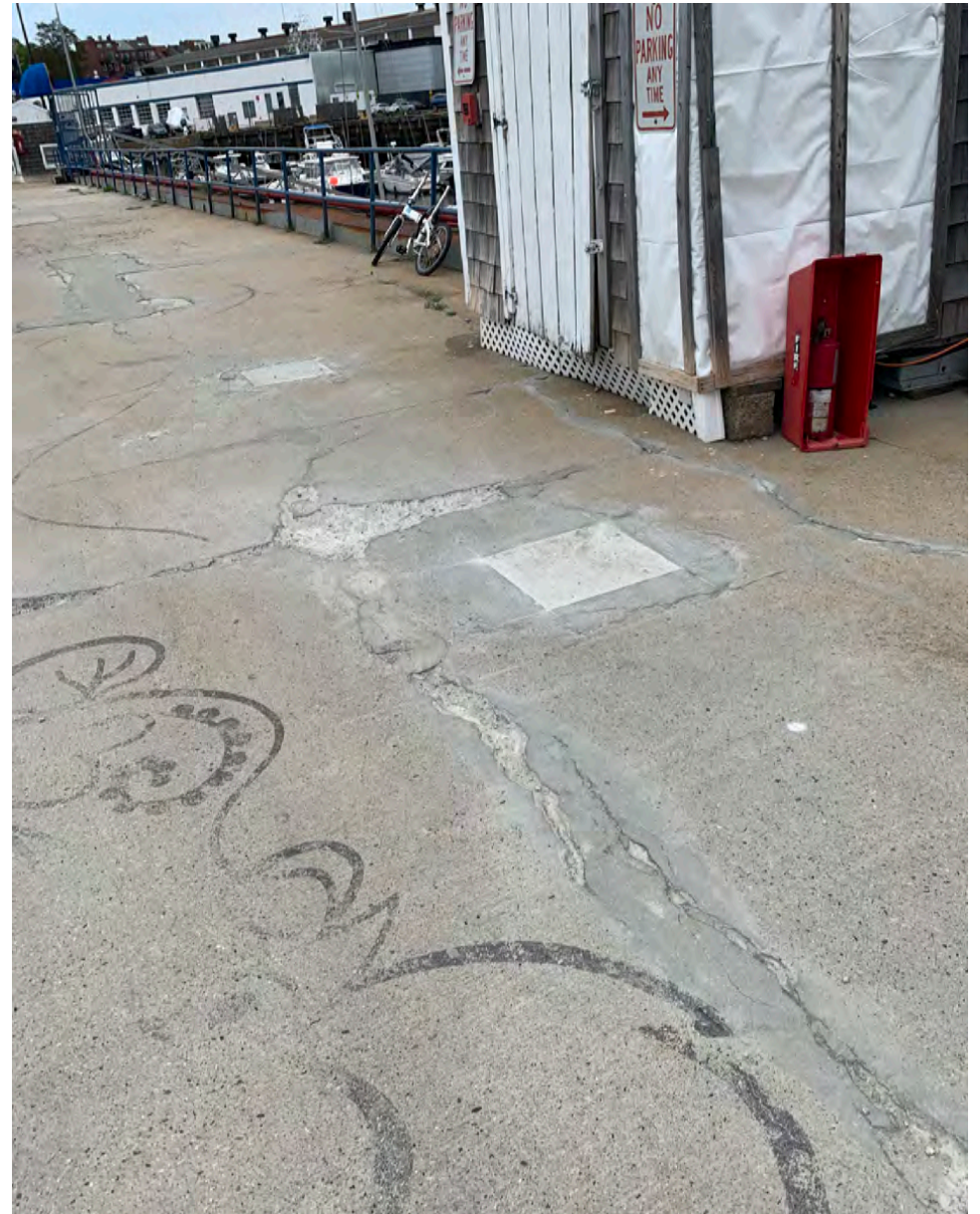
Looking north at the repaired deck section of Pier #1.
