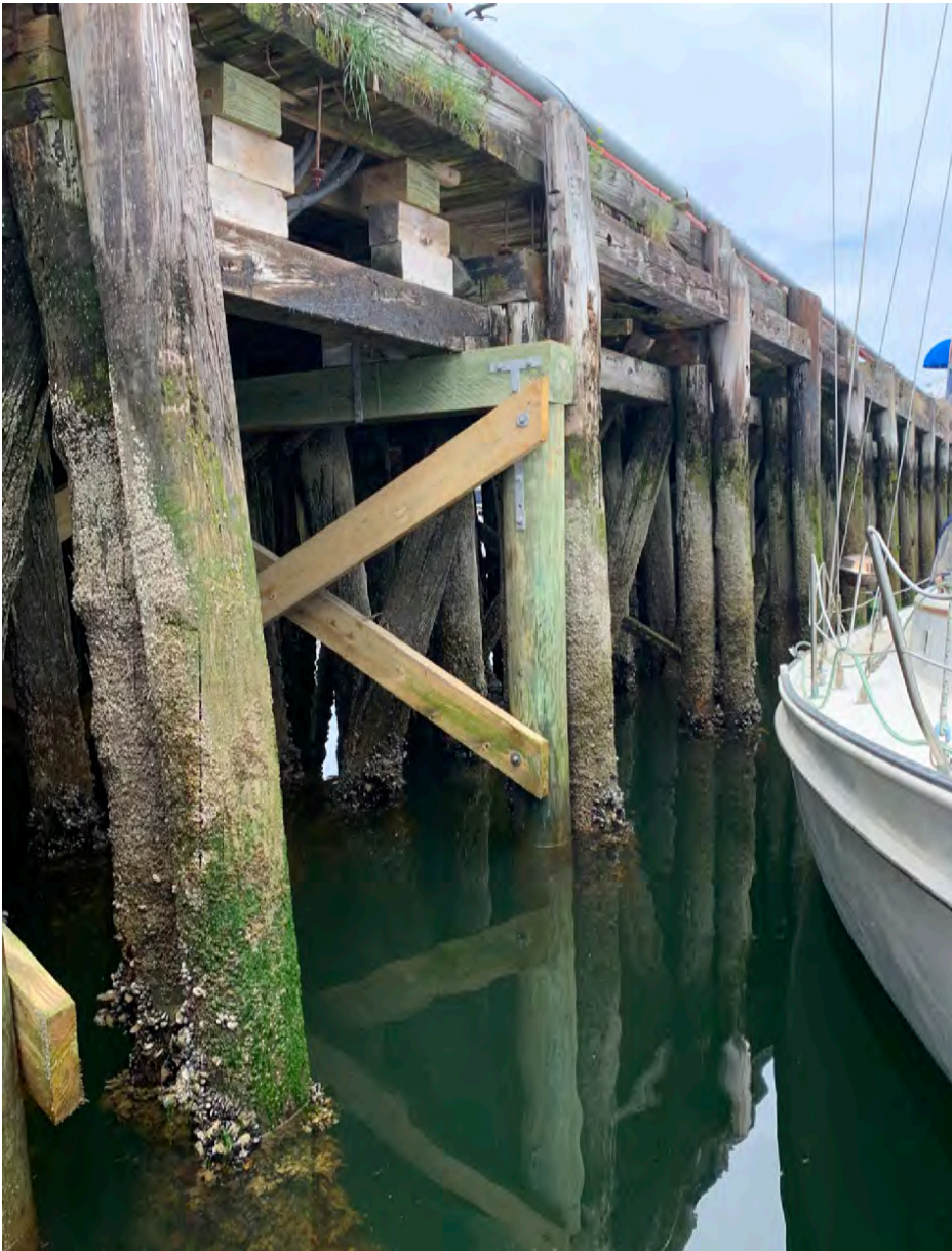
Looking north at completed work on the Project Site.
