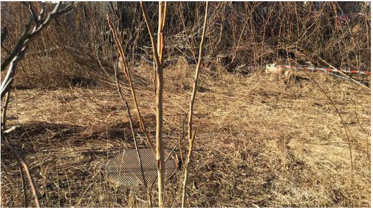
Photo #10: View of the manhole and location of the vault for the existing 54” tide gate, located along the pathway footprint and owned by DCR. Facing west.
