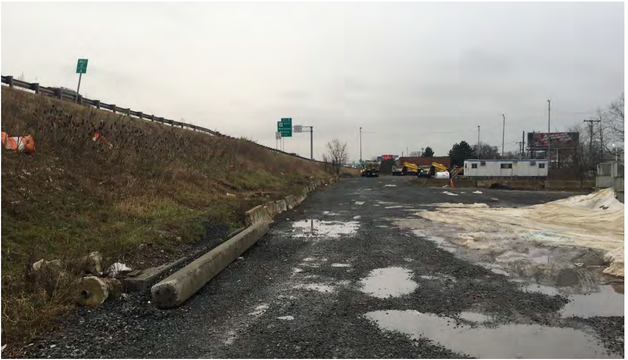
Photo #8: View of the western embankment of I-93 from Victory Road. The southern section of the multi-use path is proposed parallel to the expressway in LSCSF. Facing south
