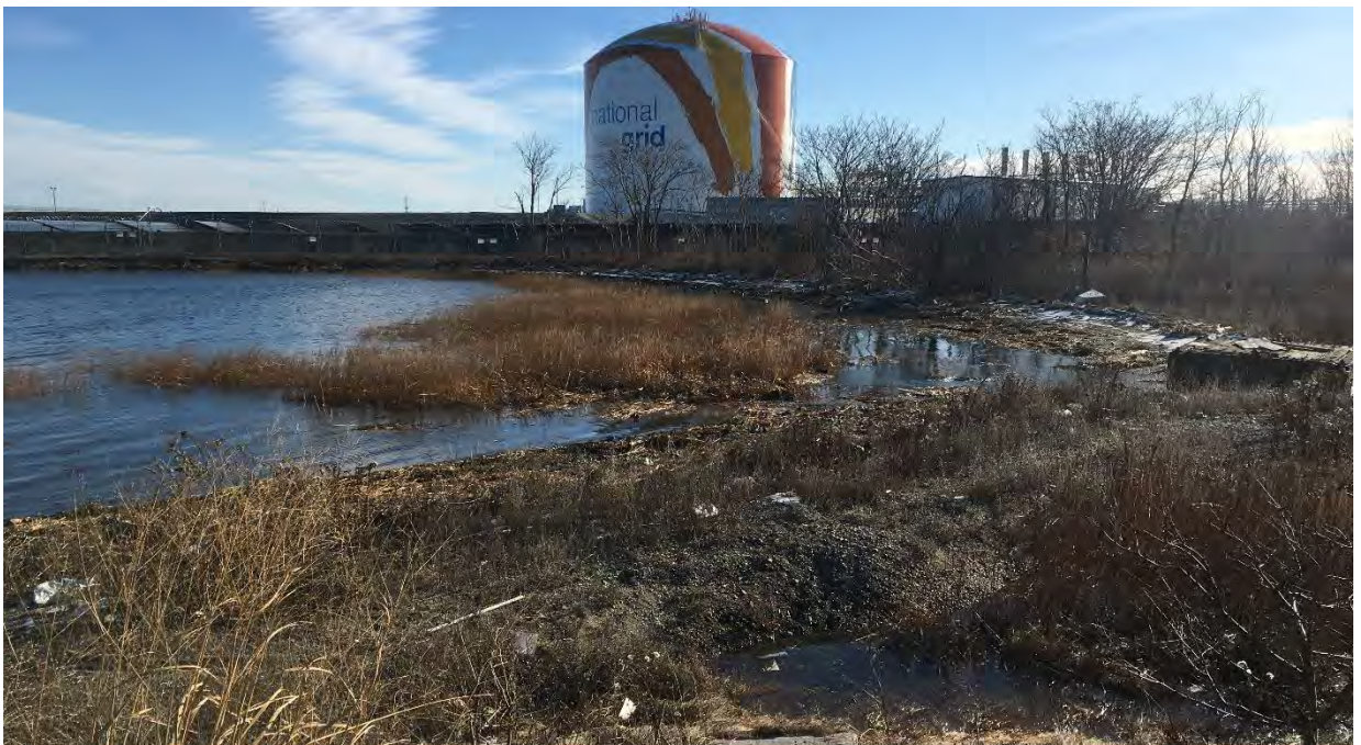
Photo #4: View towards the National Grid energy facility and LNG storage tank from the exit ramp embankment, in the area of the proposed boardwalk. Facing southeast.
