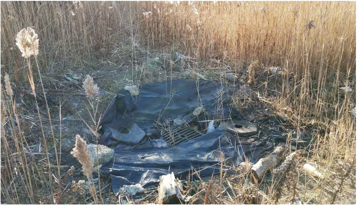
Photo #12: View of an existing stormwater catch basin and catchment area in the vicinity of the proposed path. A Phragmites stand is present but hydric soil was not encountered.
