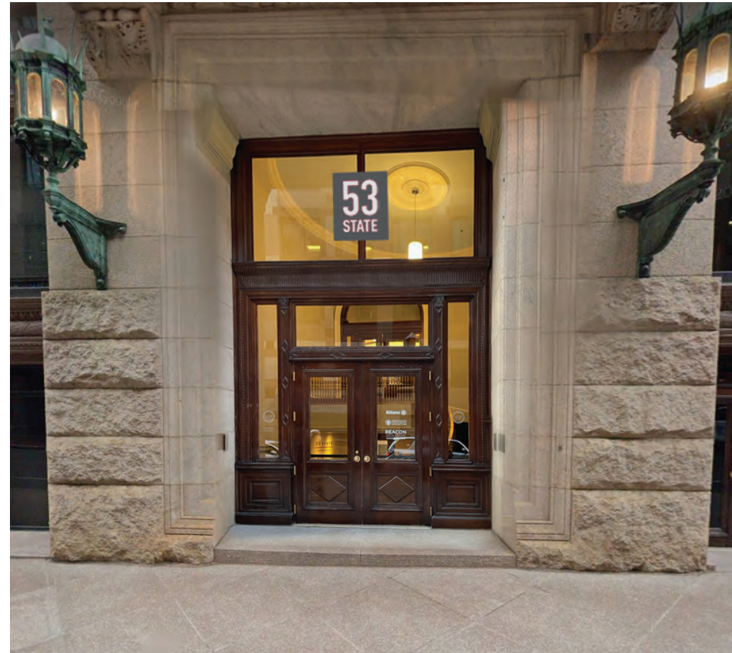
GRAY and WHITE BUILDING ID, dimensional letters on gray powder coated aluminum panel with white dimensional characters, attached with standoffs on glass
