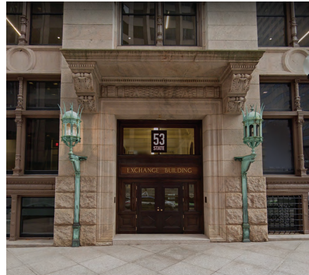
BROWN and GRAY BUILDING ID, dimensional letters on brown powder coated aluminum panel with gray dimensional characters, attached with standoffs on glass
