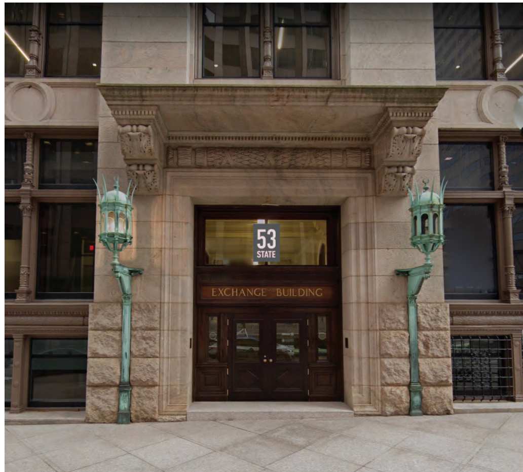
GRAY and WHITE BUILDING ID, dimensional letters on gray powder coated aluminum panel with white dimensional characters, attached with standoffs on glass
