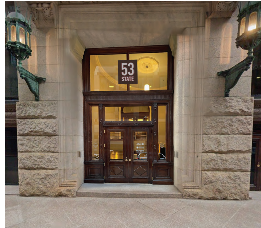
BROWN and GRAY BUILDING ID, dimensional letters on brown powder coated aluminum panel with gray dimensional characters, attached with standoffs on glass
