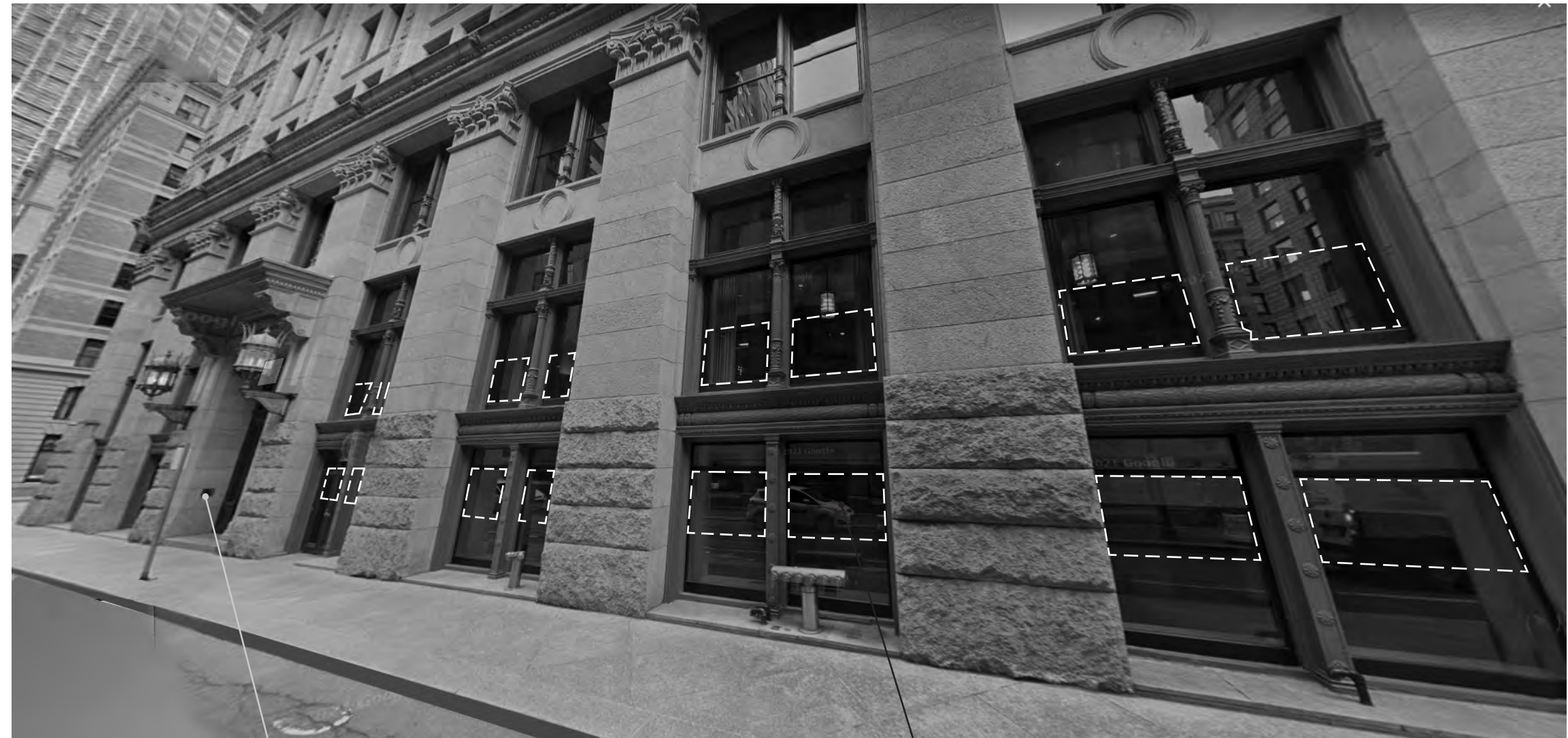
Existing egress signage
