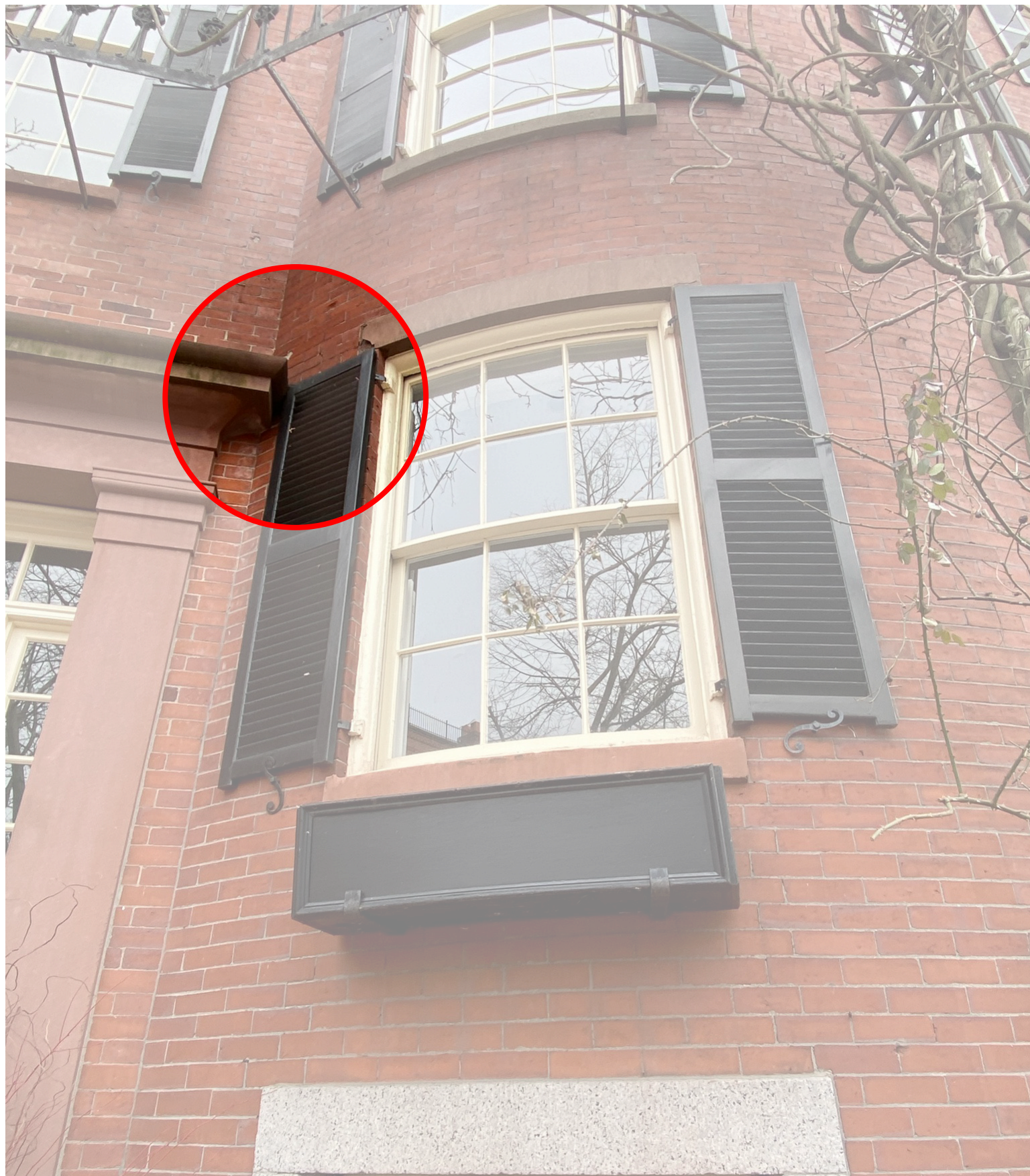
Existing Shutters are less than 1/2 width of masonry opening and cannot be corrected due to position of window
