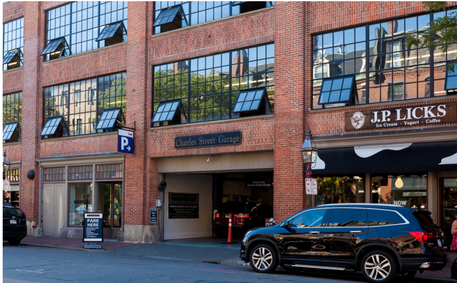
View from Charles Street towards parking entry
