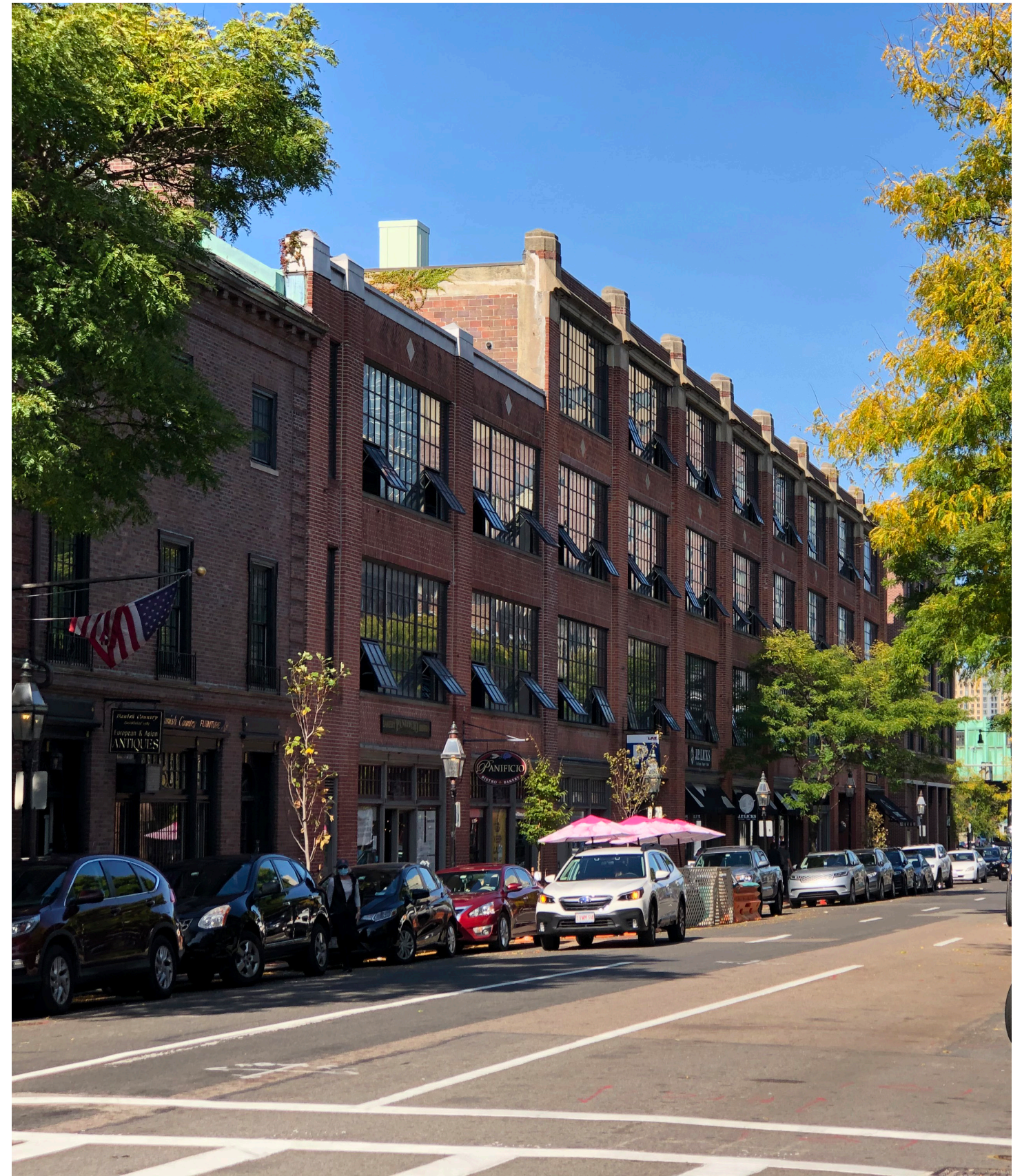
EXISTING VIEW FROM CHARLES STREET
