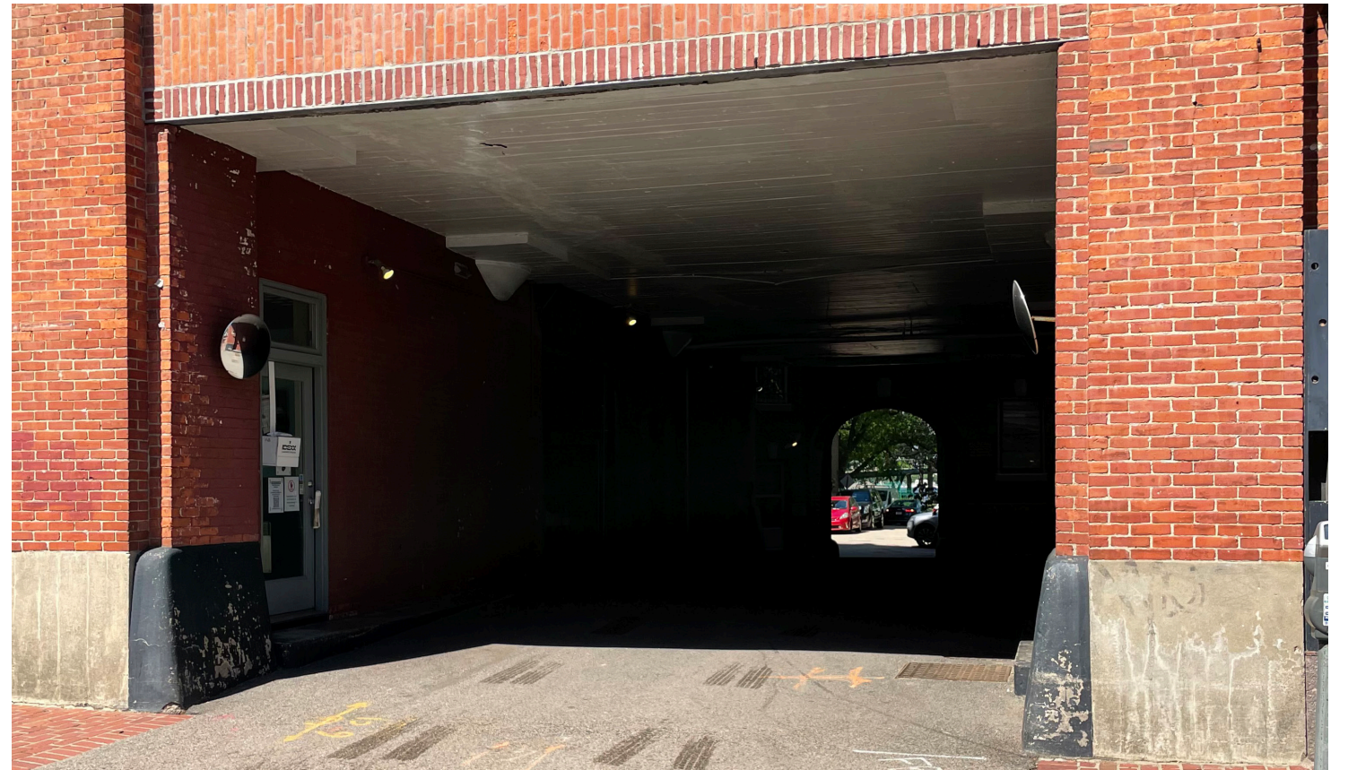
EXISTING VIEW LOOKING WEST
