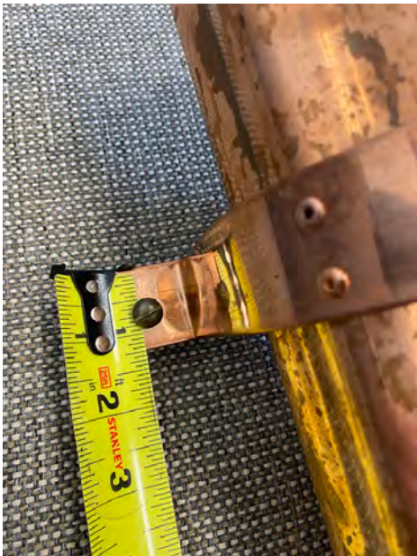
1.25" WIDE COPPER STRAP RIVETED SECURELY TO DOWNSPOUT
