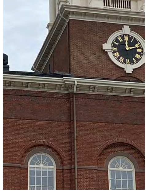
DETAIL OF FACADE WITH PAINTED DOWNSPOUTS
