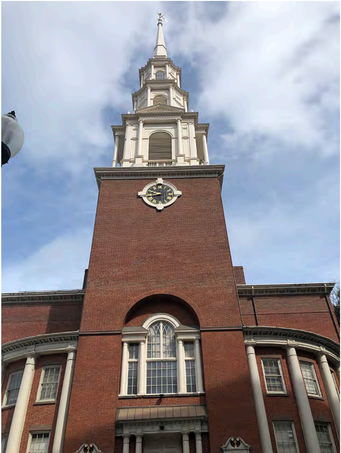
PARK STREET CHURCH TREMONT STREET VIEW OF TOWER & STEEPLE
