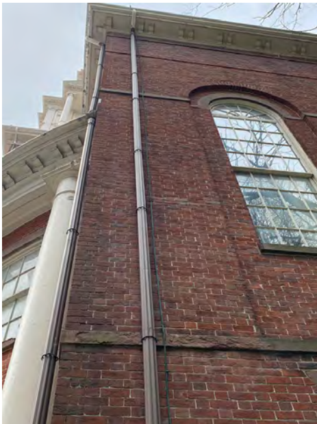
GRANARY BURYING GROUND FACADE DOWNSPOUT WITH INTERMITTENT BRACKETS
