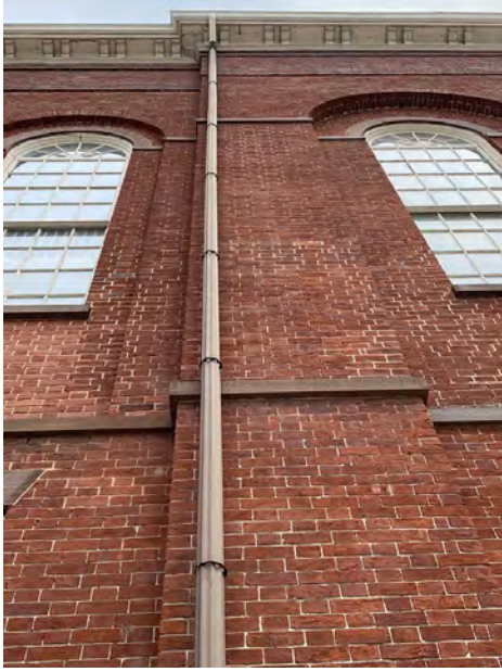
PARK STREET FACADE DOWNSPOUT WITH INTERMITTENT BRACKETS
