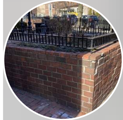
EXISTING BRICK RAISED PERIMETER PLANTERS
