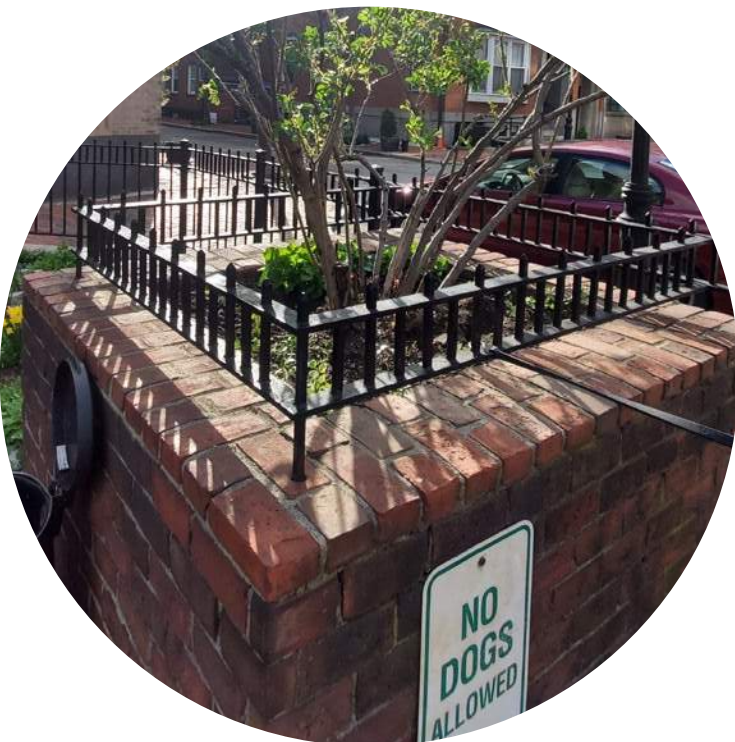
Raised planter at Melrose Street entrance
