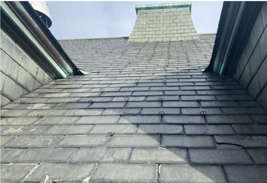
(E) Snow Guards on Main Roof
