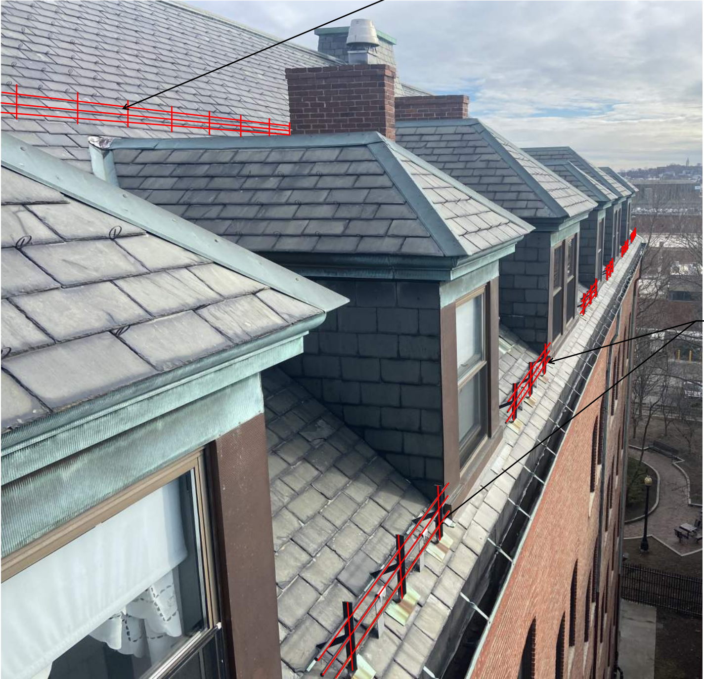
Proposed Snow Fence Layout
