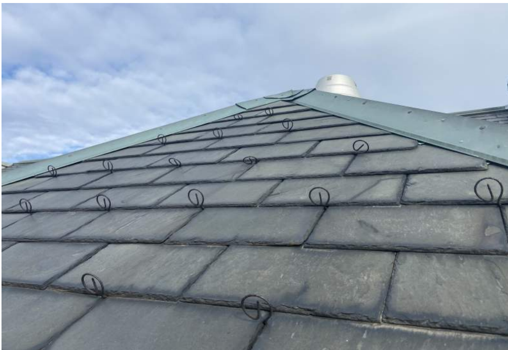
(E) Snow Guards on Dormer Roof
