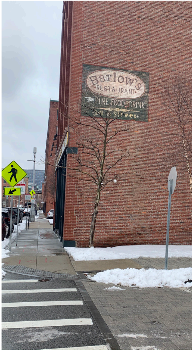
Minor Work During Renovation
