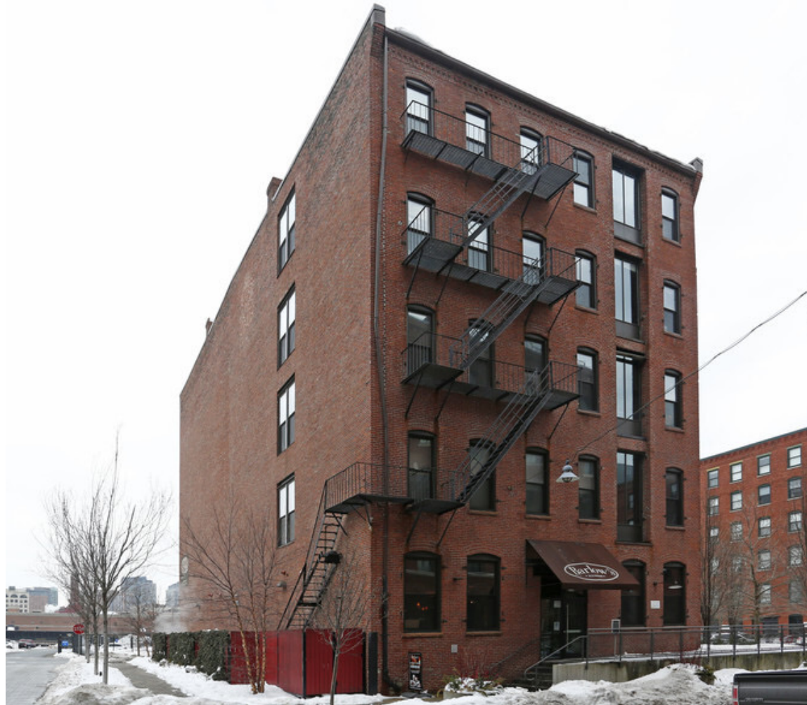
Fire Escape View From Channel Center Street
