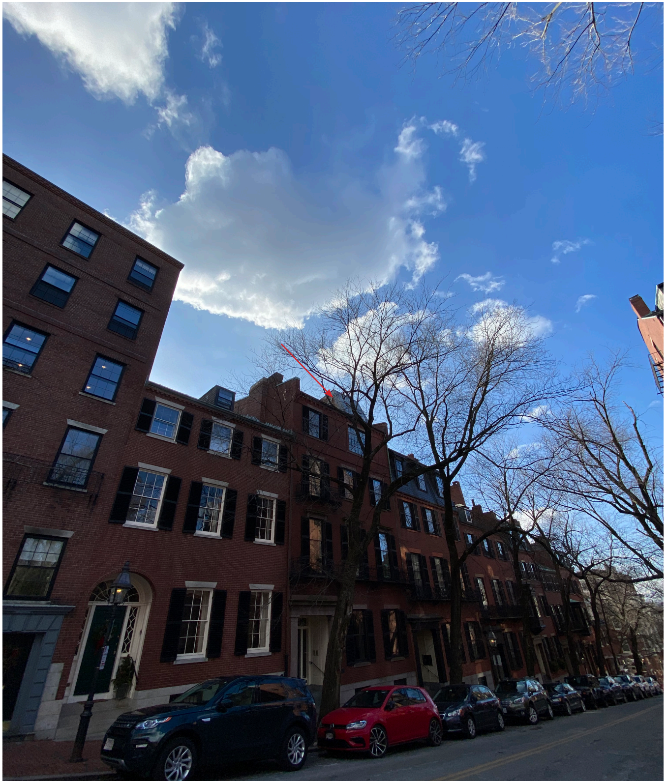
5. LEFT SIDE OF DORMER CLADDING
