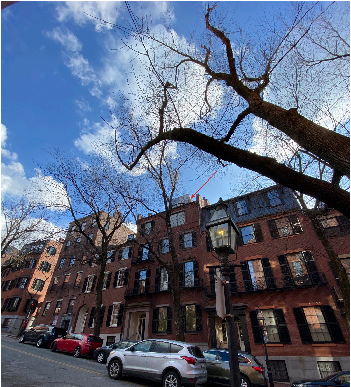
3. RIGHT SIDE OF DORMER CLADDING
