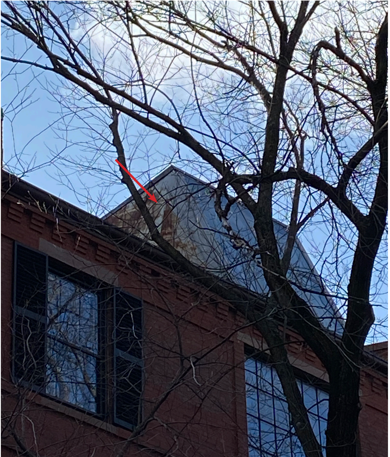
⑥ LEFT SIDE OF DORMER CLADDING
