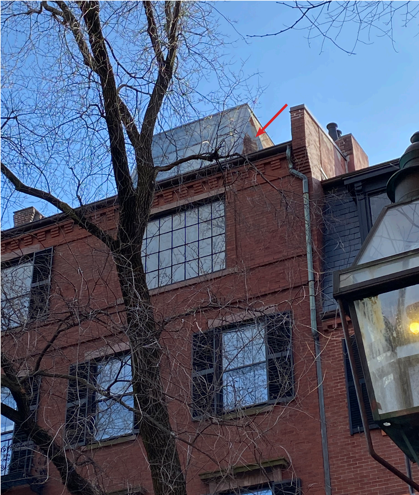
4. RIGHT SIDE OF DORMER CLADDING
