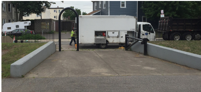
Ramp on Harbor View Street
