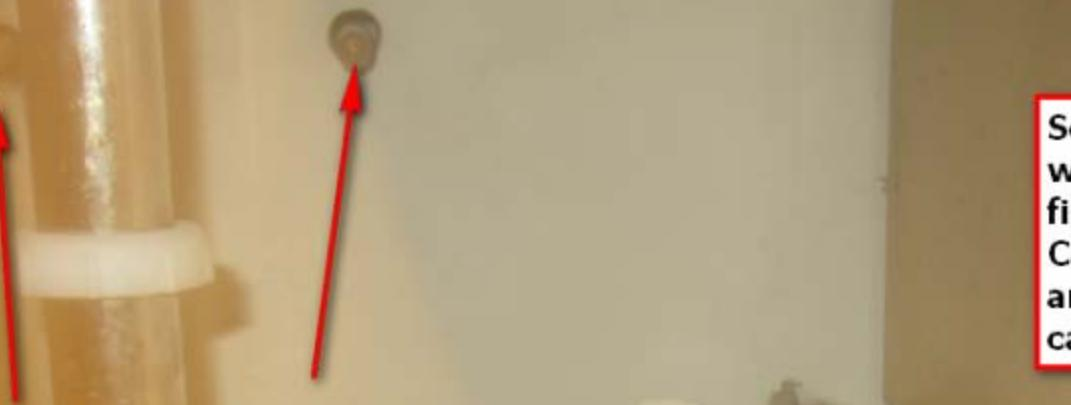
**Problem:** this kitchen cabinet replacement project includes running new pipe penetrations through existing walls. This will give mice and roaches access to the void behind the new cabinets.
