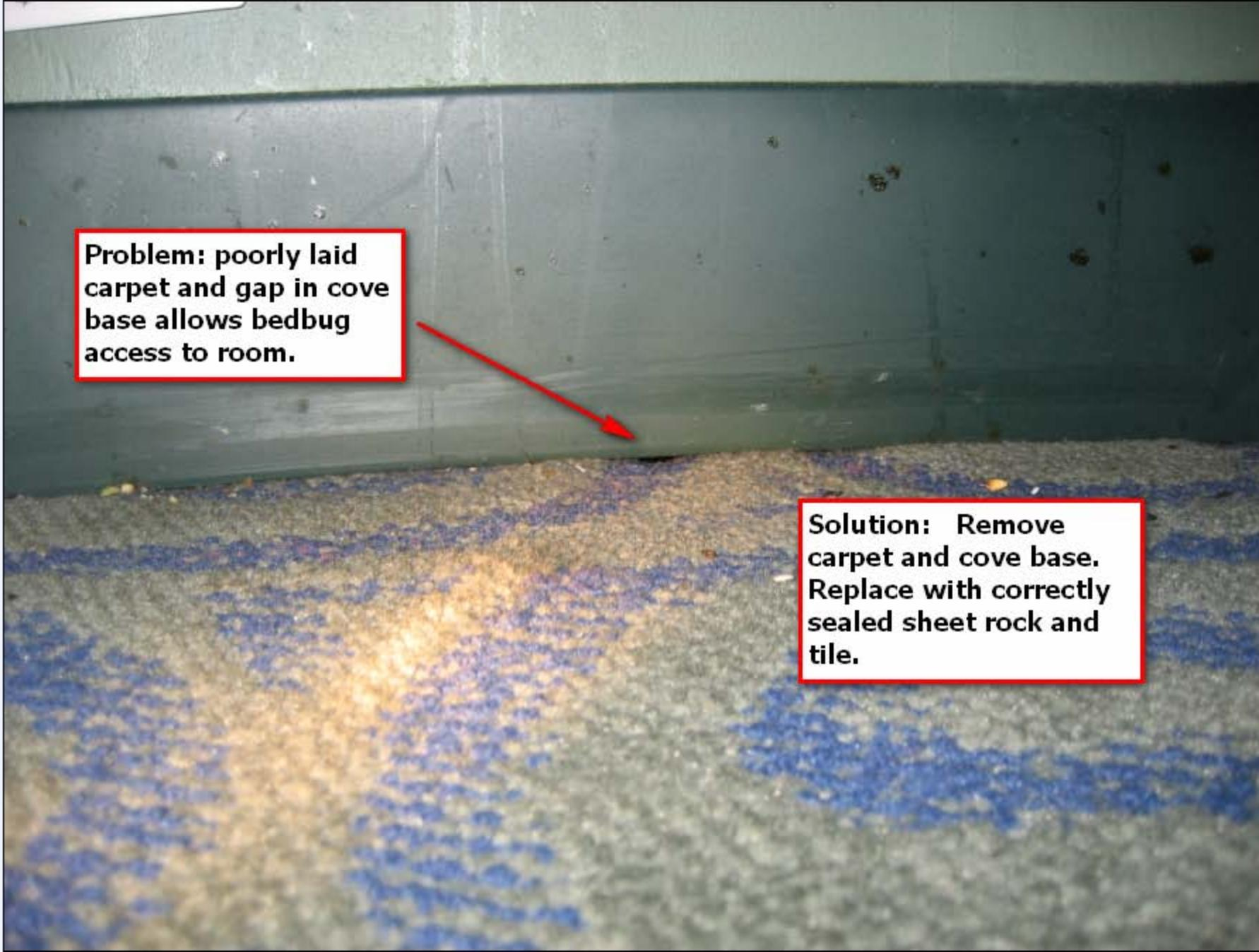
**Problem:** poorly laid carpet and gap in cove base allows bedbug access to room.
