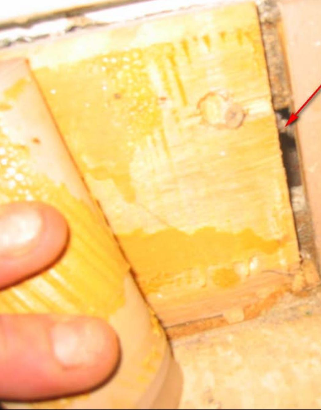
**Problem:** gap in wood backing gives pests access to wall cavity and other rooms.
