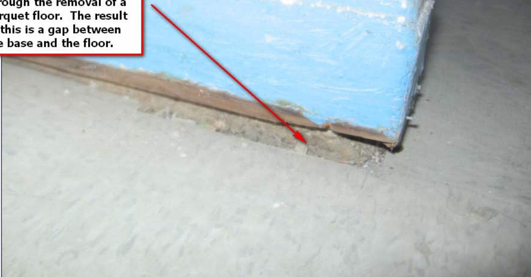
**Problem:** the installation of the new strip creates access and harborage for insects and if large enough, for mice.
