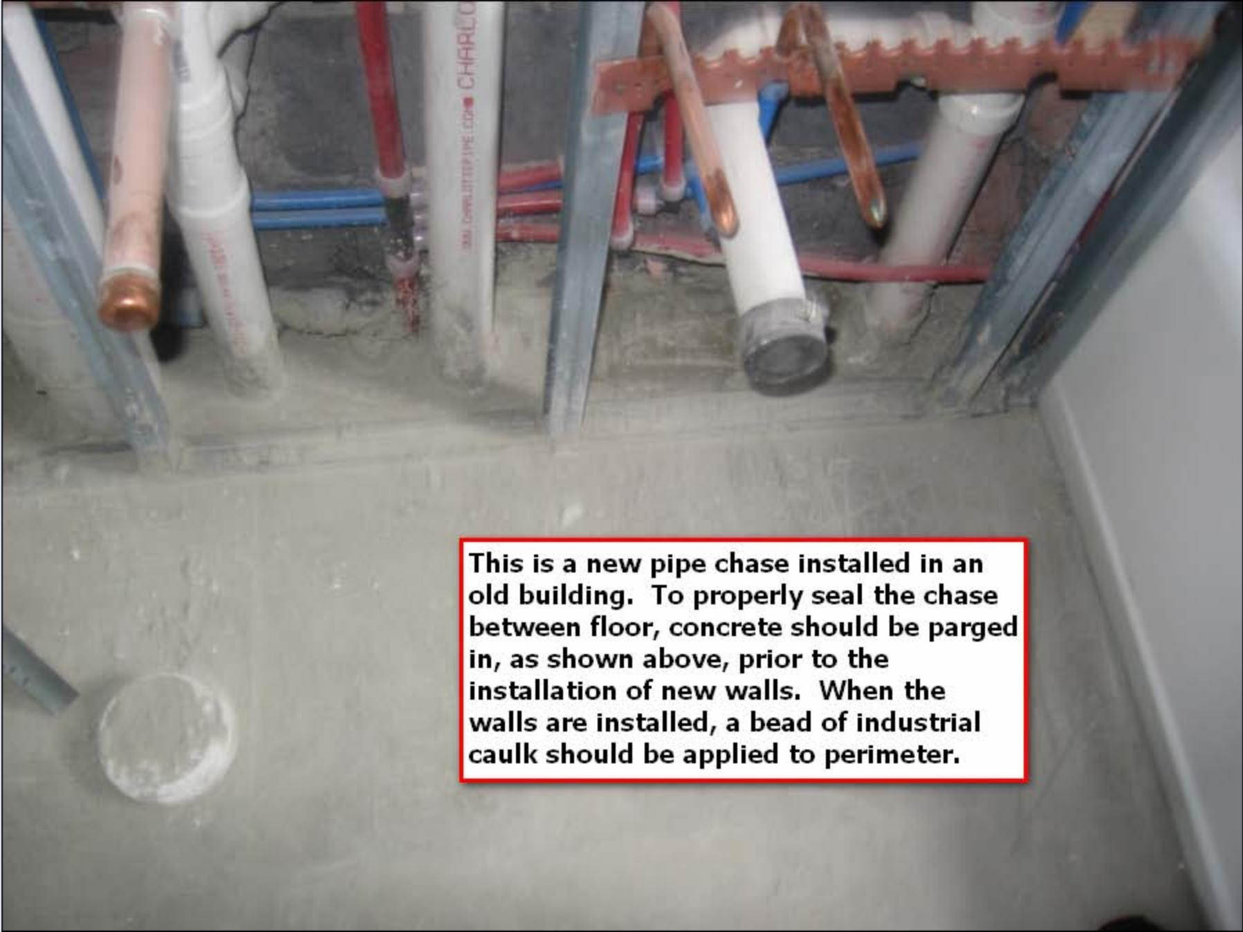
This is a new pipe chase installed in an old building. To properly seal the chase between floor, concrete should be parged in, as shown above, prior to the installation of new walls. When the walls are installed, a bead of industrial caulk should be applied to perimeter.
