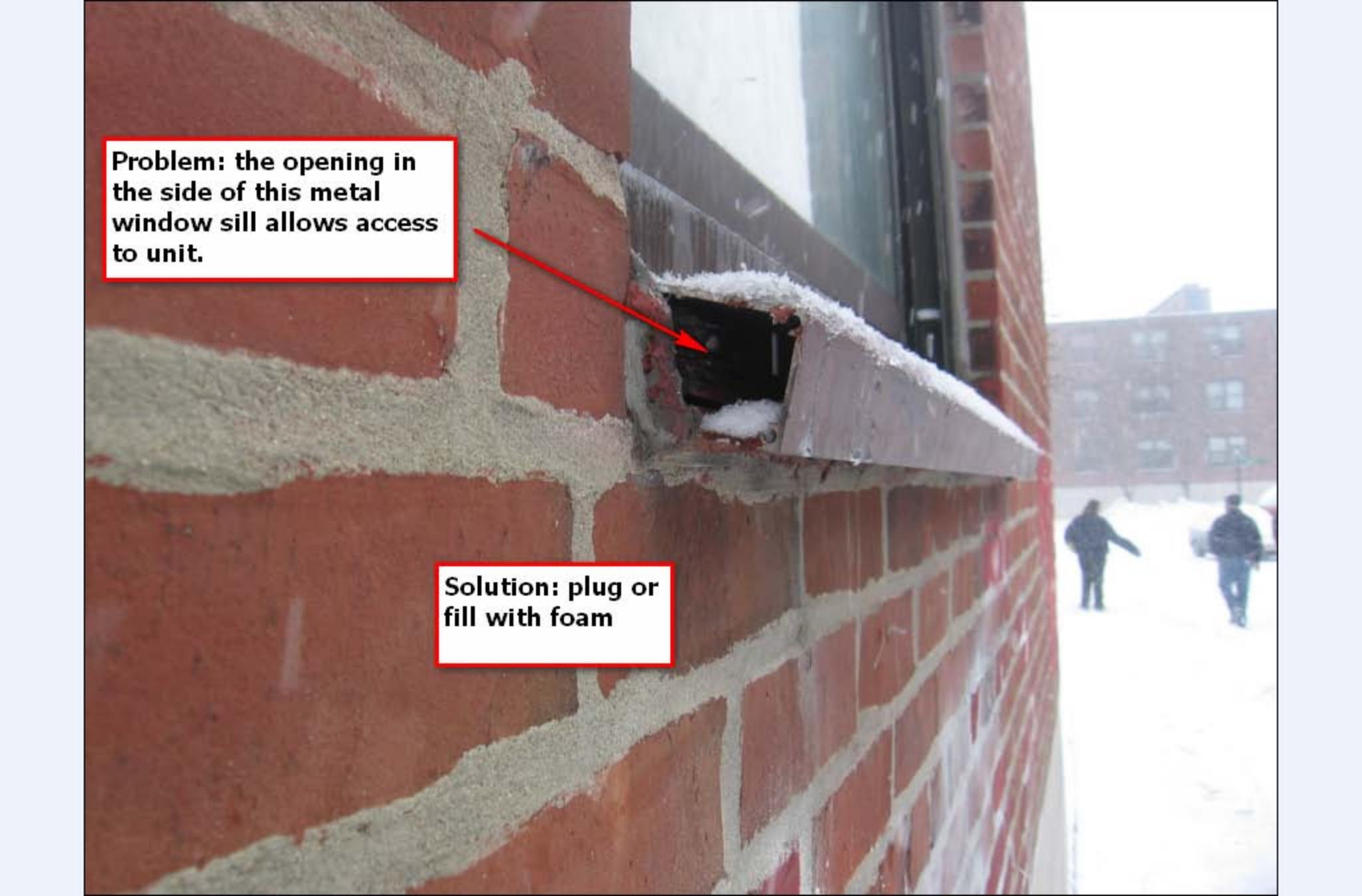
**Problem:** the opening in the side of this metal window sill allows access to unit.
