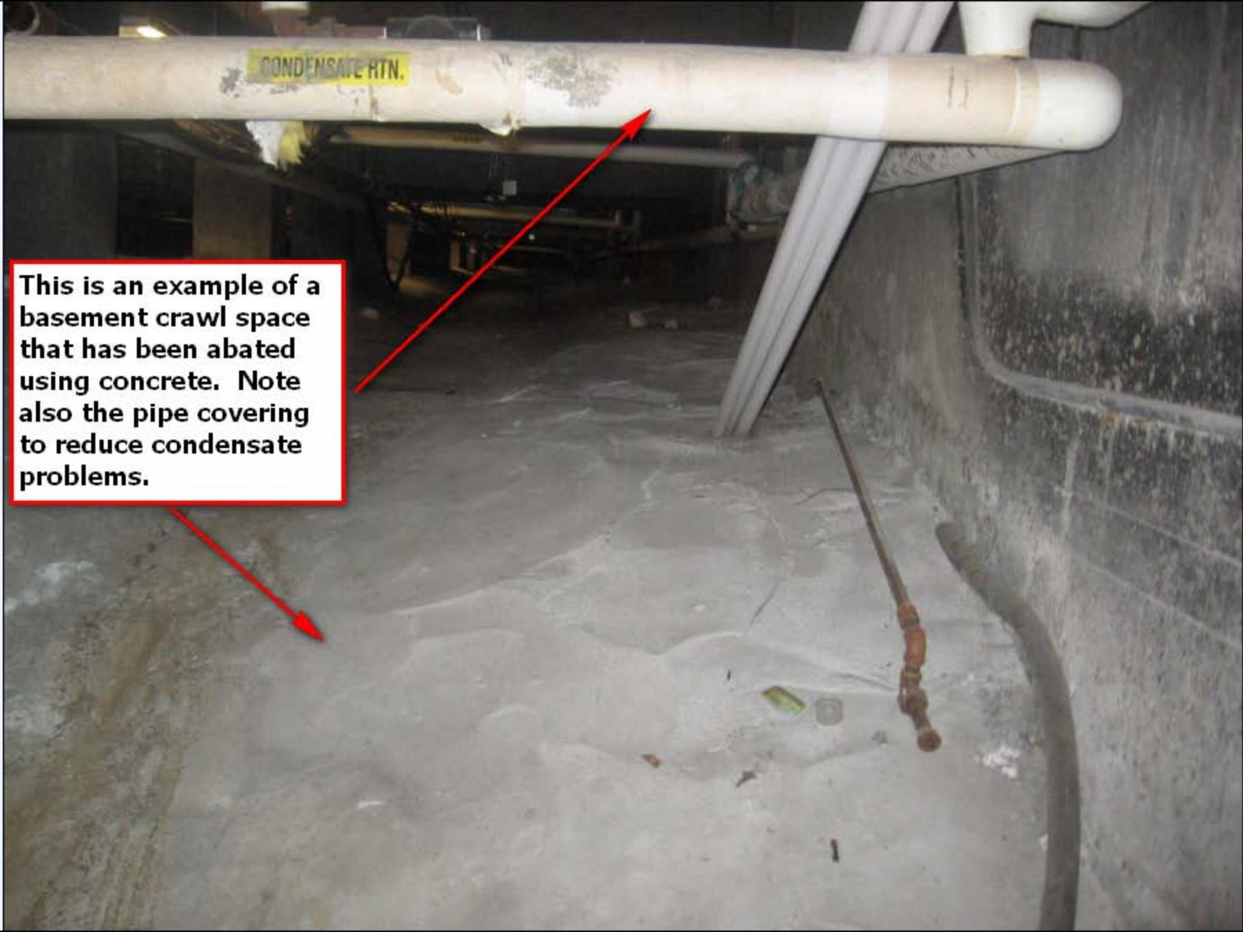
This is an example of a basement crawl space that has been abated using concrete. Note also the pipe covering to reduce condensate problems.
