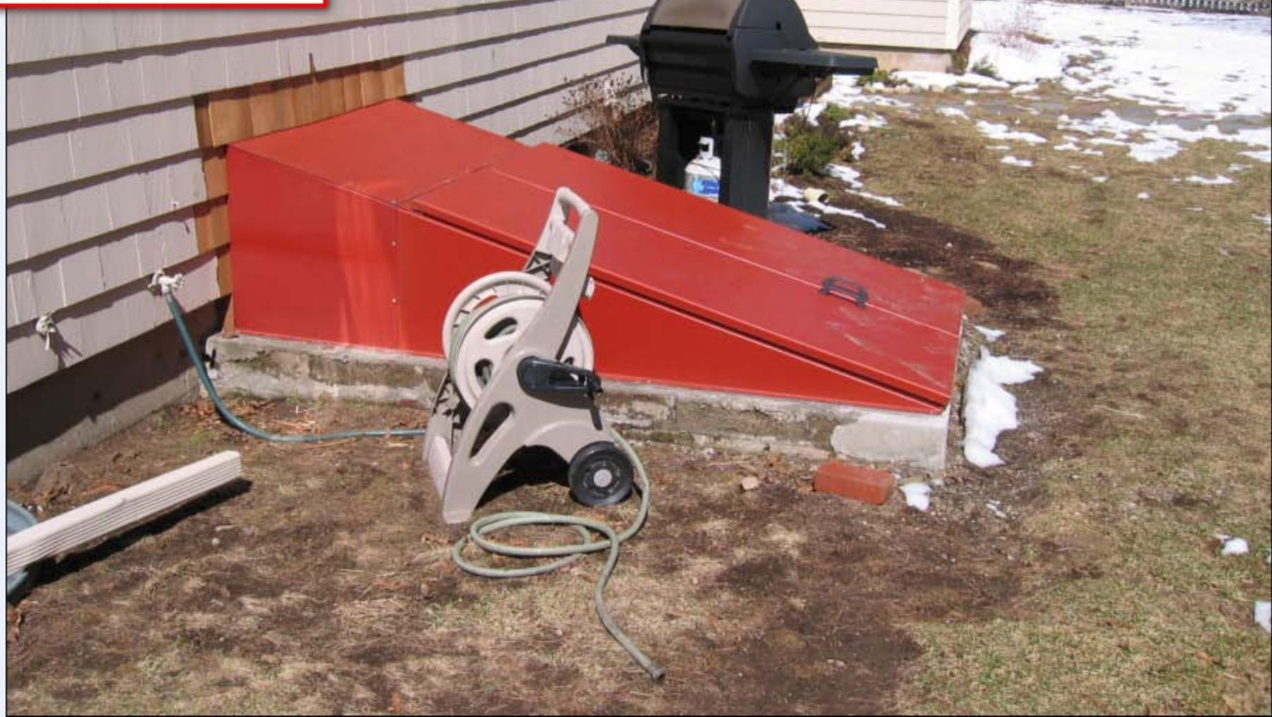
**Problem:** Daylight indicates gaps in bulkhead doors and frame. Easy access for pests.
