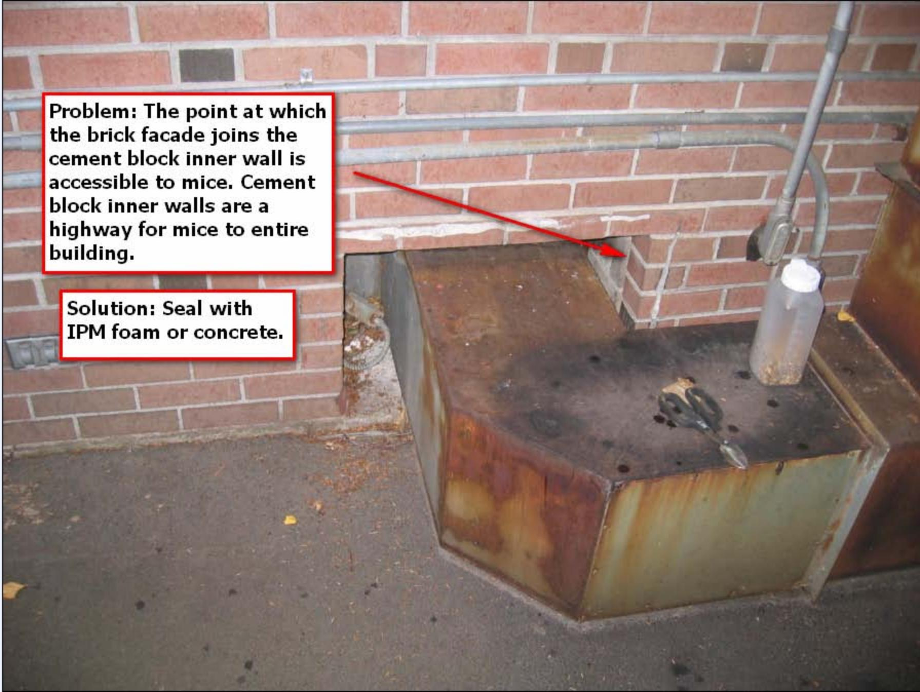
**Problem:** Open exterior wall penetration for utility lines creates easy access for pests.
