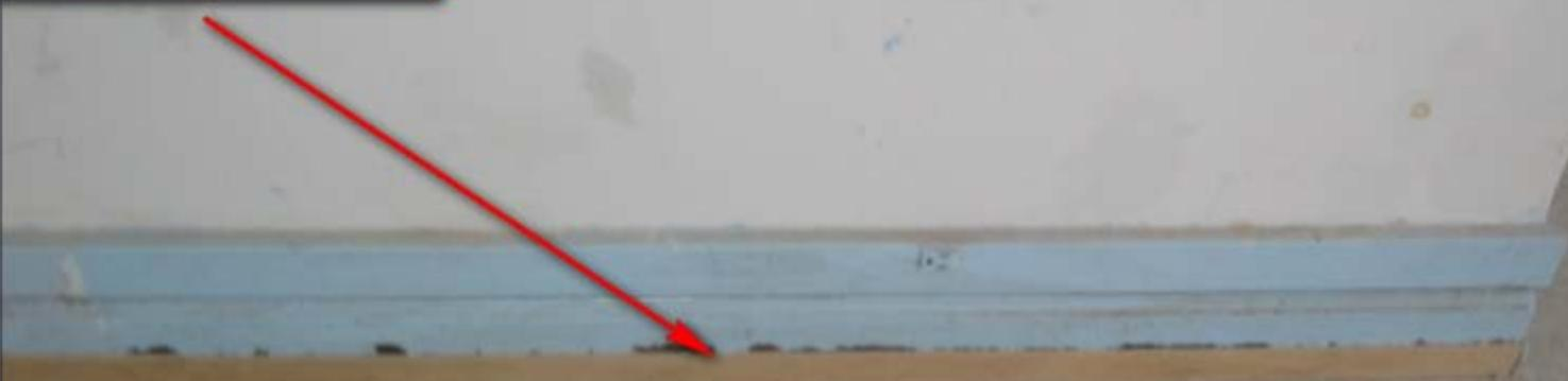
However, another view shows that the level of the floor has been dropped through the removal of a parquet floor. The result of this is a gap between the base and the floor.
