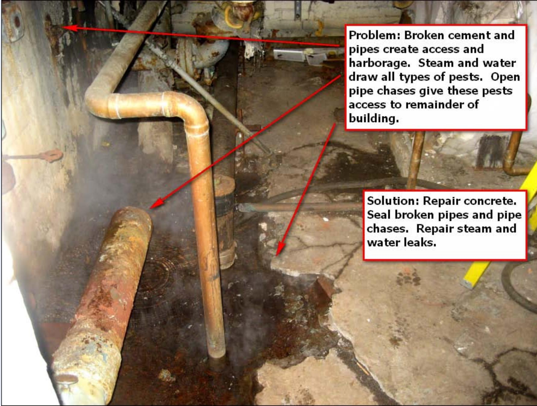
**Problem:** Broken cement and pipes create access and harborage. Steam and water draw all types of pests. Open pipe chases give these pests access to remainder of building.
