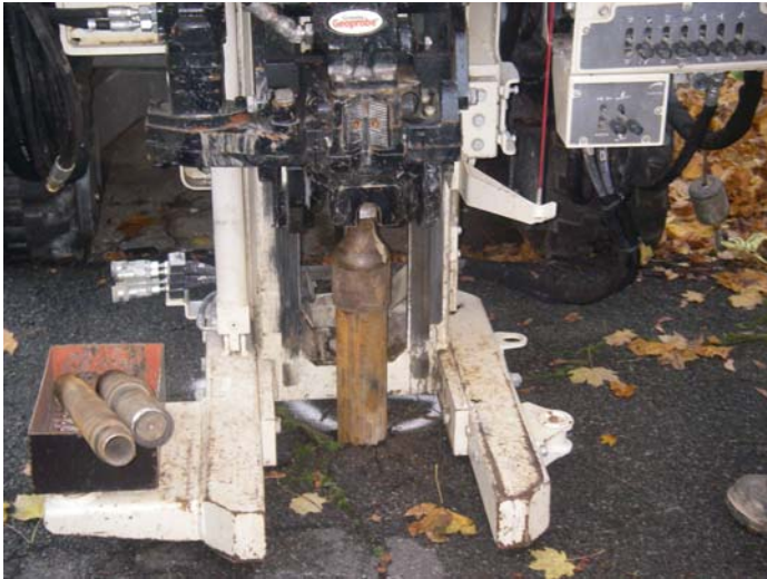
Photo 1: Rubber track percussion drill rig
