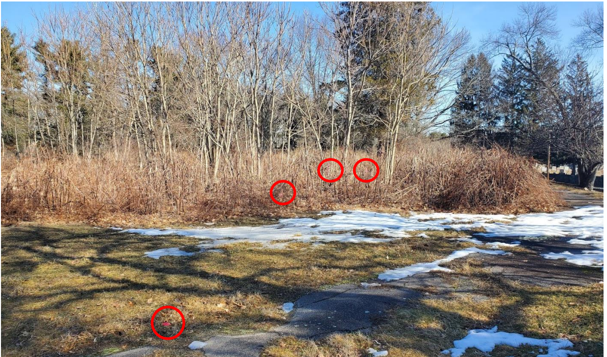
Photo #2: View of the project area and the stands of Japanese knotweed and tree of heaven obscuring and damaging the historic foundation. Pink flags denote the limits of the 100-foot buffer zone. The wetland resources are located to the right of this photo. Facing east.
