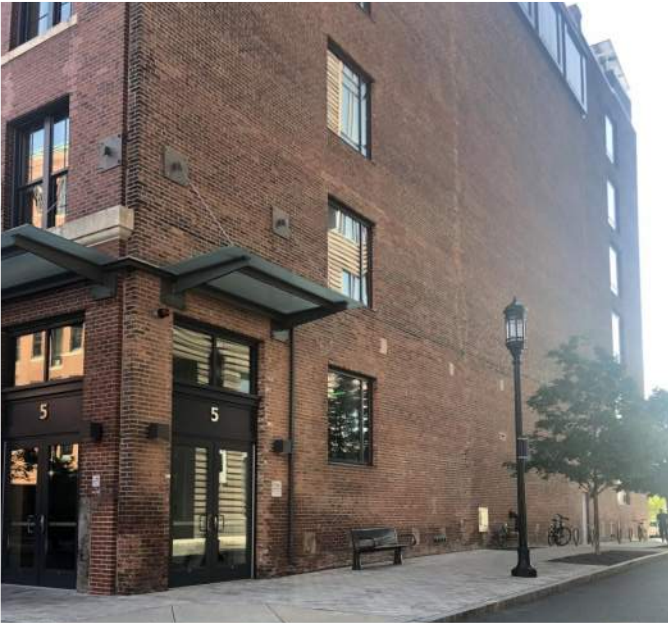
VIEW OF IRON STREET FACADE FROM CHANNEL ST
