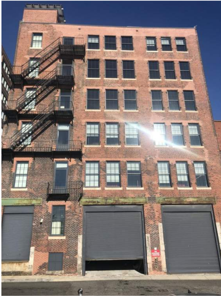
VIEW OF FRONT FACADE
