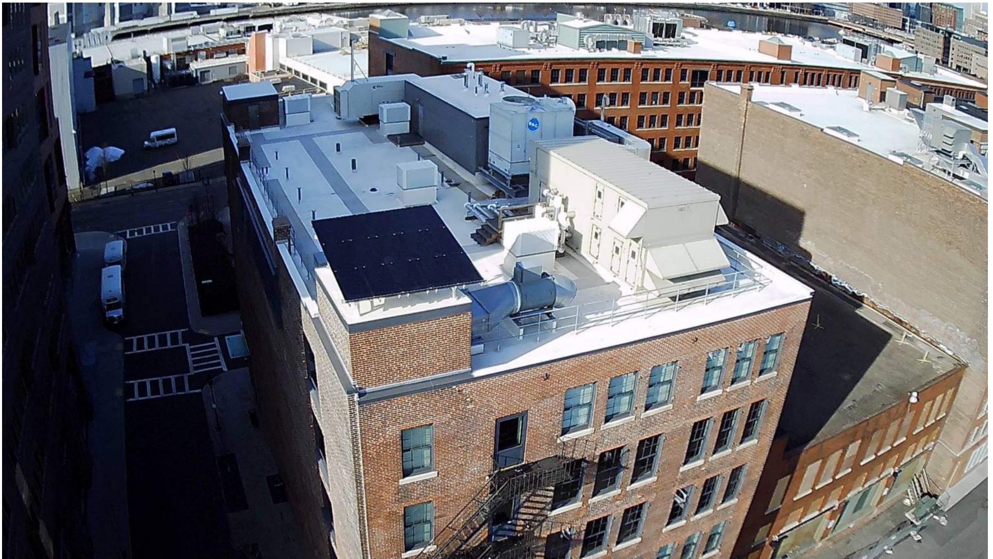
AERIAL VIEW OF EXISTING ROOFTOP EQUIPMENT
